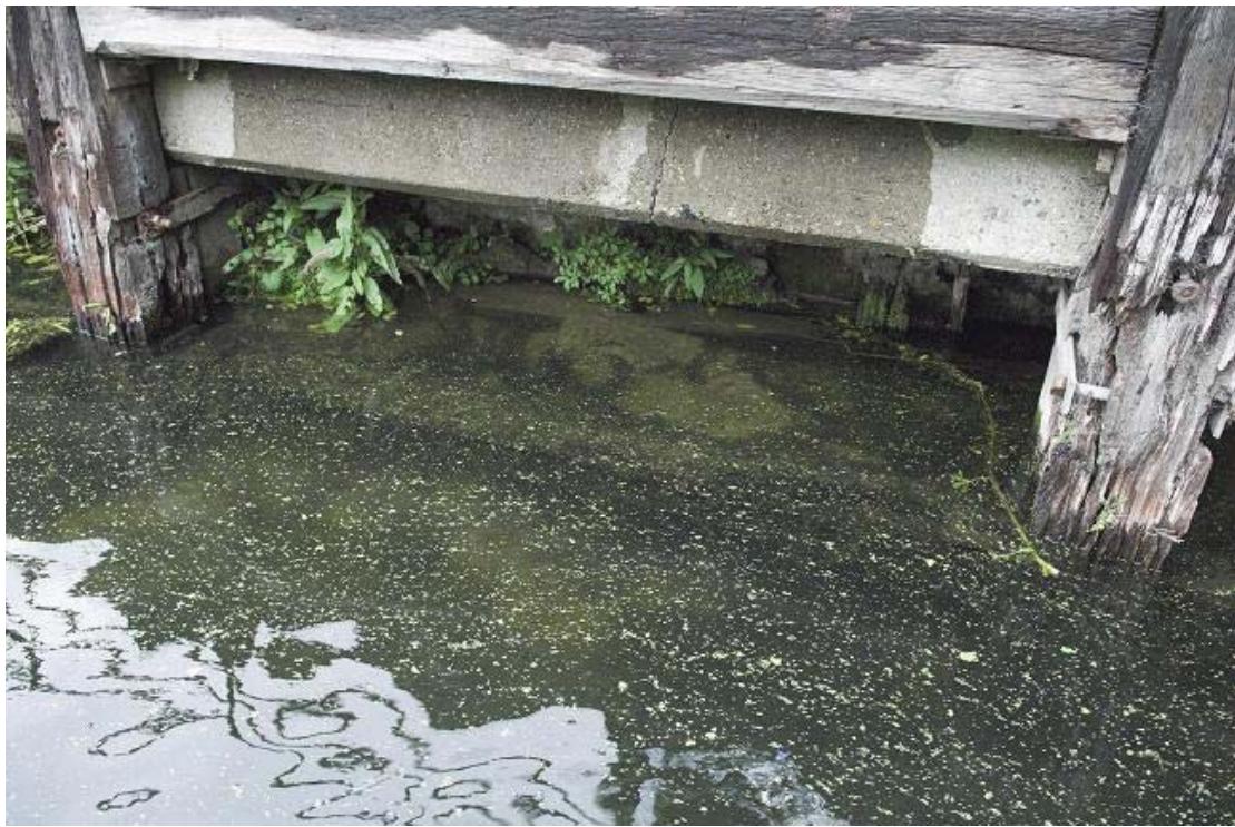
Plate 28 View of eastern concrete bank of City Mill River with timber pull-up piles, looking south-east: OL-01207
