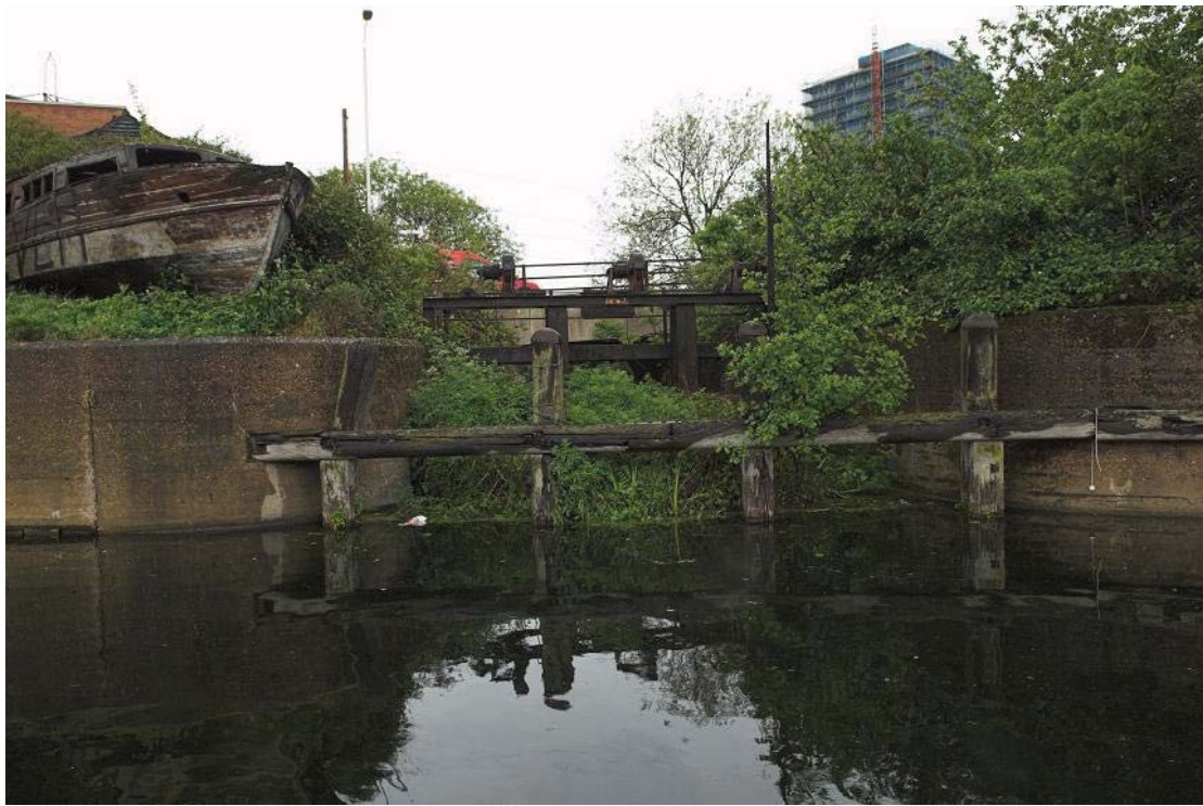
Plate 30 View of disused portion of Marshgate Lane Lock, City Mill River, looking east: OL-07407
