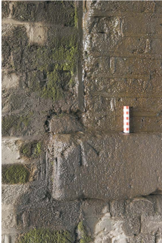
Plate 43 Detail of a benchmark carved into the impost band of the primary phase of construction of the GER bridge across Pudding Mill Lane, looking south-west
