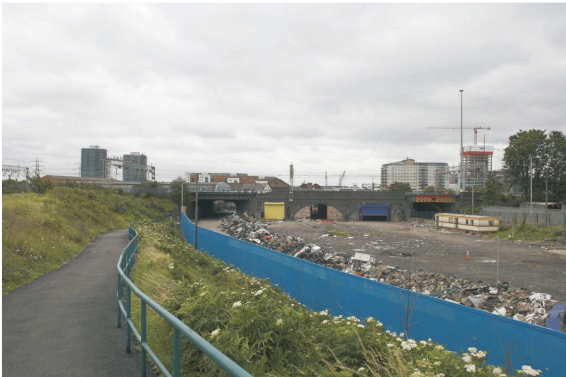
Plate 8 Part of the GER Stratford viaduct, between Pudding Mill Lane and Marshgate Lane, seen from the Greenway, looking south
