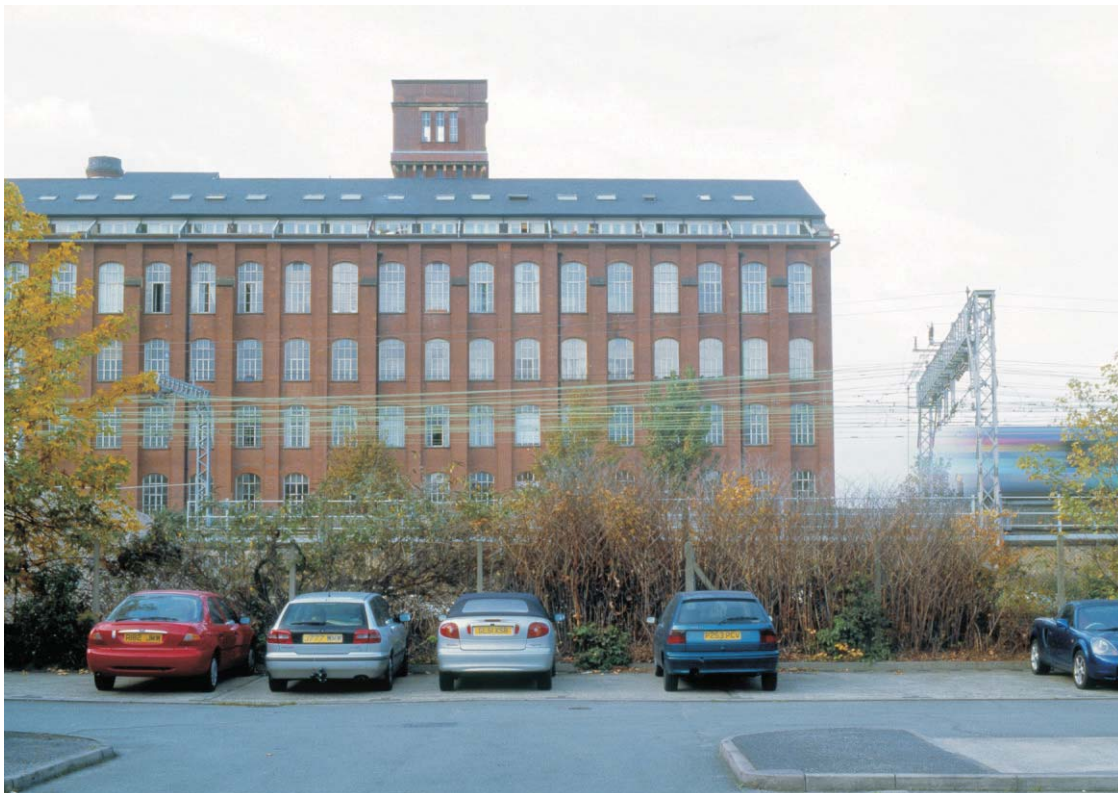
Plate 2 The low brick viaduct carrying the GER past the former Bryant and May match factory, looking north
