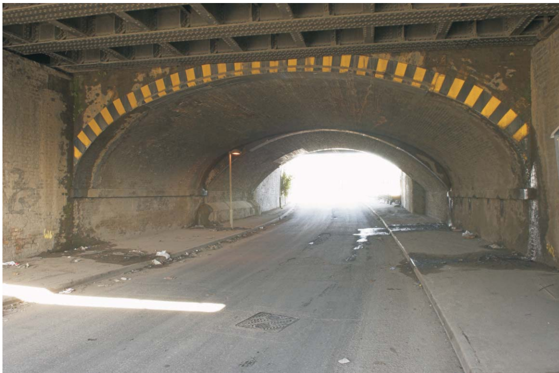
Plate 36 The elliptical Braithwaite arch of the primary phase of construction of the GER bridge over Pudding Mill Lane, looking north-west
