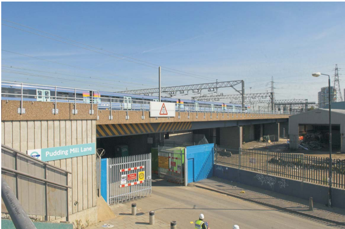
Plate 32 The southern side of the GER Stratford viaduct, looking north-east
