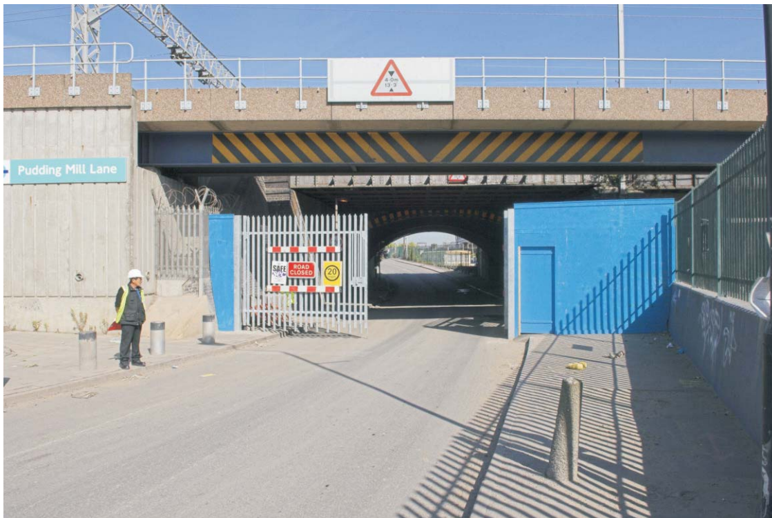
Plate 35 The southern side of the GER bridge across Pudding Mill Lane, looking north-west
