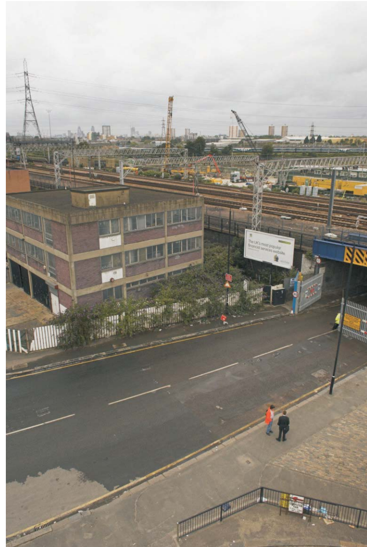
Plate 12 The GER embankment, from Carpenter's Road, looking north-west
