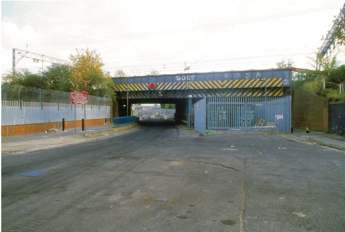
Plate 3 The GER bridge over Wick Lane, looking south
