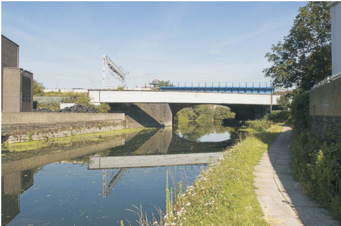
Plate 6 The GER embankment and bridge over the River Lea, looking north-west
