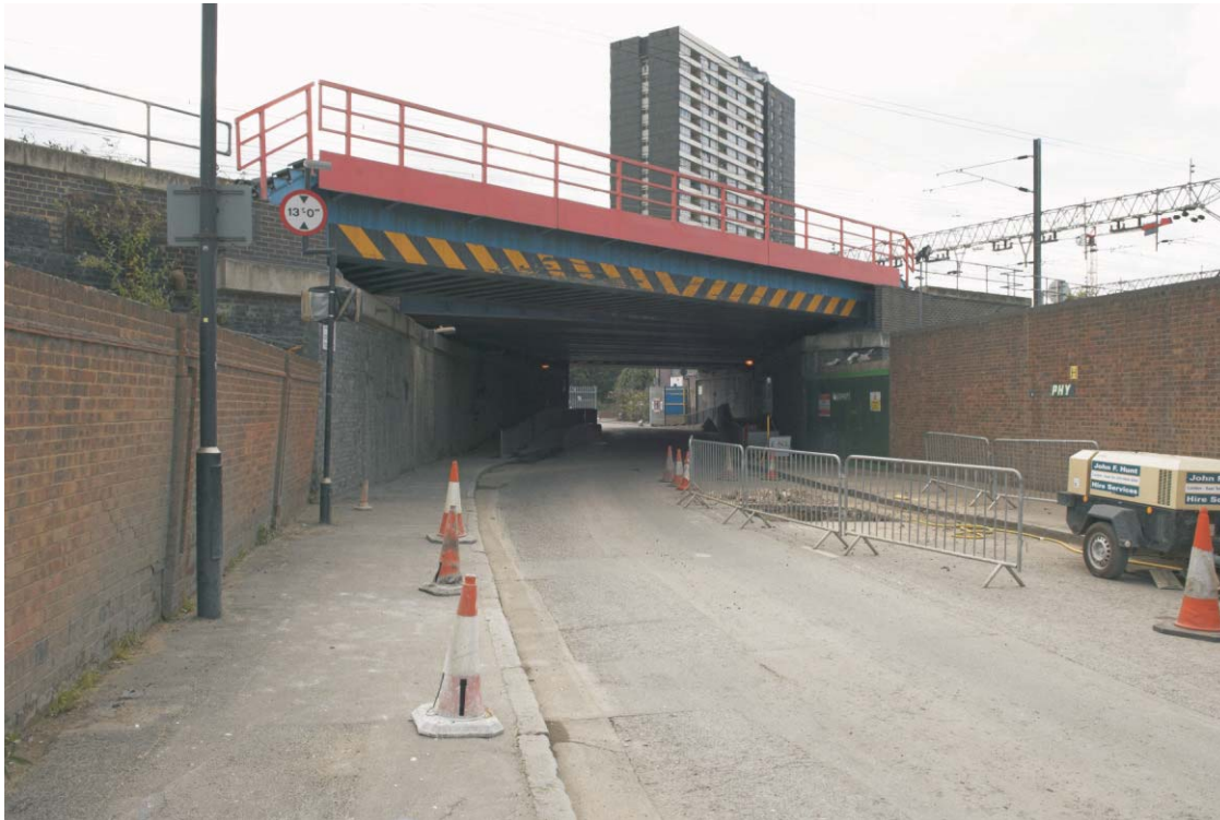
Plate 13 The GER bridge over Carpenter's Road, looking south-east
