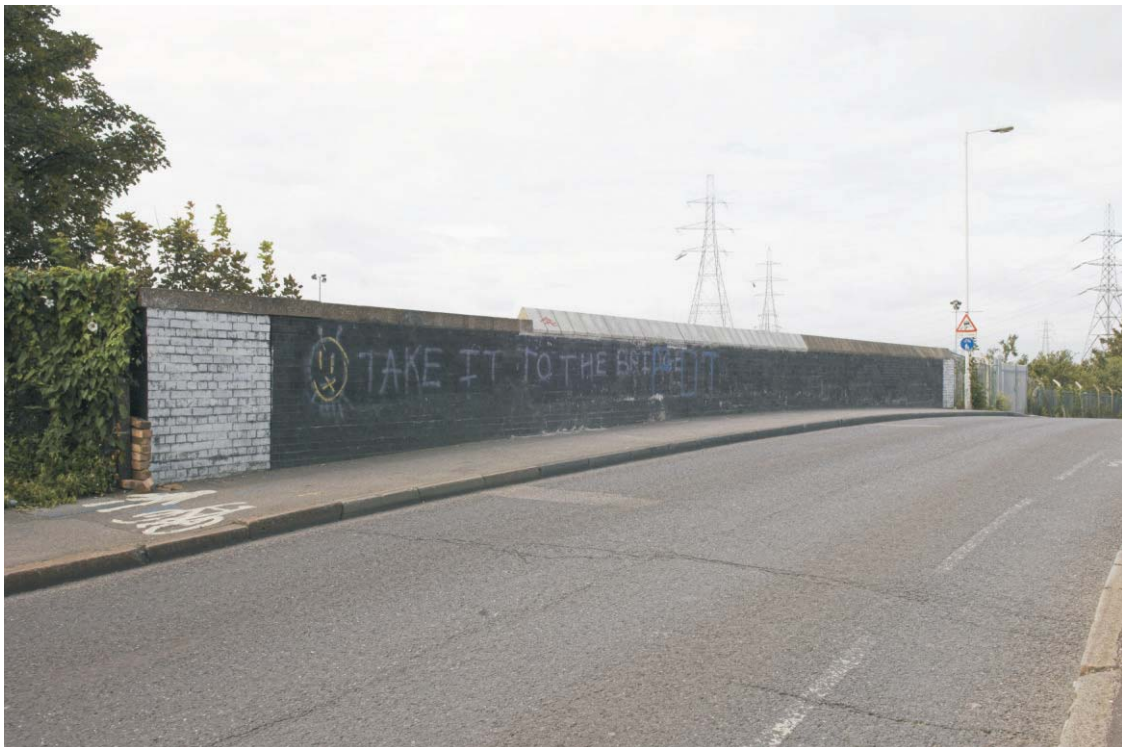
Plate 20 Temple Mill Lane bridge, looking south-west
