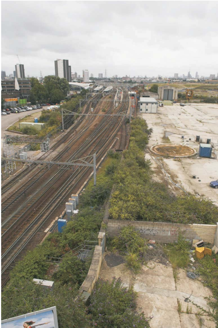
Plate 15 The GER line to Stratford Station, looking west from Angel Lane
