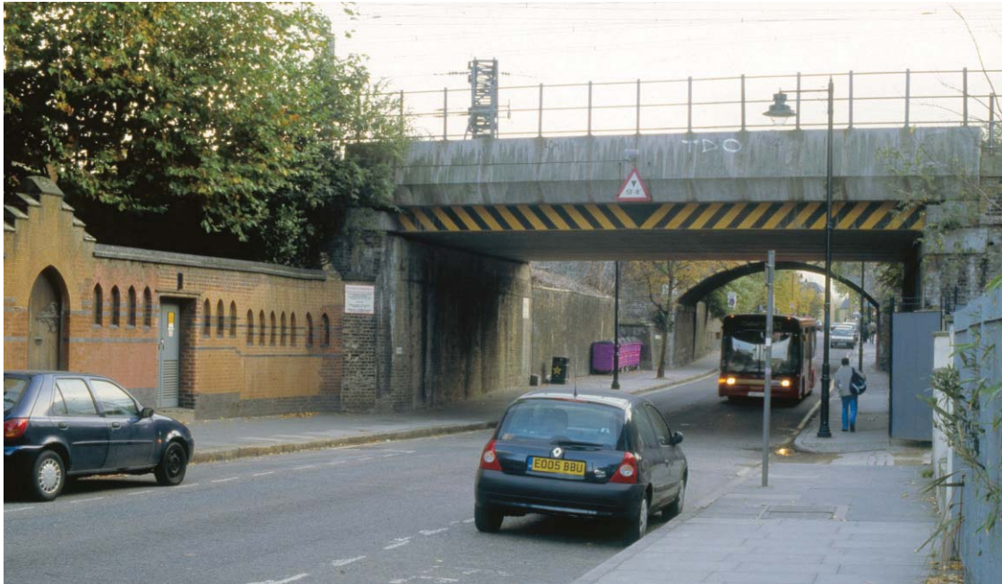
Plate 1 The GER bridge over Fairfield Road in Bow, looking south
