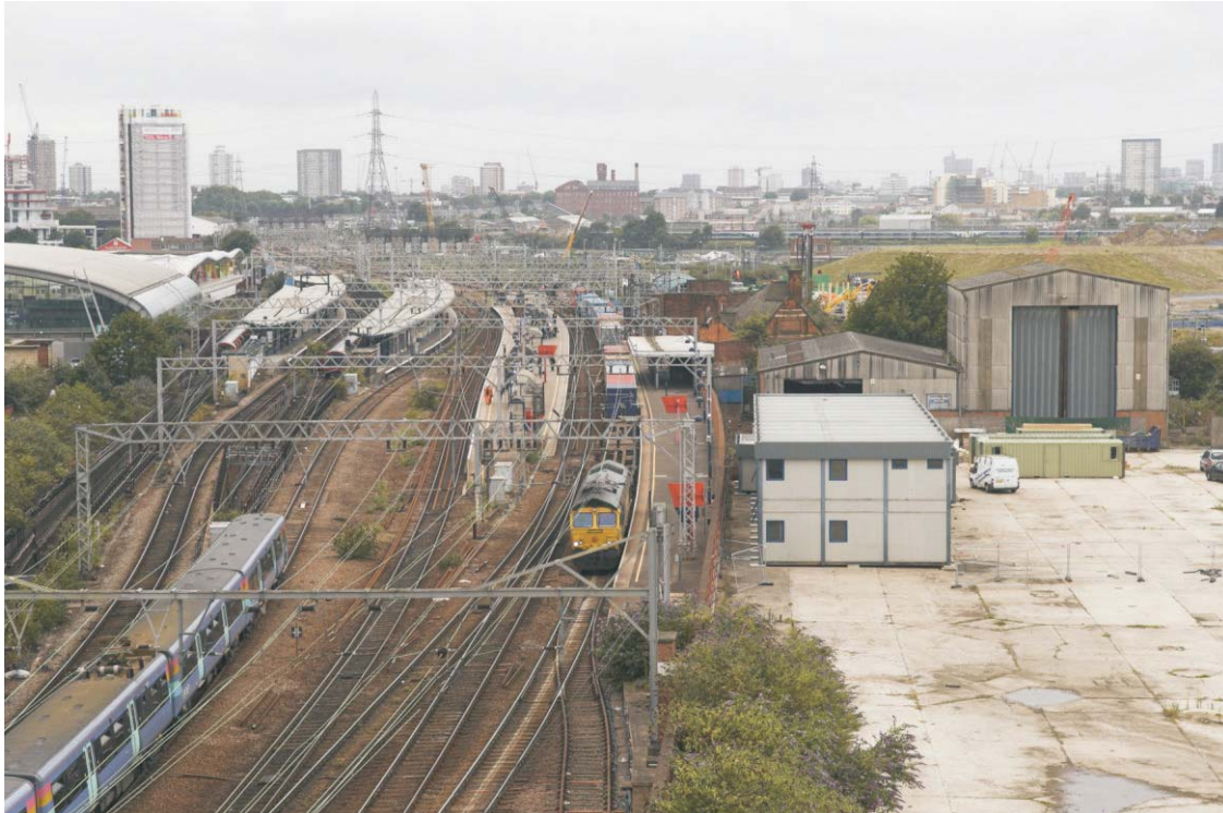
Plate 17 Stratford Station, looking west
