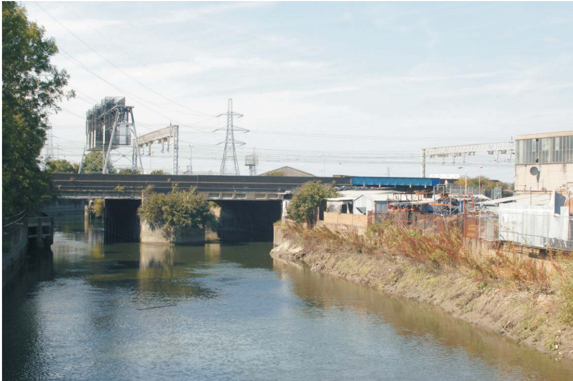
Plate 9 The GER bridge over the Waterworks River, looking north
