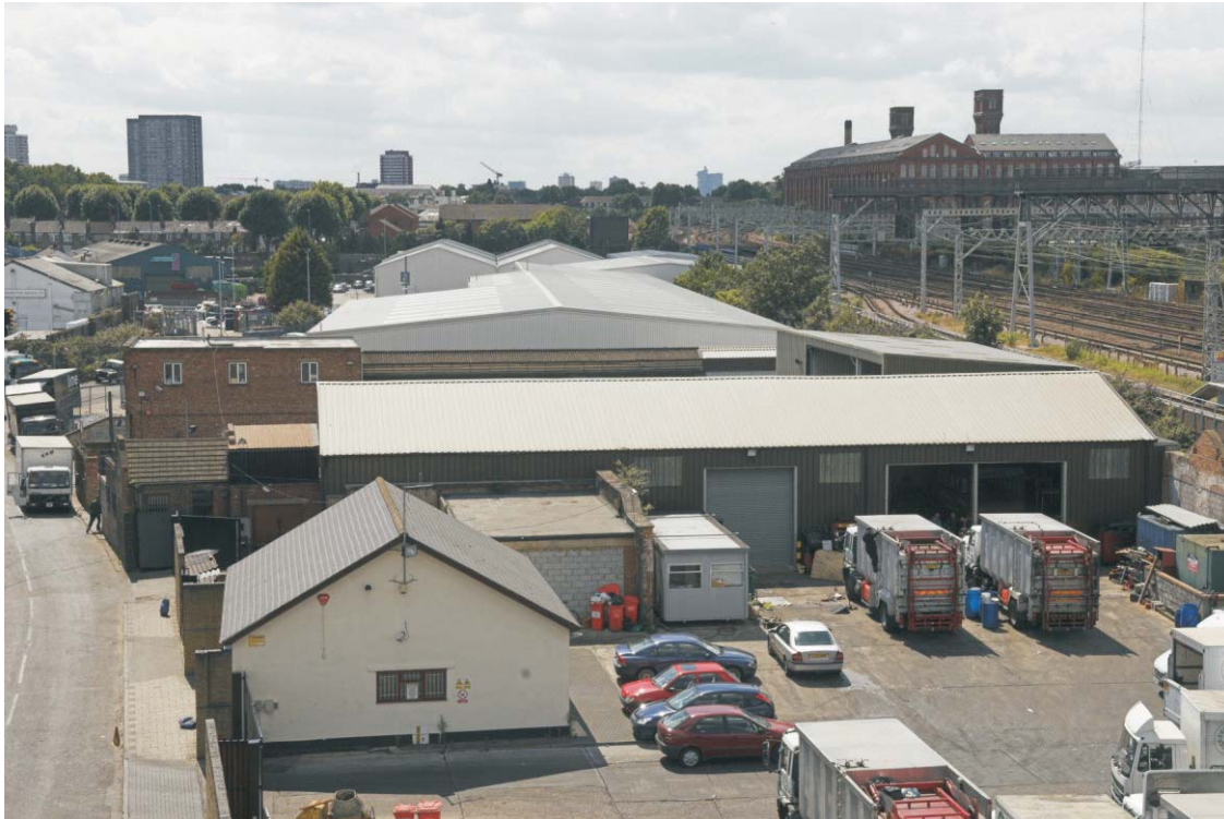
Plate 7 The GER embankment between the River Lea and Pudding Mill Lane
