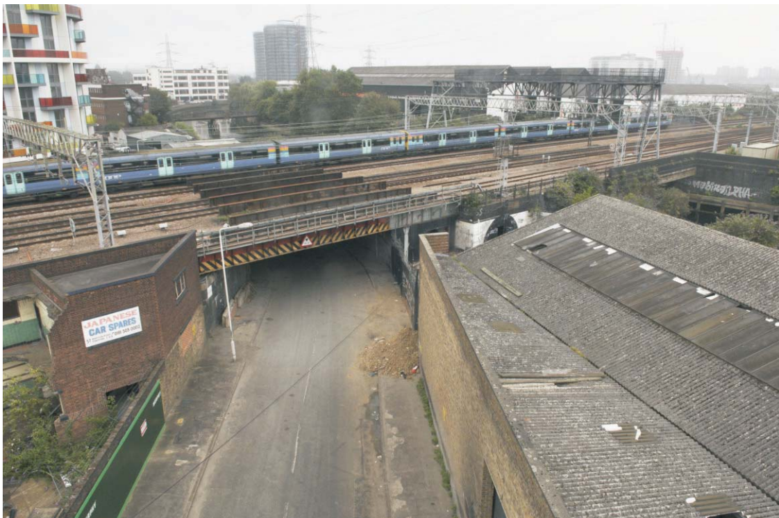
Plate 10 The GER bridge over Warton Road, looking south-east
