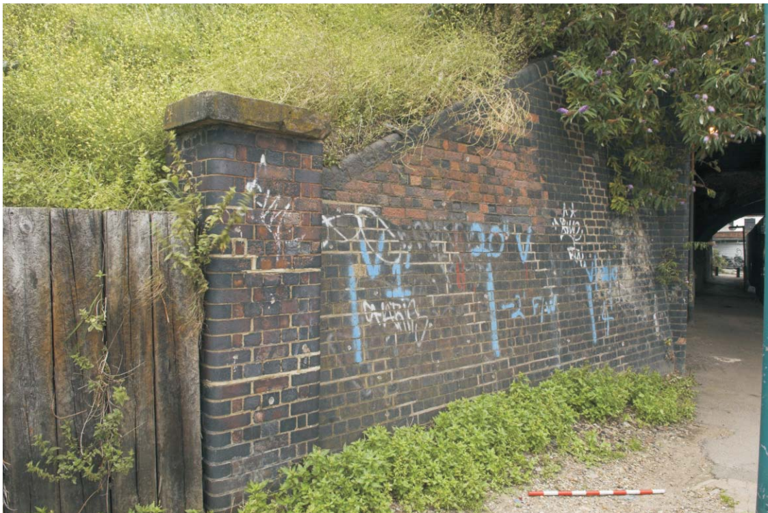
Plate 56 The brick retaining wall of the embankment to the east of Marshgate Lane, looking south-east
