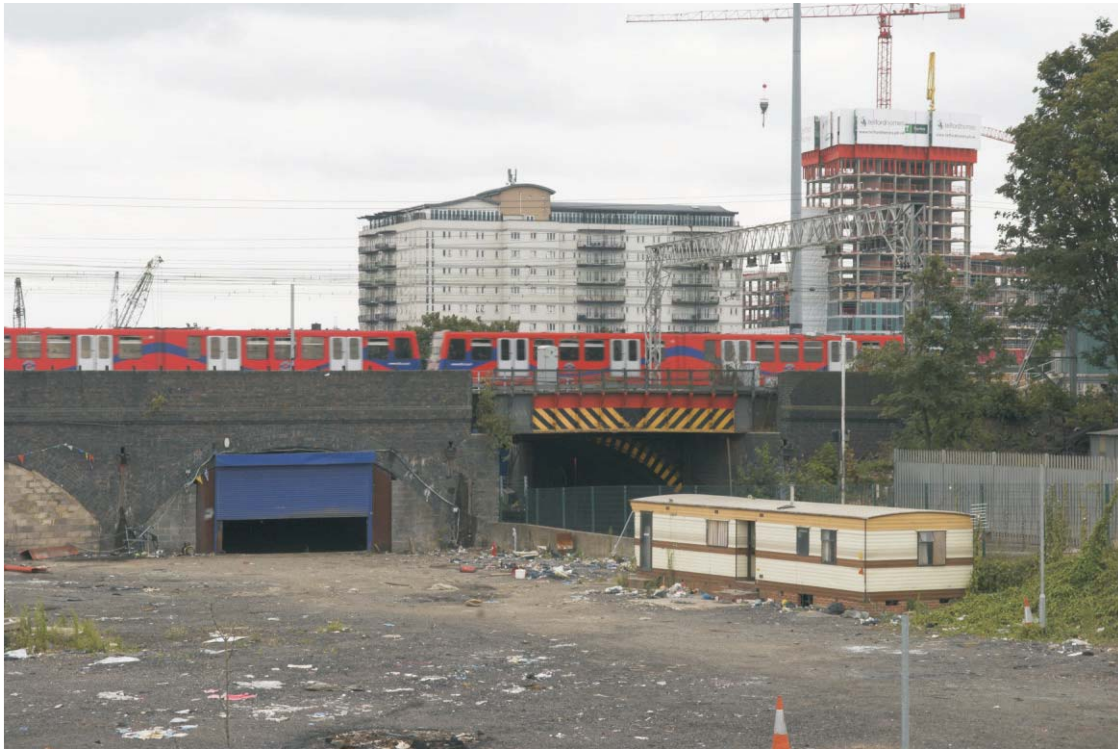
Plate 33 The northern side of the GER Stratford viaduct, looking south
