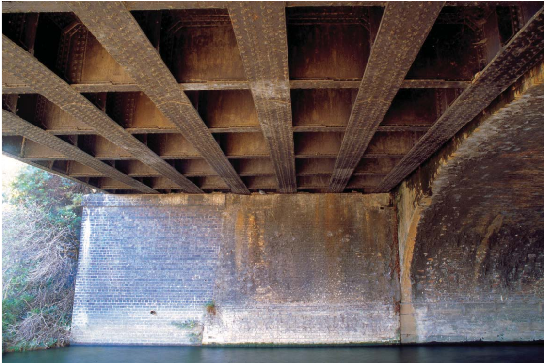
Plate 60 The southern end of the western abutment of the GER bridge over the City Mill River, looking south-west
