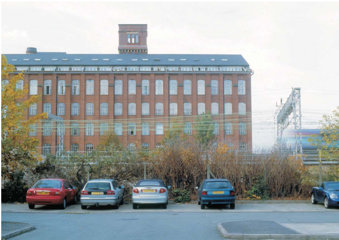
Plate 2 The low brick viaduct carrying the GER past the former Bryant and May match factory, looking north
