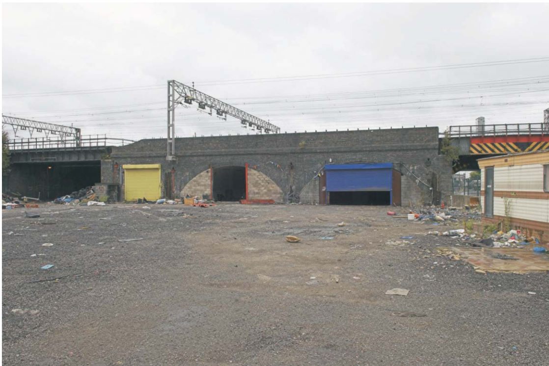
Plate 44 The north-facing external elevation of the viaduct arches between Pudding Mill Lane and Marshgate Lane, looking south-east
