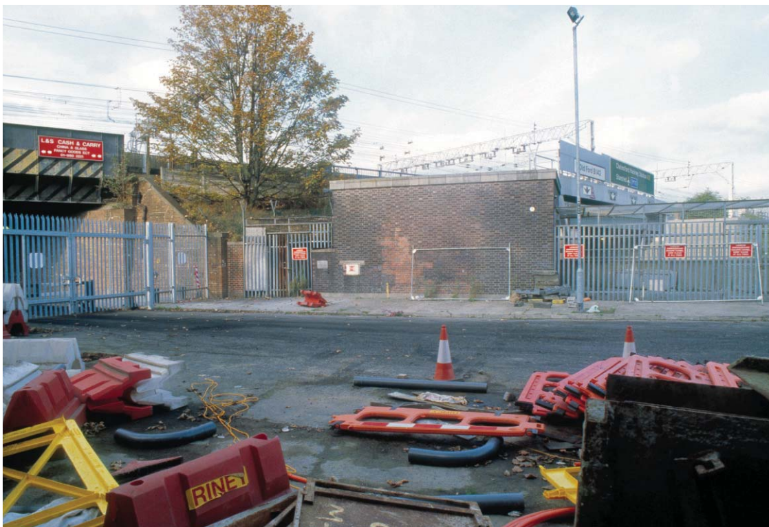
Plate 4 The emergency exit for the Central Line, adjacent to Wick Lane bridge, looking north-east
