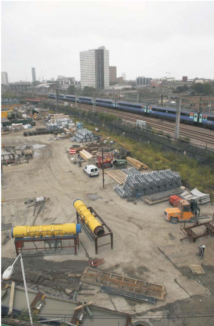
Plate 11 The GER embankment between Warton Road and Carpenter's Road, looking north-east
