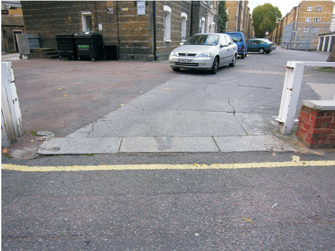
Fig 8 Looking north-west at the paving where the south end of Peabody Avenue meets Turpentine Lane. Note the scars of a former double-leaf gate (posts on either side and central scar where the two leaves of the gate would meet when closed).
