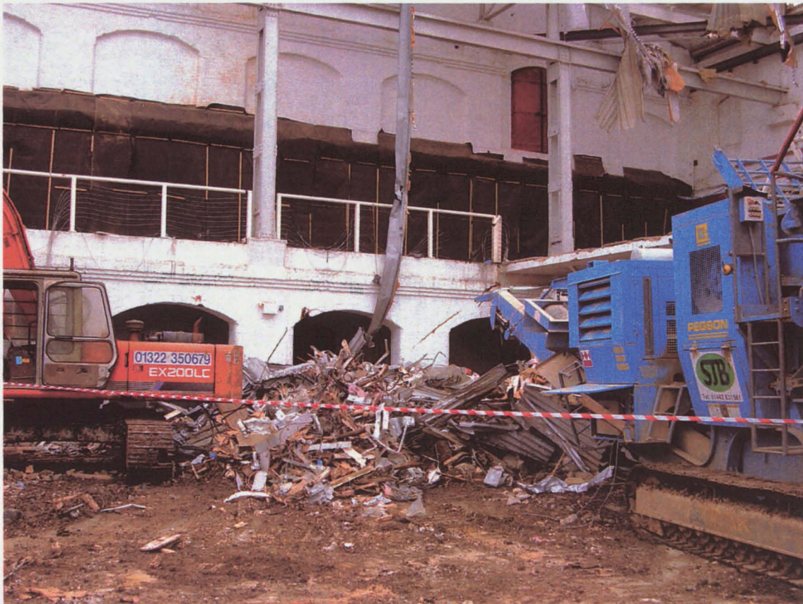
Fig 12 Photograph showing arched brick arcade, looking south-east
