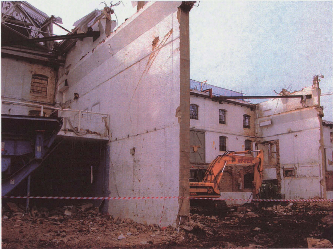
Fig 9 Photograph showing partition wall between 'O' and 'N' looking south-west
