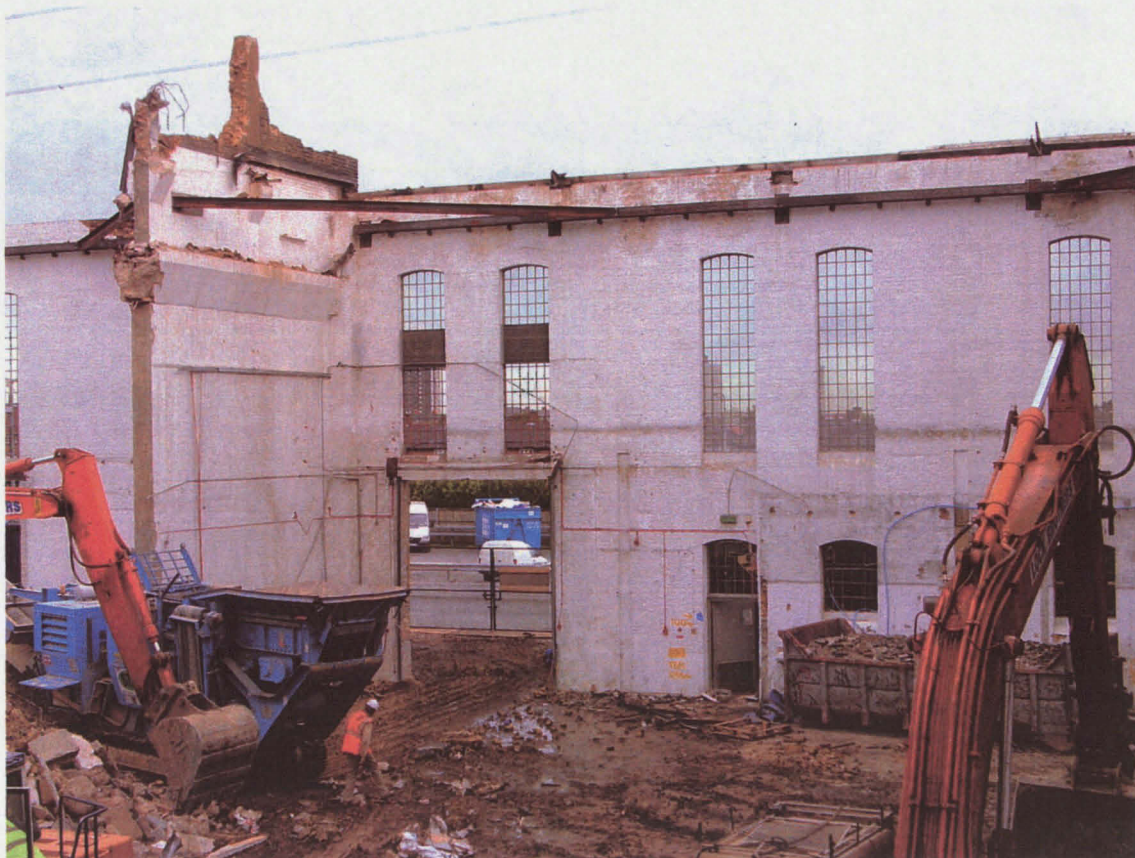
Fig 8 Photograph showing northern elevation, windows looking north-west
