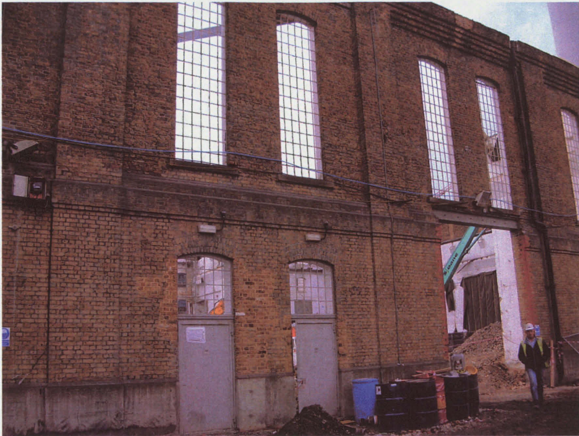
Fig 7 Photograph showing northern elevation, looking south-west
