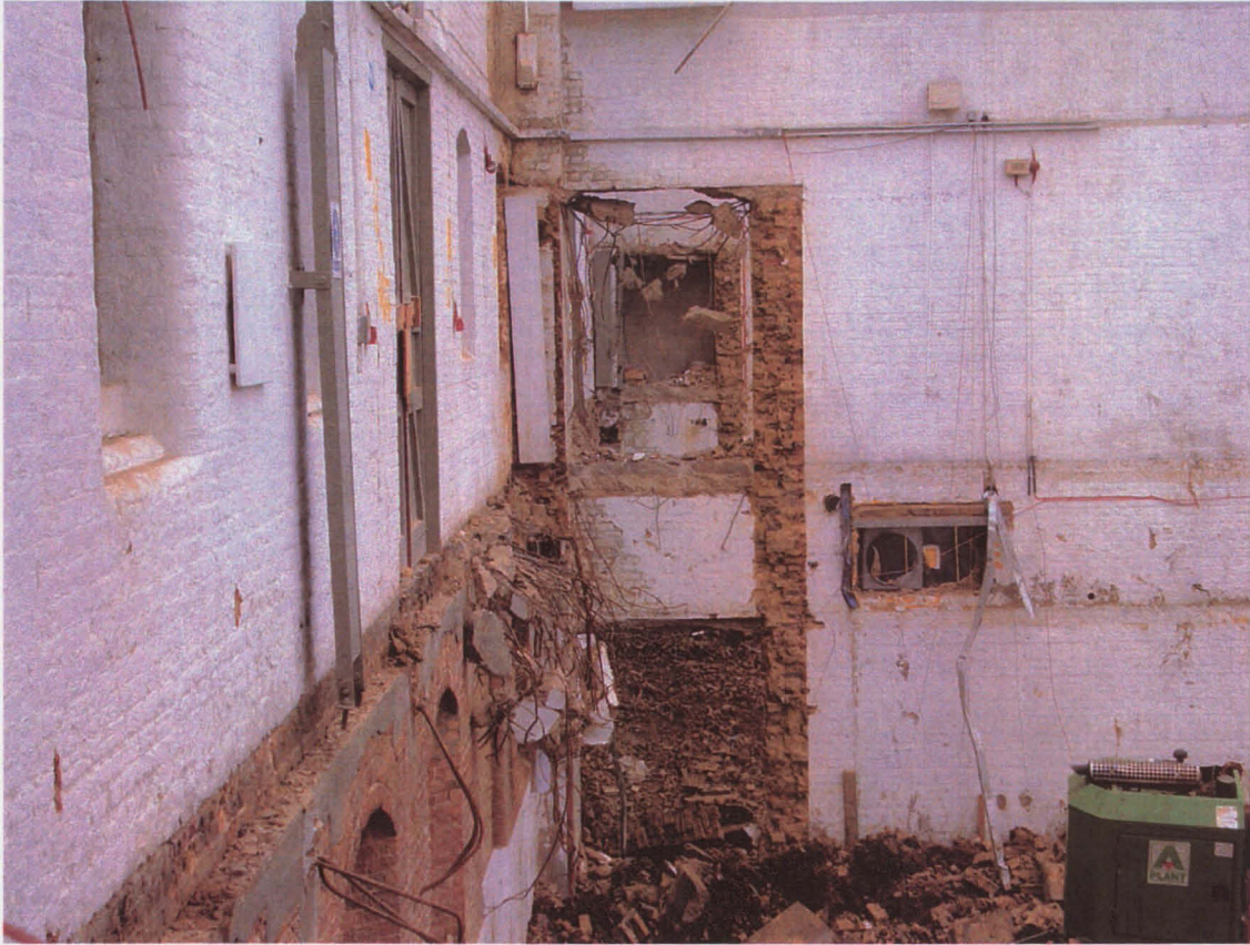
Fig 11 Photograph showing demolished mezzanine, looking west
