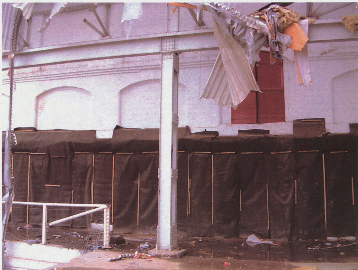
Fig 14 Photograph showing riveted girder in 'N', looking north-east
