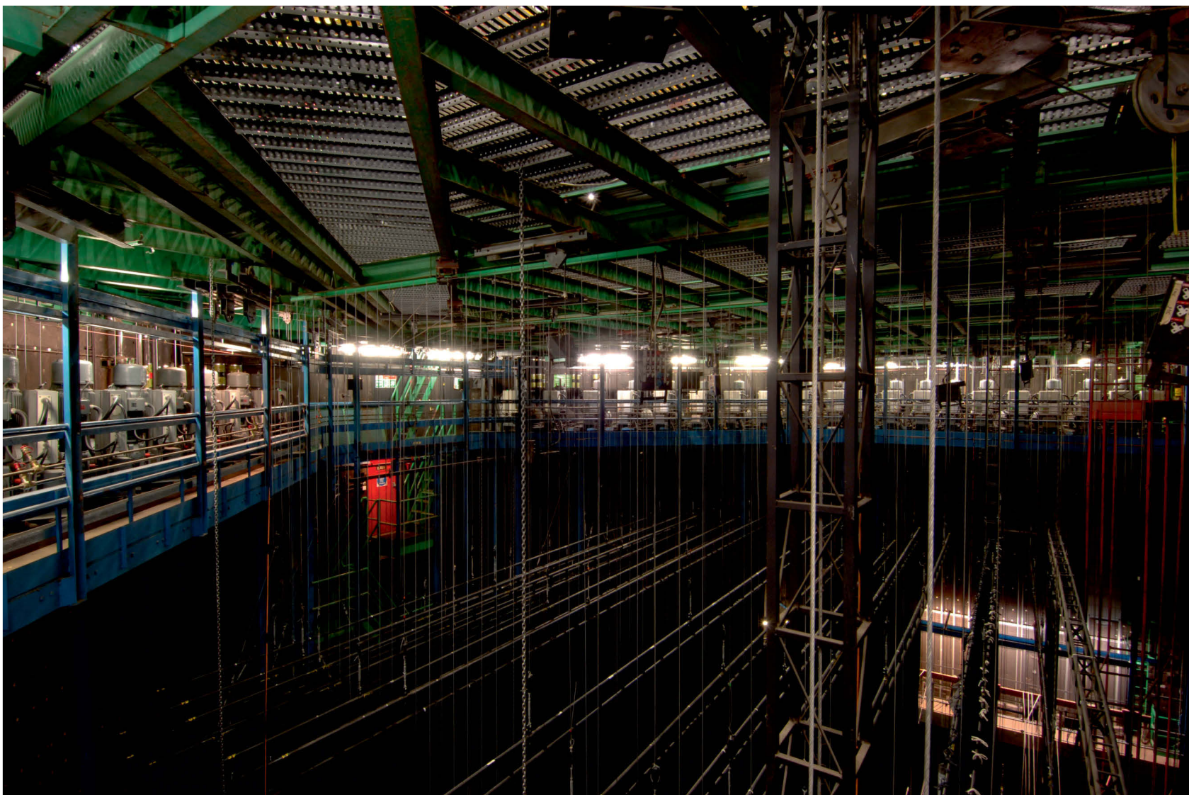
Fig 16 Looking SE (from downstage, stage right, looking toward the centre back of the loft) at sub-grid level, showing the bars hanging in the fly loft below the grid – the windlass counterweight hauling lines run down from loft blocks at the back of the loft, in front of the stairs at centre left
