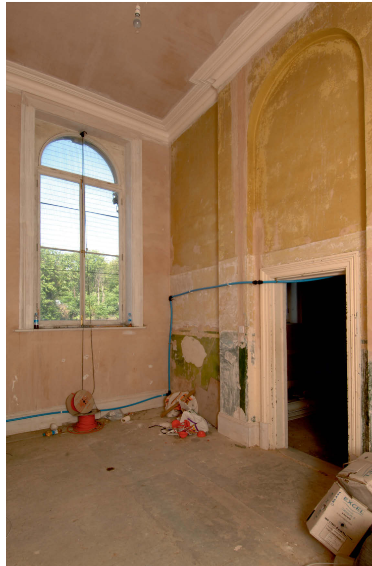
Fig 43 Task 24 far south western ground floor room in the south tower showing the green wall paint, looking west
