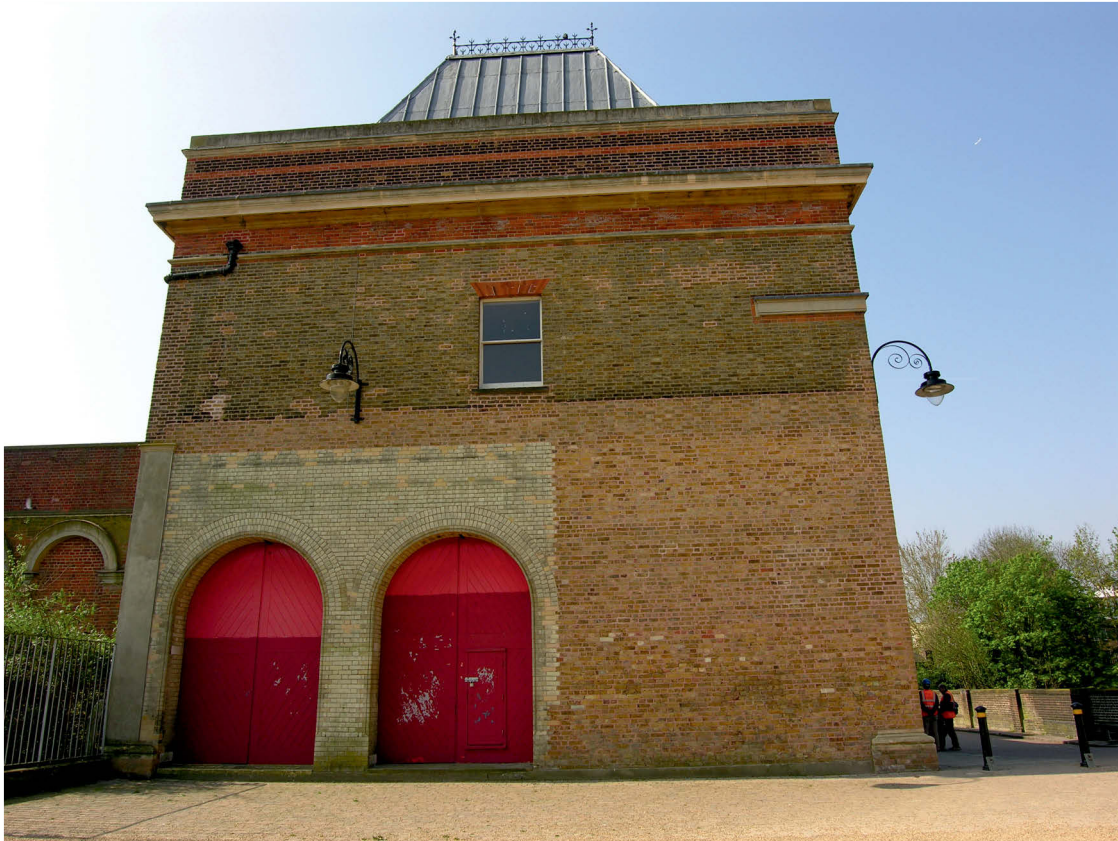
Fig 8 The north tower, north façade, looking south
