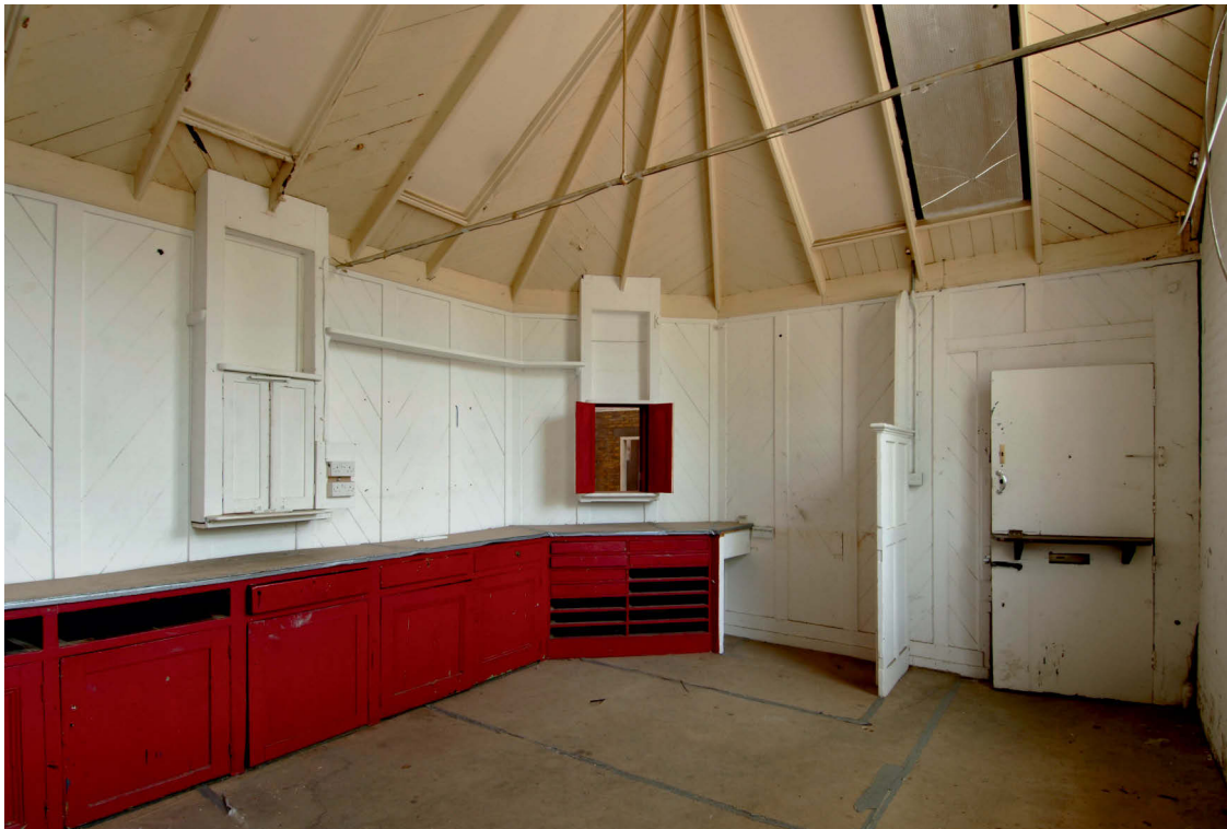
Fig 35 Task 18, internal view of the timber ticket office, looking south
