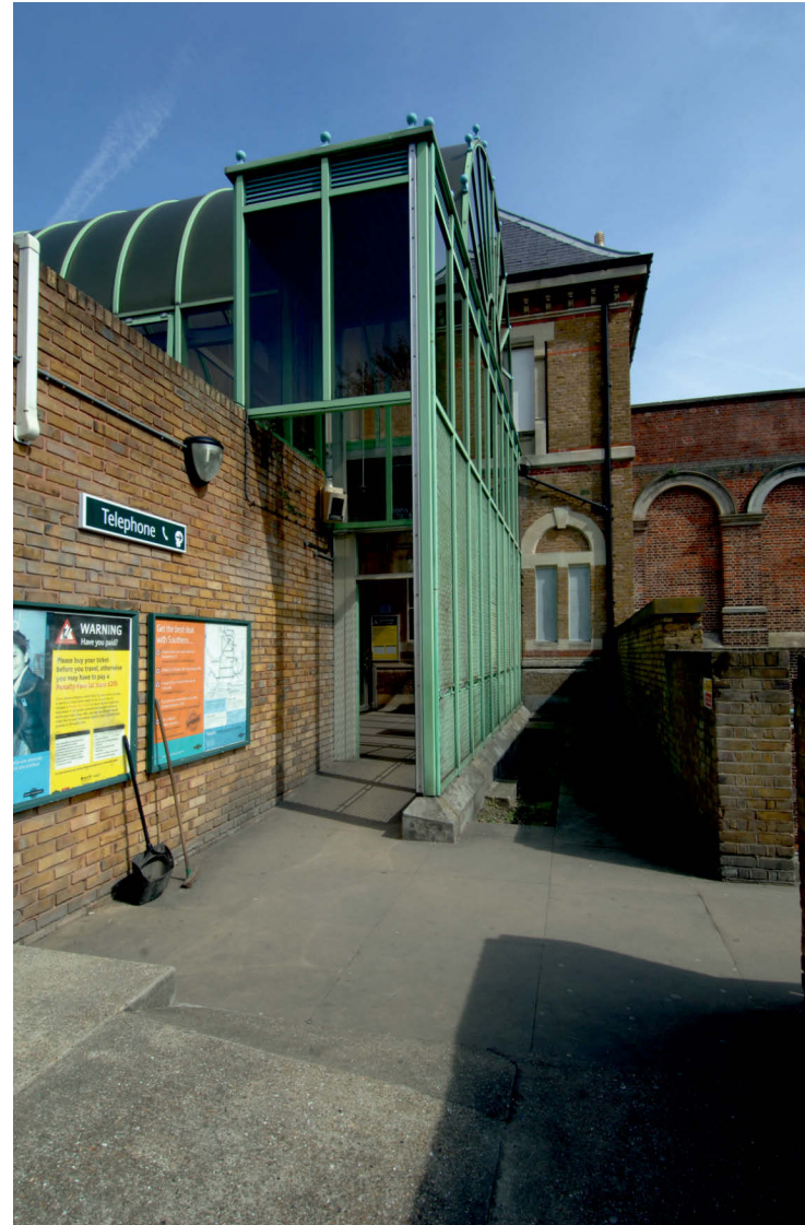
Fig 21 Task 4 south external wall of the south tower behind the entrance hall, looking north
