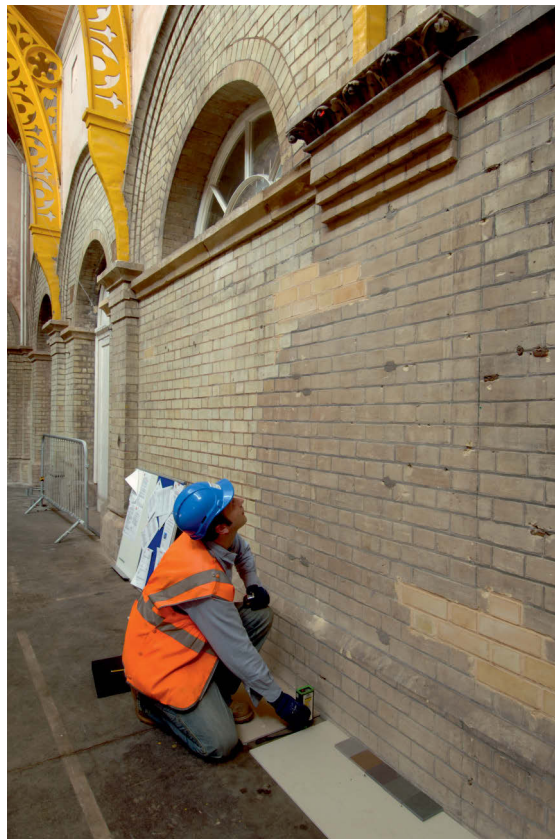
Fig 11 The decorated floating corbel, on the eastern wall of the 19th century ticket hall
