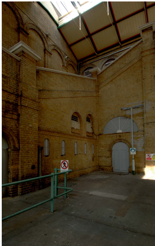
Fig 47 Task 27, North facing façade below staircase on Platform 3, looking west
