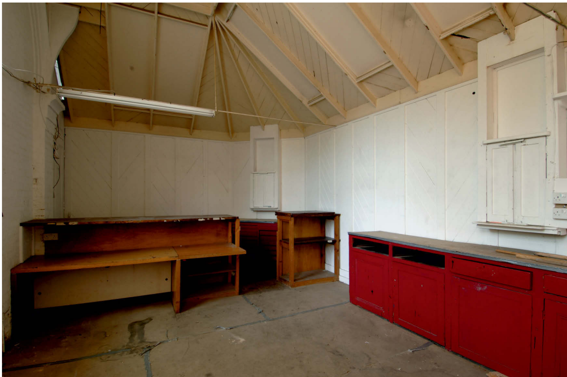
Fig 37 Task 18, internal view of the ticket office, looking north
