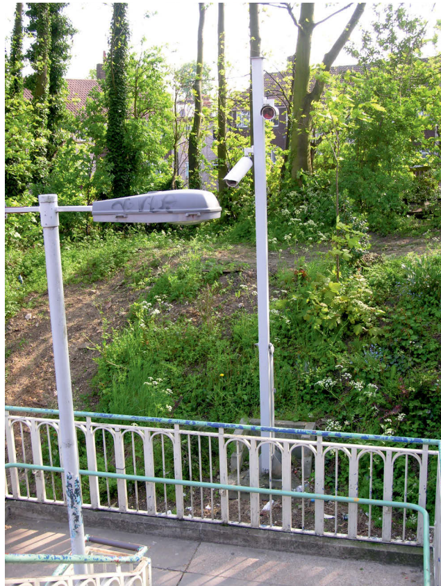
Fig 24 Task 7 CCTV camera pole and base, looking south
