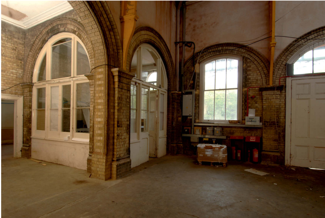
Fig 40 Task 20 glazed timber partitions to room at south end of ticket hall
