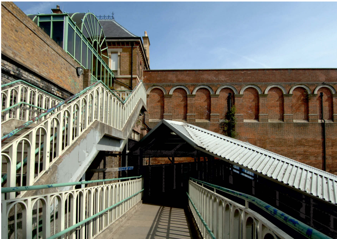
Fig 23 Task 6 stairs to footbridge looking north
