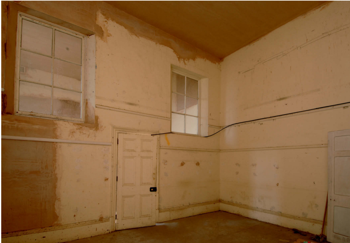
Fig 46 Task 25, southern windowed partition wall, looking south west
