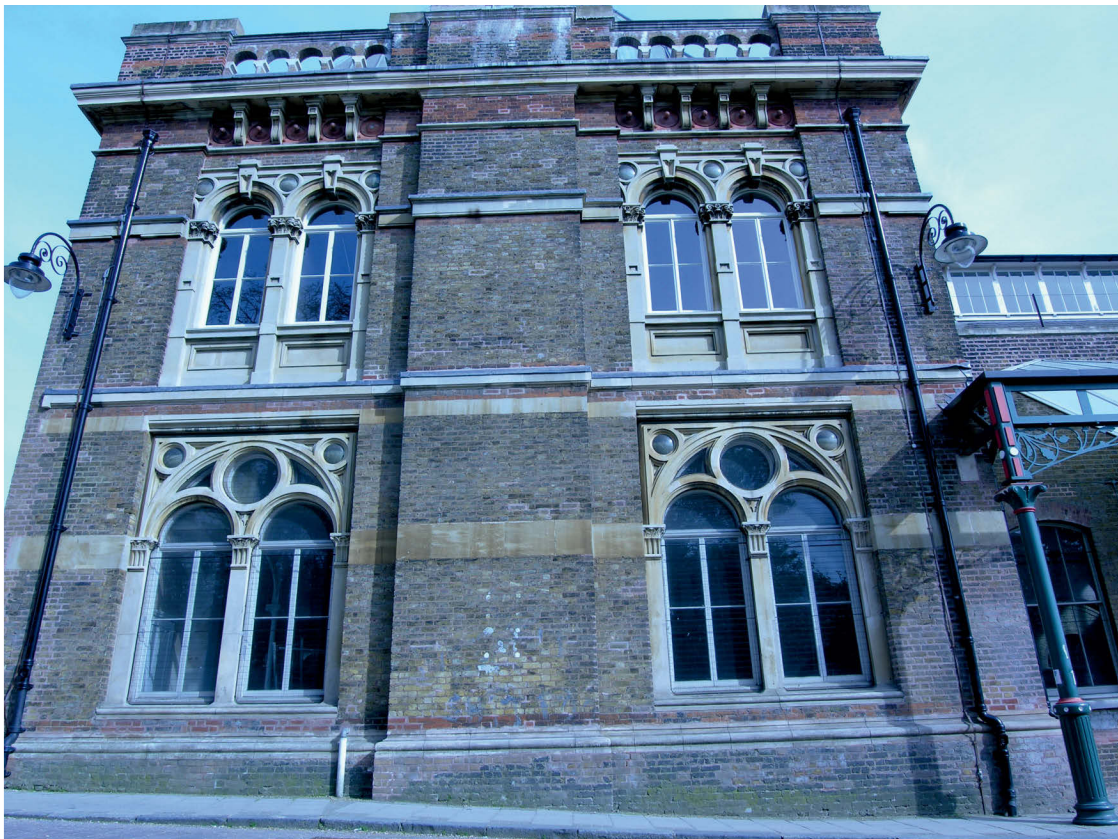
Fig 9 The north tower, west façade, looking east
