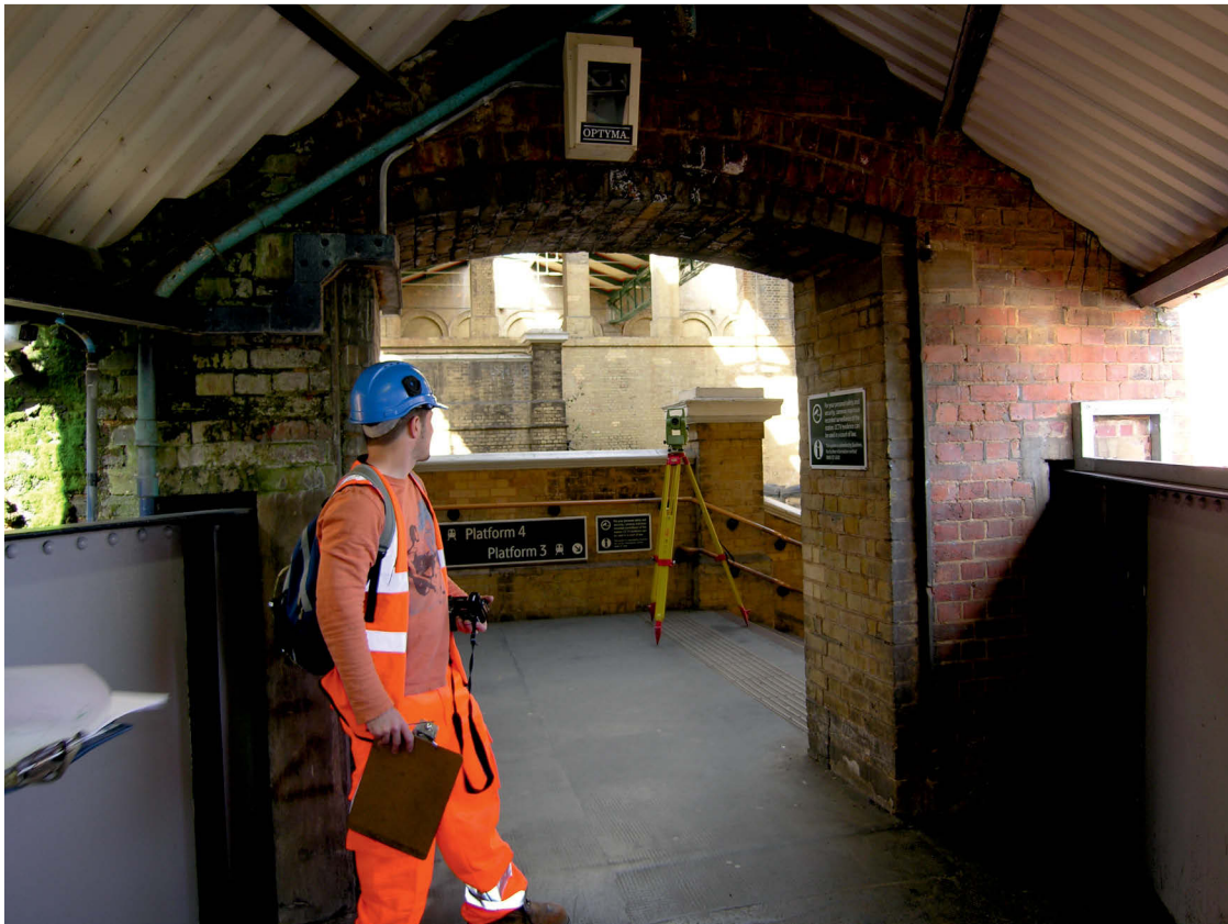
Fig 30 Task 12 doorway in south wall of main building connecting the footbridge to Platform 3, looking north
