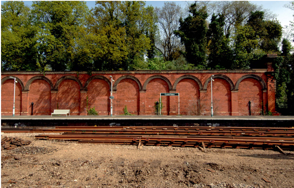
Fig 26 Task 9 the northernmost wall on Platform 4, looking north
