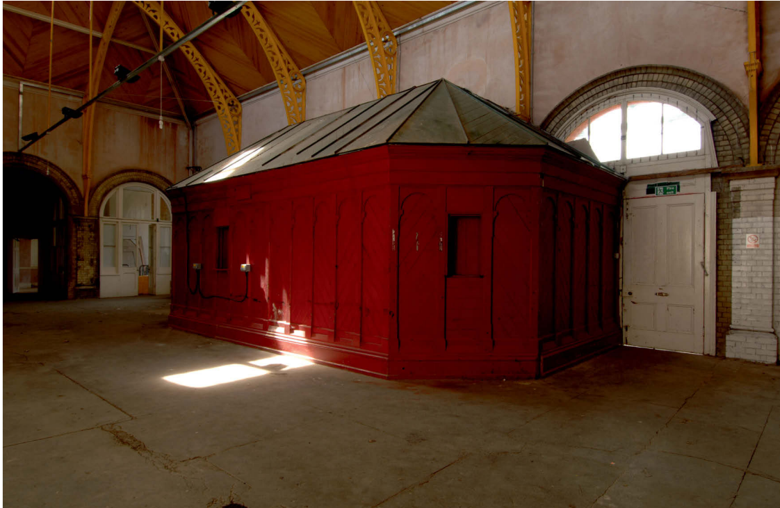
Fig 34 Task 18 the timber ticket office, looking west with hall entrance door
