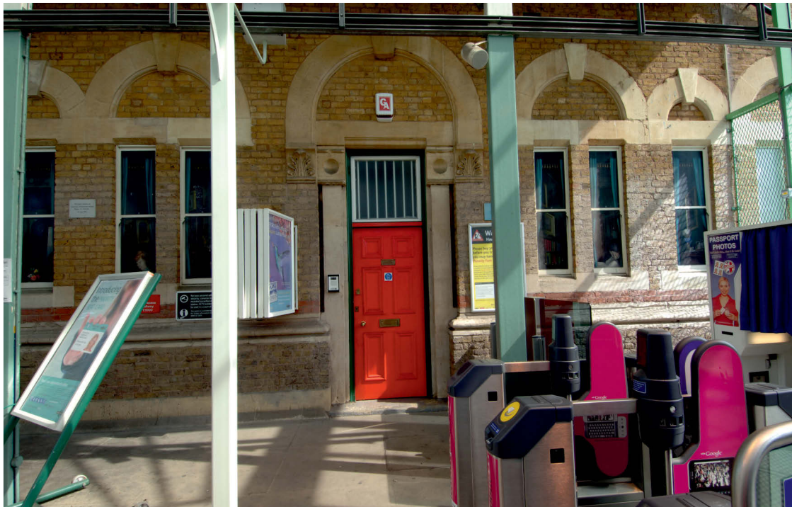
Fig 13 Southern façade of the south tower, looking north
