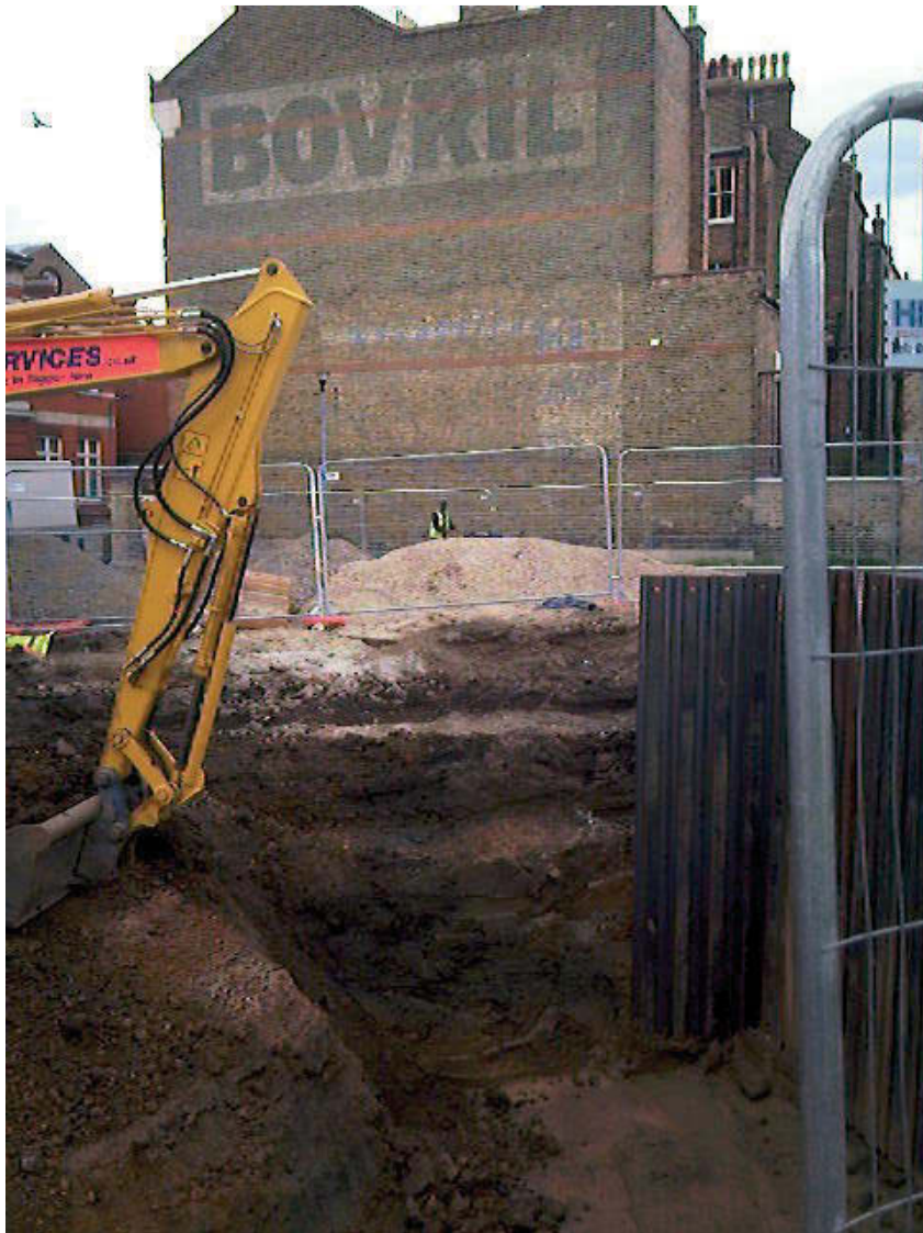
Fig 4 View to east showing pump room trench section
