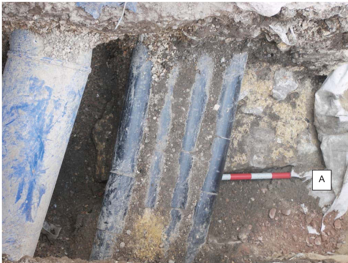
Fig 10 City wall in LIV26, looking north. Wall context [6], earlier exposed in LIV16, continues beneath ducts. Position "A" is the same in both photographs.
