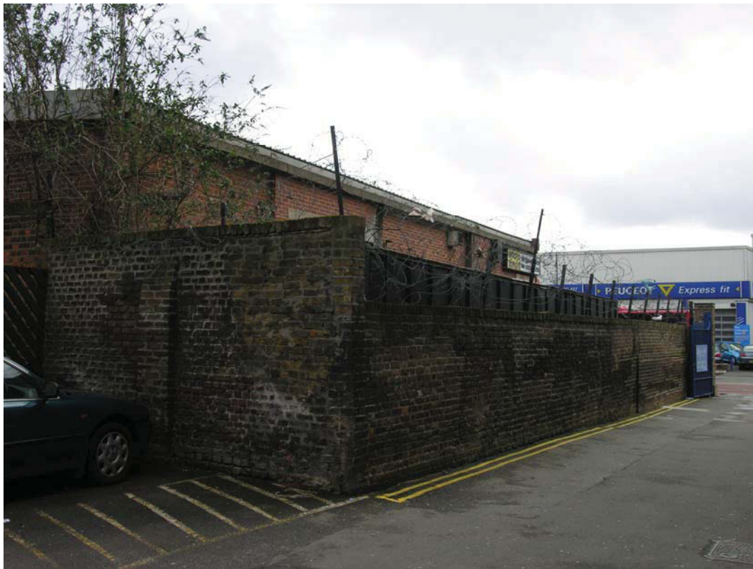
Fig 5 The earliest part of the cemetery wall, (2) left and (1) right, near Mile End Road, looking south-east (MoLAS)
