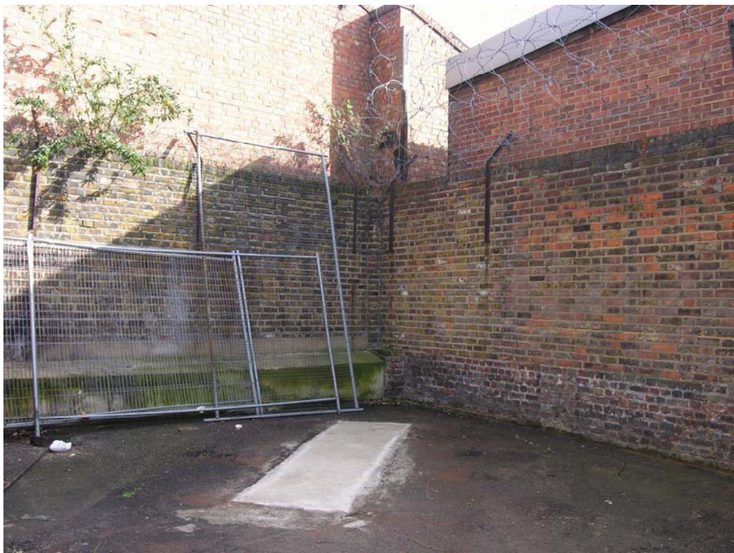
Fig 6 An internal corner of the wall, (3) left and (2) right, showing different ground levels and rebuilds, looking south-east (MoLAS)
