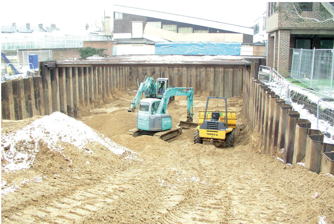
Fig 5 The groundwork in progress
