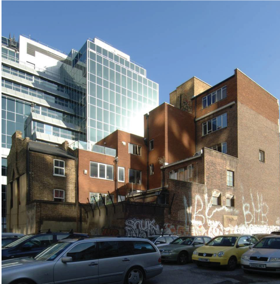
Fig 13 The back and south side of the building, looking North East
