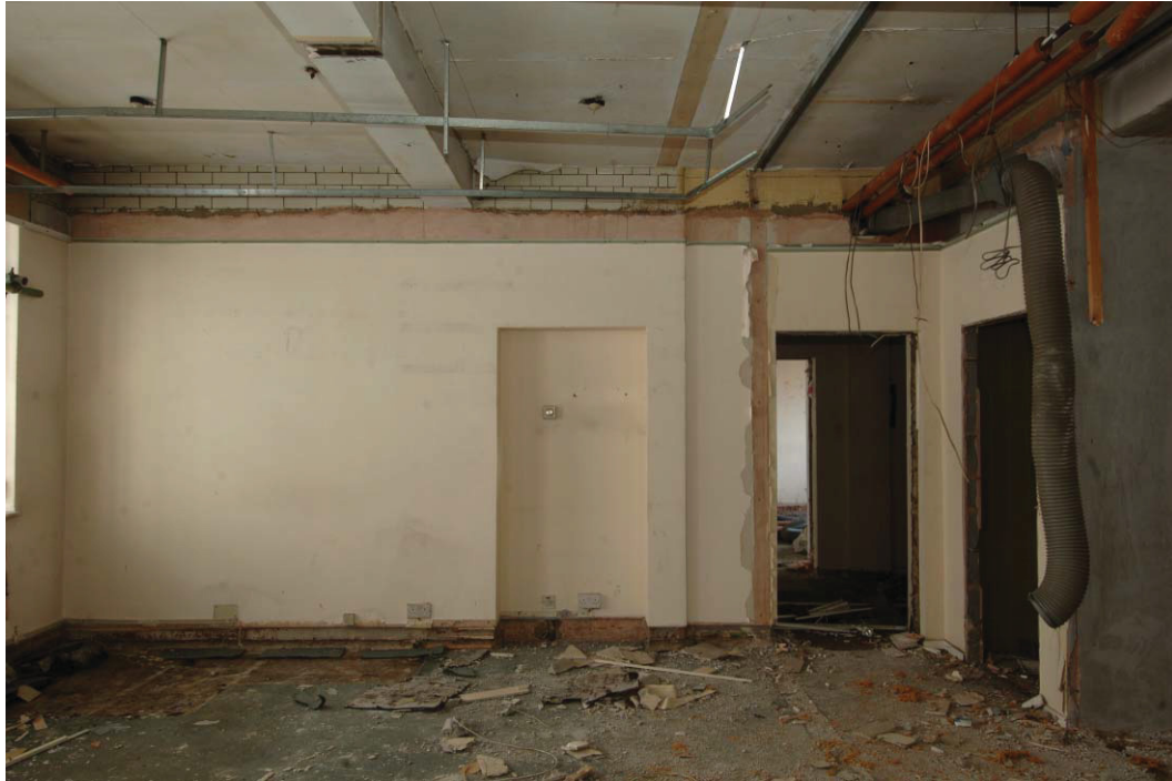
Fig 17 The 3rd floor front room at 46 Blackfriars Road, looking North
