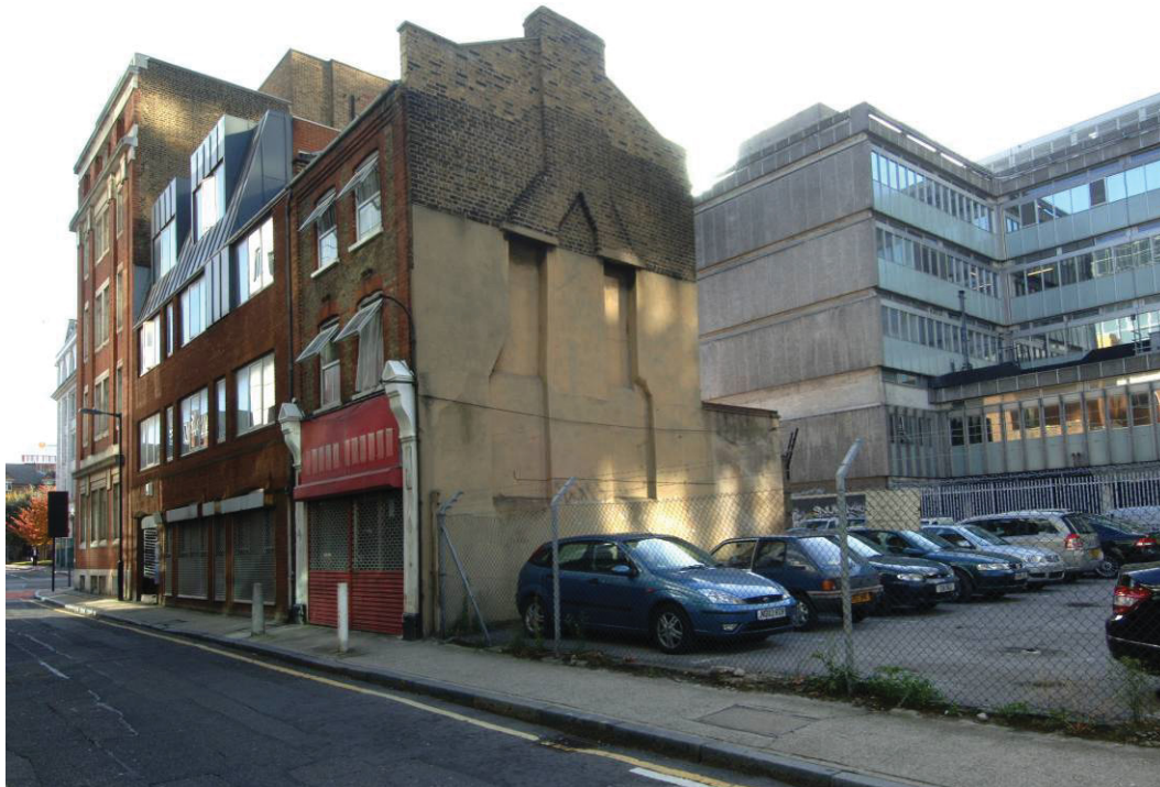
Fig 14 View of Meymott Street, looking South West
