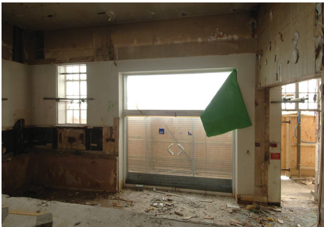
Fig 18 The ground floor front room at 46 Blackfriars Road, looking East
