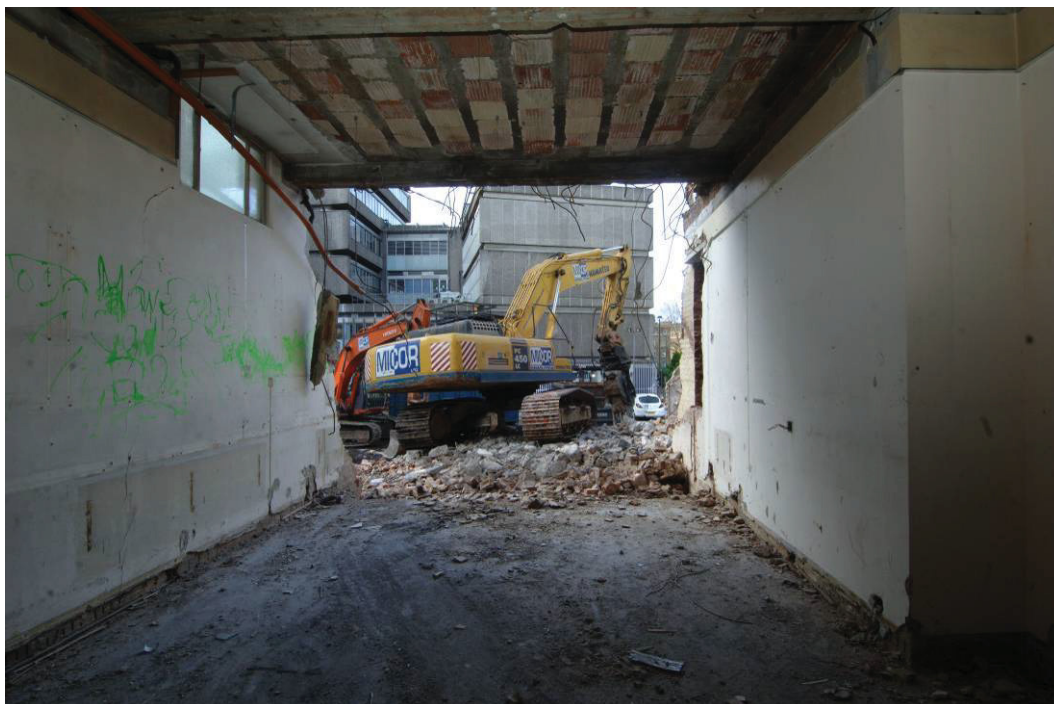
Fig 16 The ground floor room at 47 Blackfriars Road, looking West
