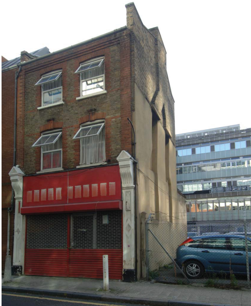
Fig 15 The front of 7 Meymott Street, looking West
