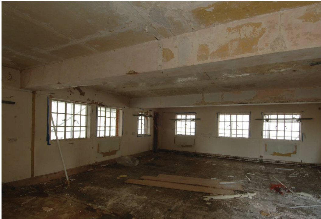
Fig 19 The room on the 4th floor at 46 Blackfriars Road, looking East
