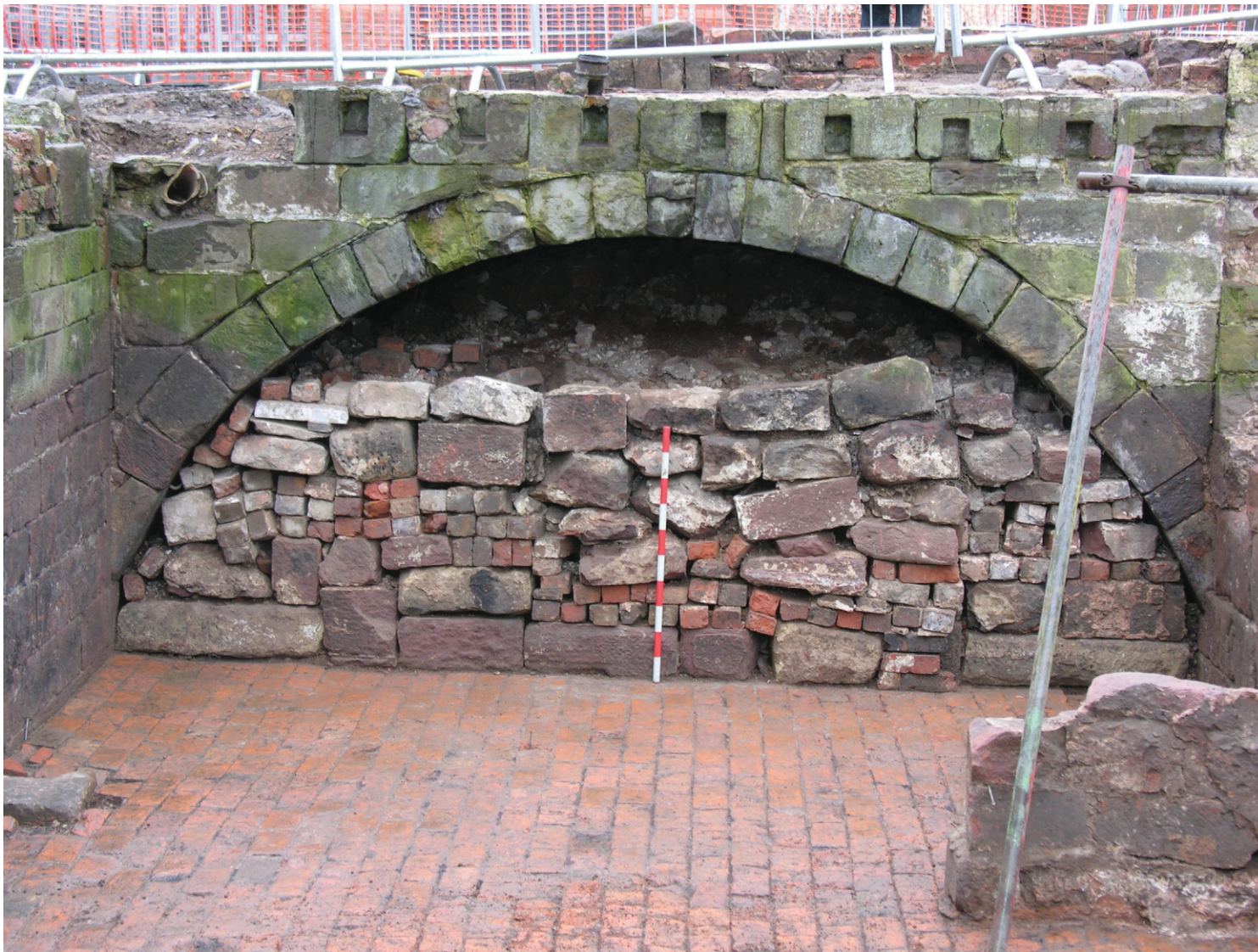
Fig 16 Photo of the western side of the bridge arch, showing the ramshackle blocking wall constructed during the 1960s out of demolition material (looking east)
