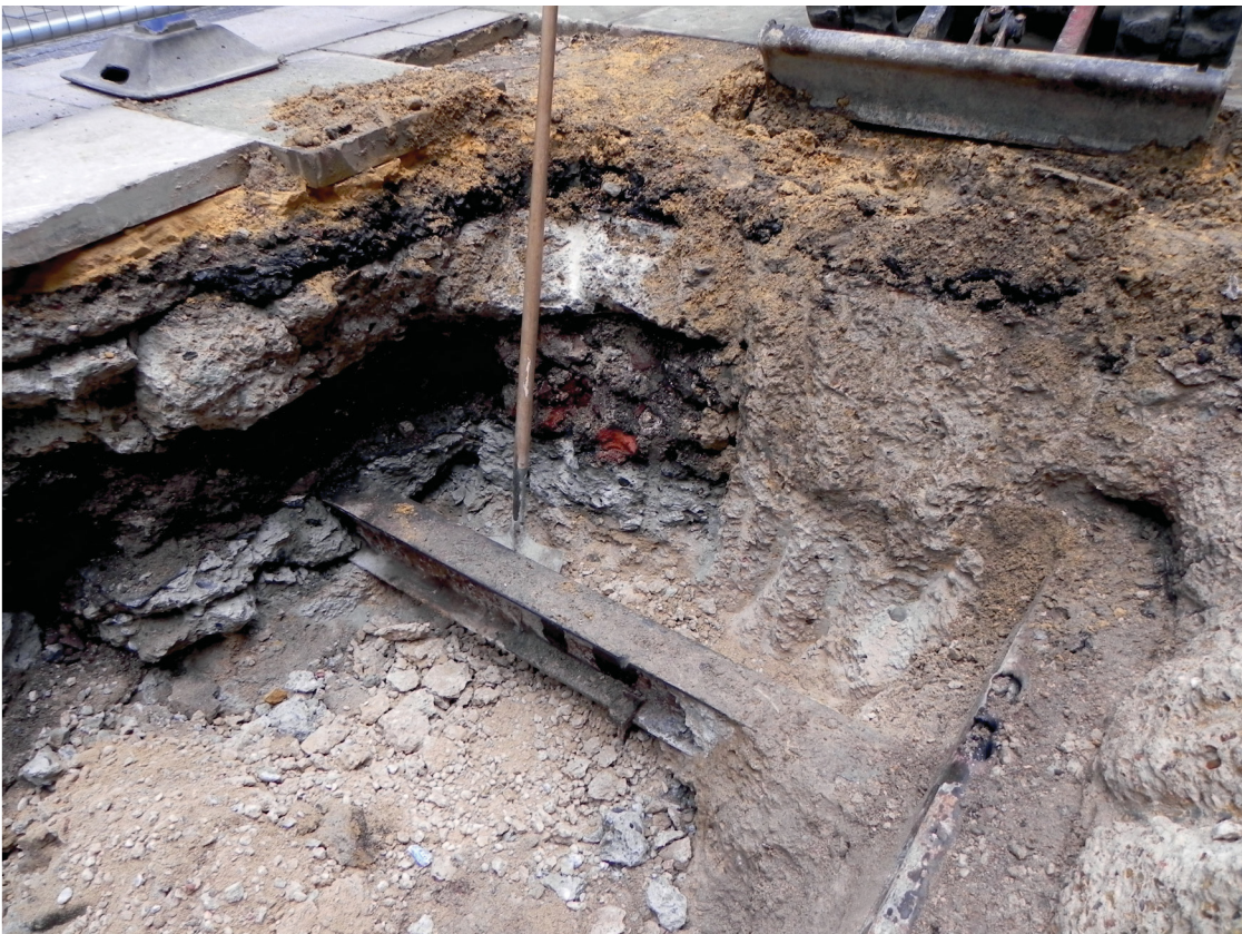
Fig 6 Photograph of excavation of toilet placement
