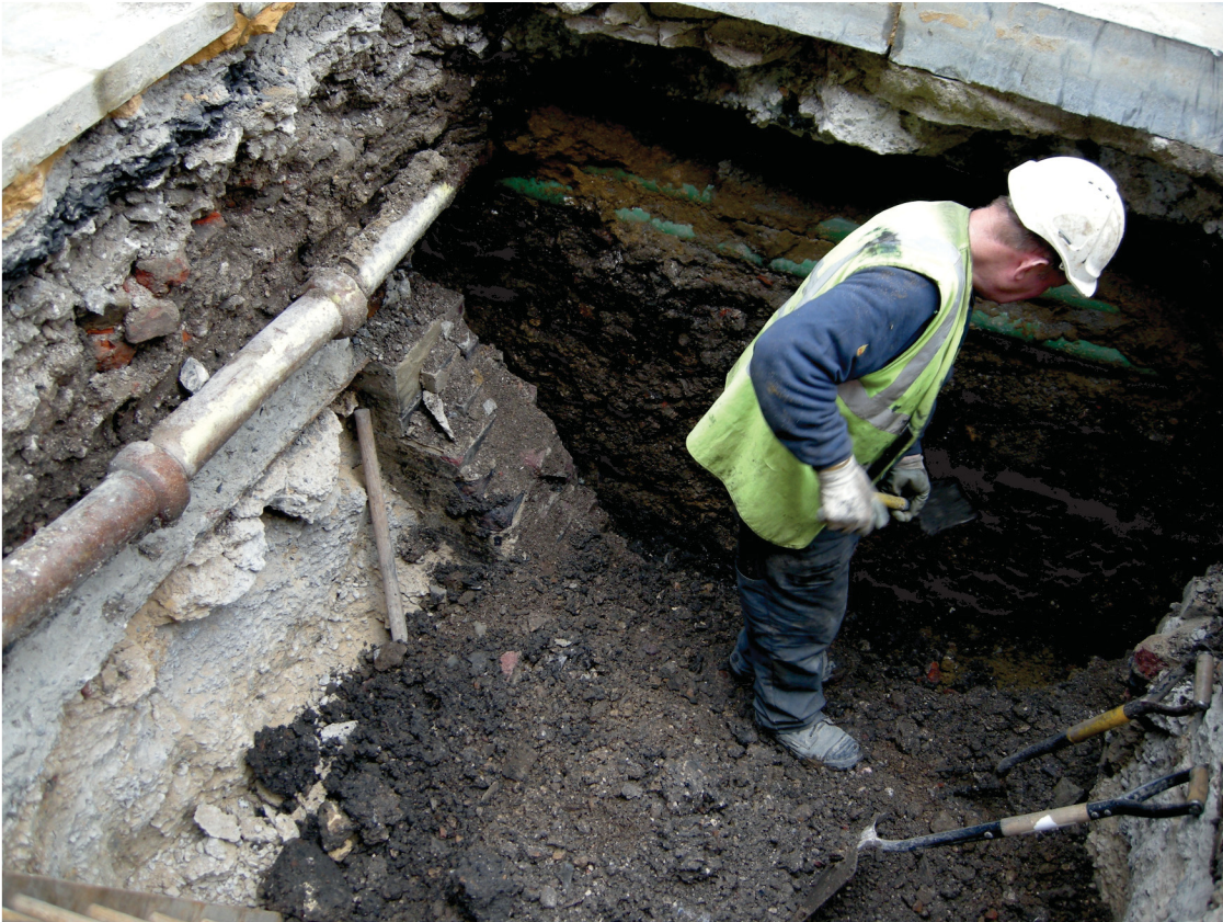
Fig 5 Photograph of dropshaft during excavation
