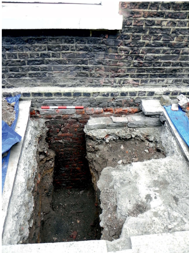
Fig 6 View of the external wall of the main Skinners' Hall building (looking north) with stepped brick footing [7] beneath the scale
