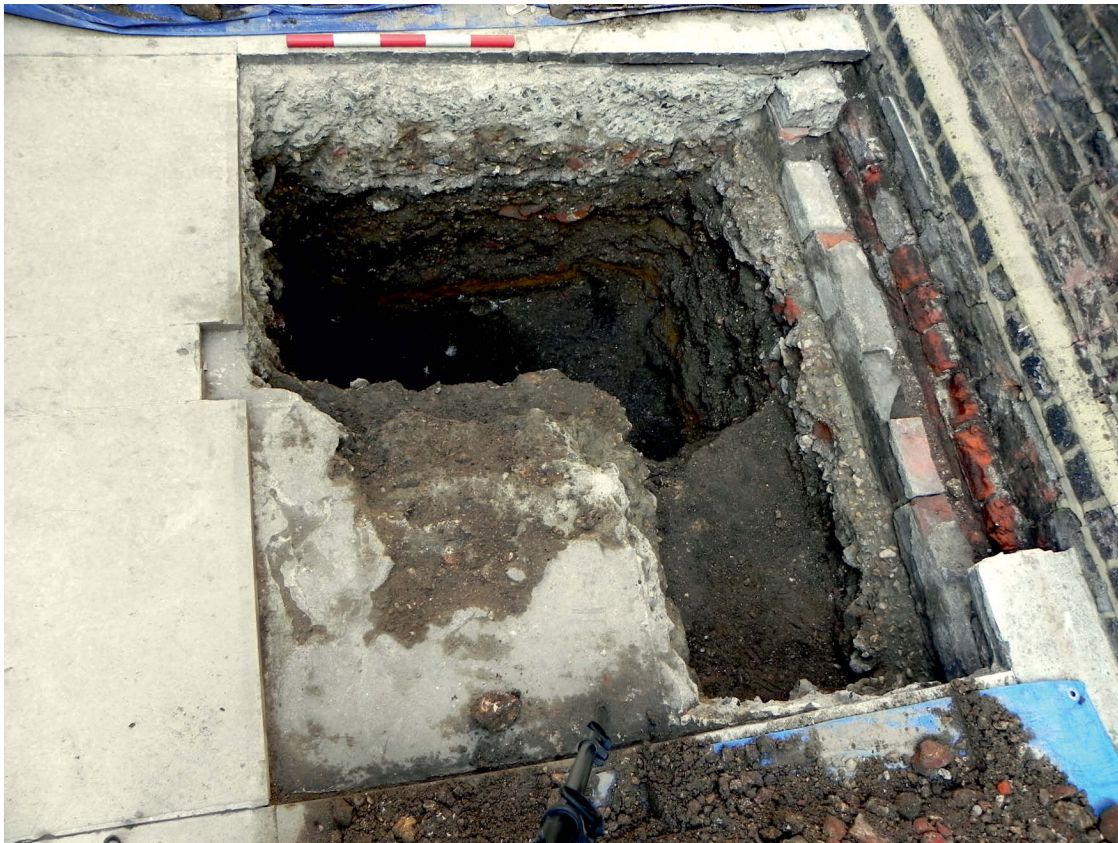
Fig 5 Overview of the trial pit (looking west)
