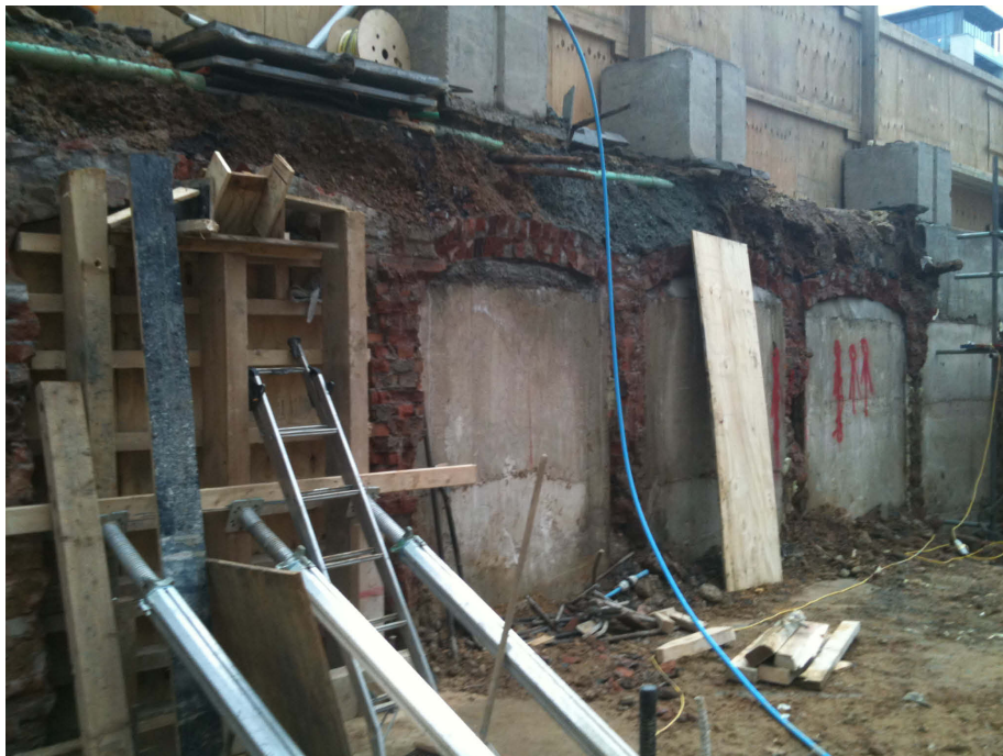
Fig 3 Infilled brick vaults
