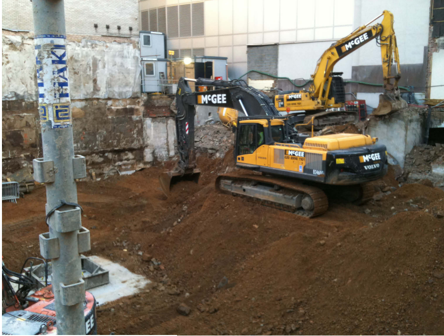
Fig 2 Ground reduction monitoring
