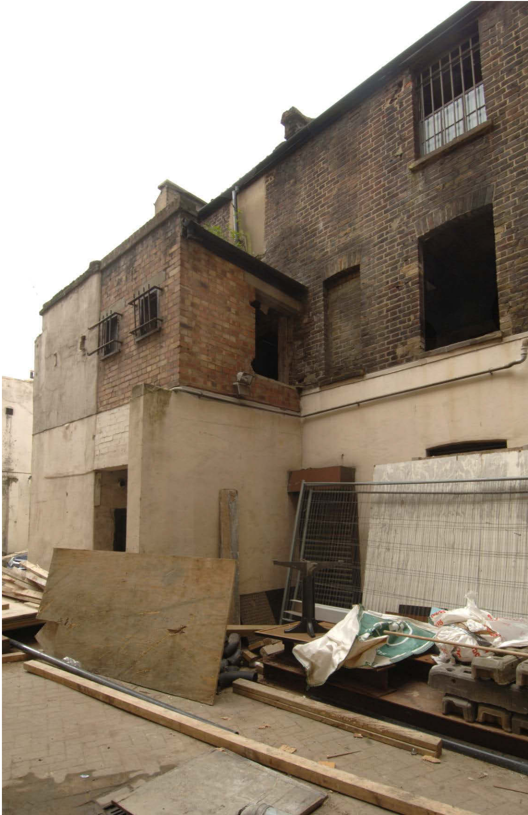
Fig 8 The back extension to 245 Long Lane, looking south-east
