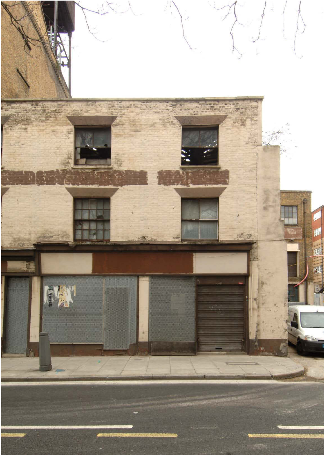
Fig 7 The front elevation of 243–245 Long Lane, looking north
