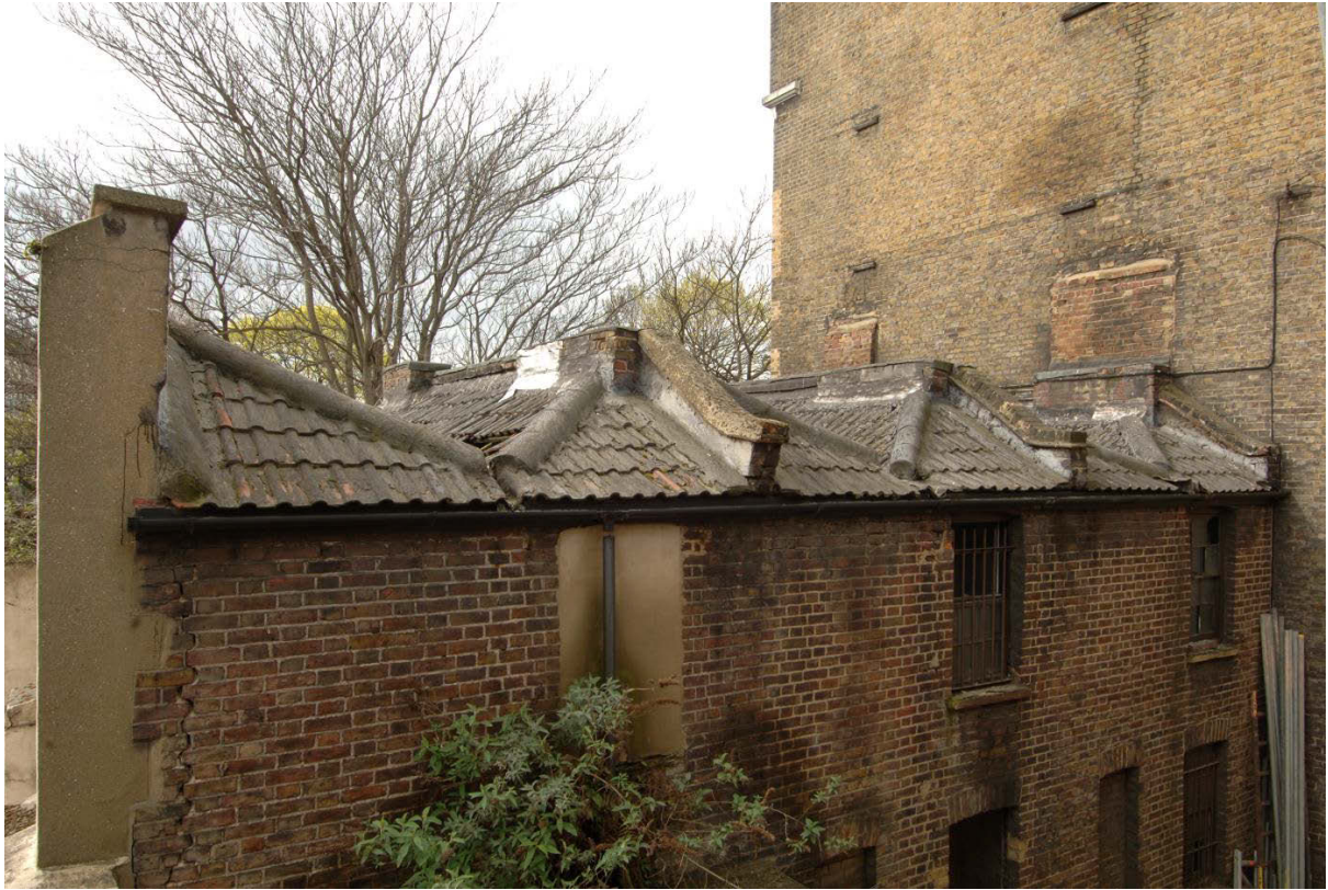
Fig 9 Detail of the roof of 241–245 Long Lane, looking south
