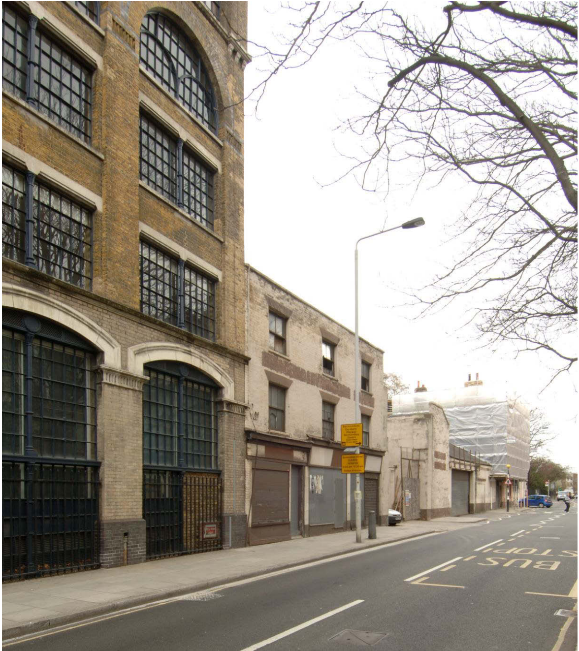
Fig 5 The street front of the building and its surroundings, looking east
