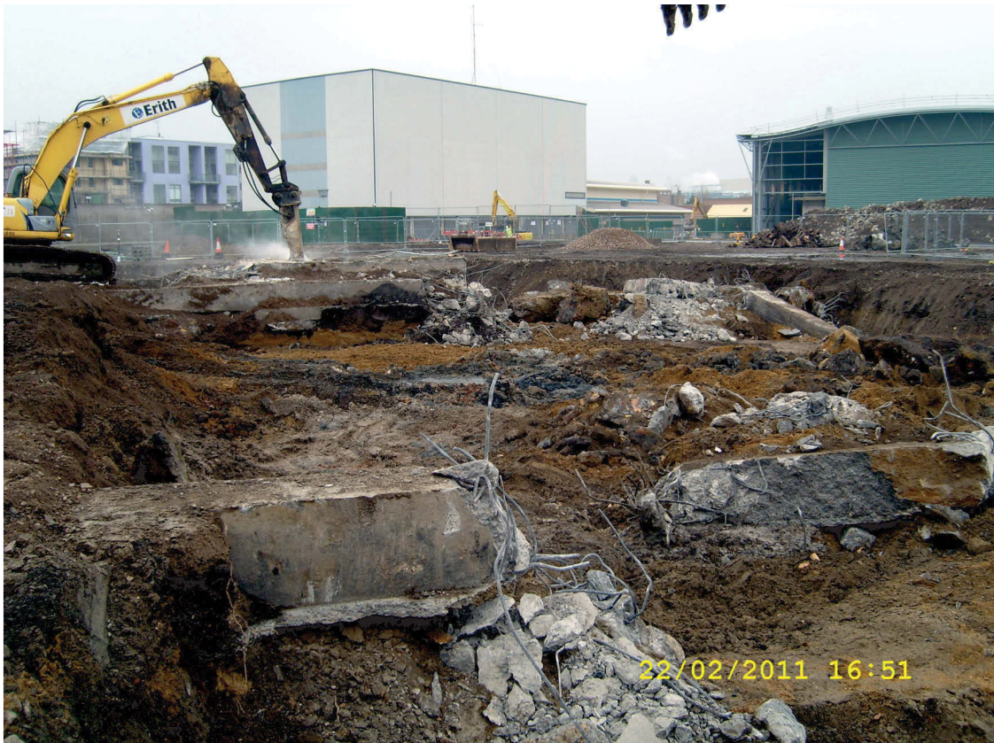
Fig 4 Site of former garage on south side of site, looking east
