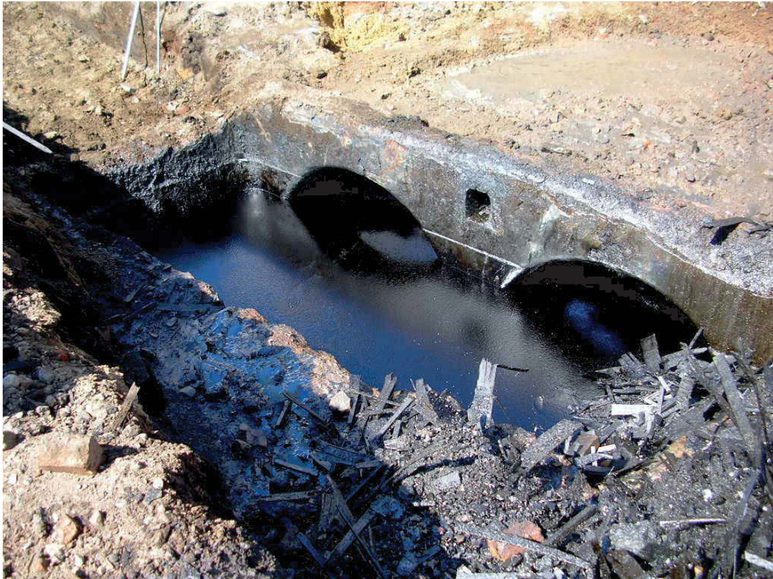
Fig 3 Purification tanks on north side of site, looking north
