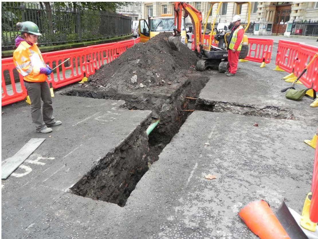
Photo 1: Western grout shaft trial trench. Telecommunications services (green cable) visible at centre. Facing south.
