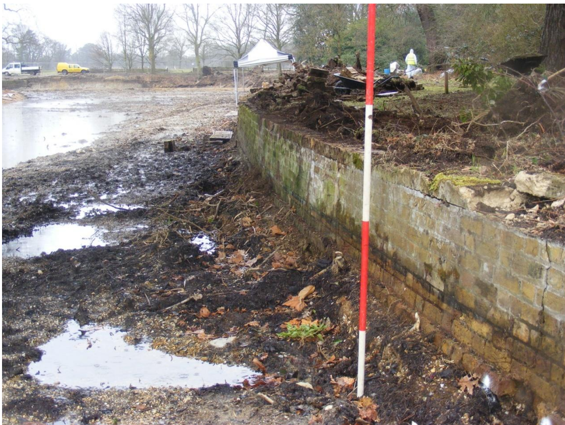
The retaining wall, looking to the north: Fig 15
