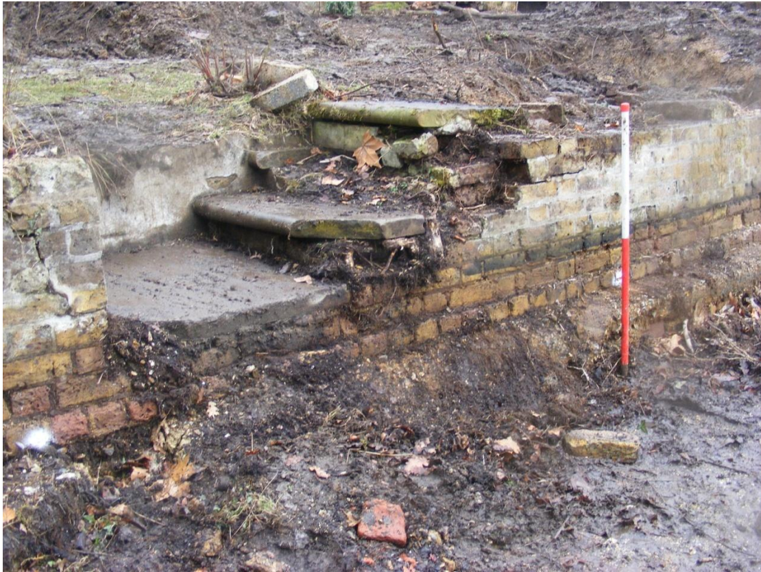
The retaining wall and steps adjacent to the boathouse: Fig 14
