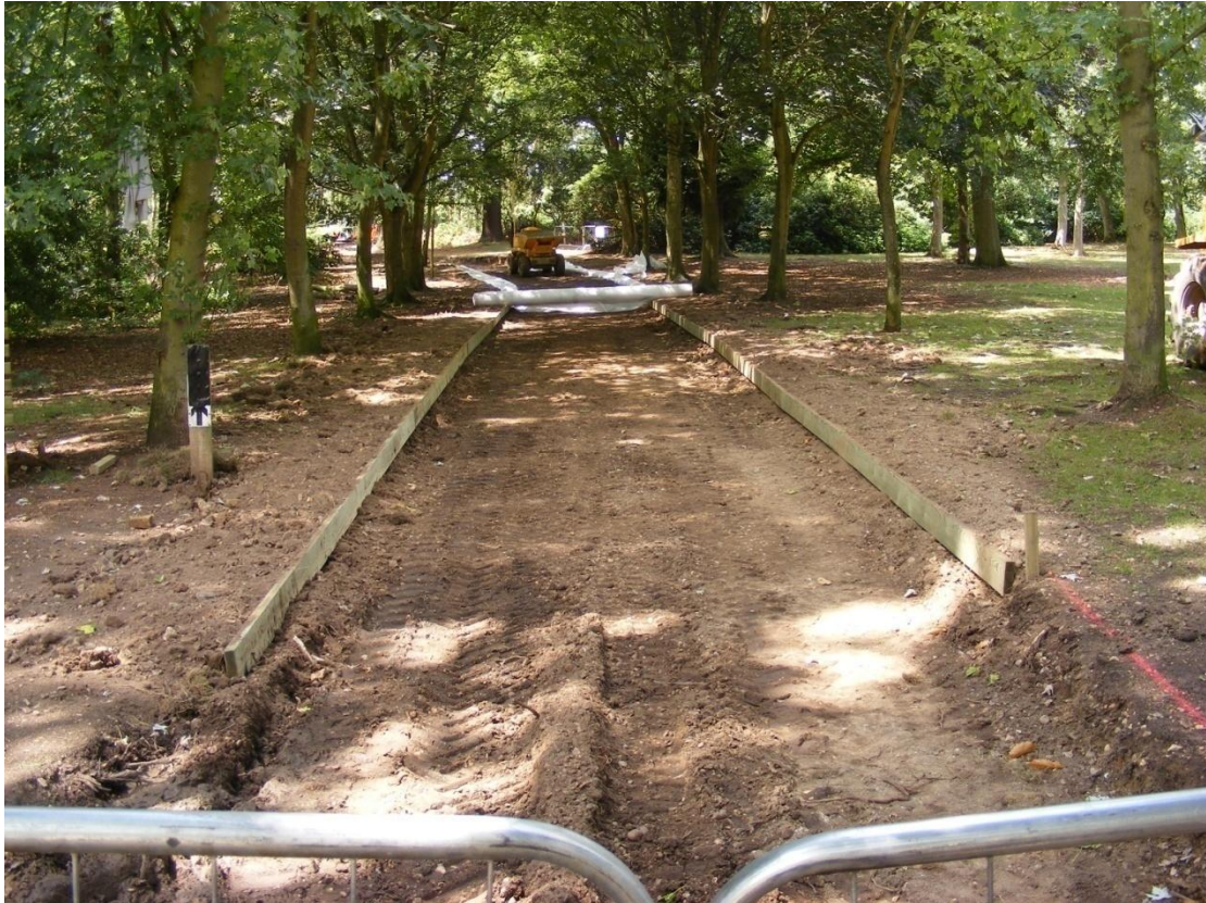
The footpaths during construction, looking towards the visitor centre: Fig 5
