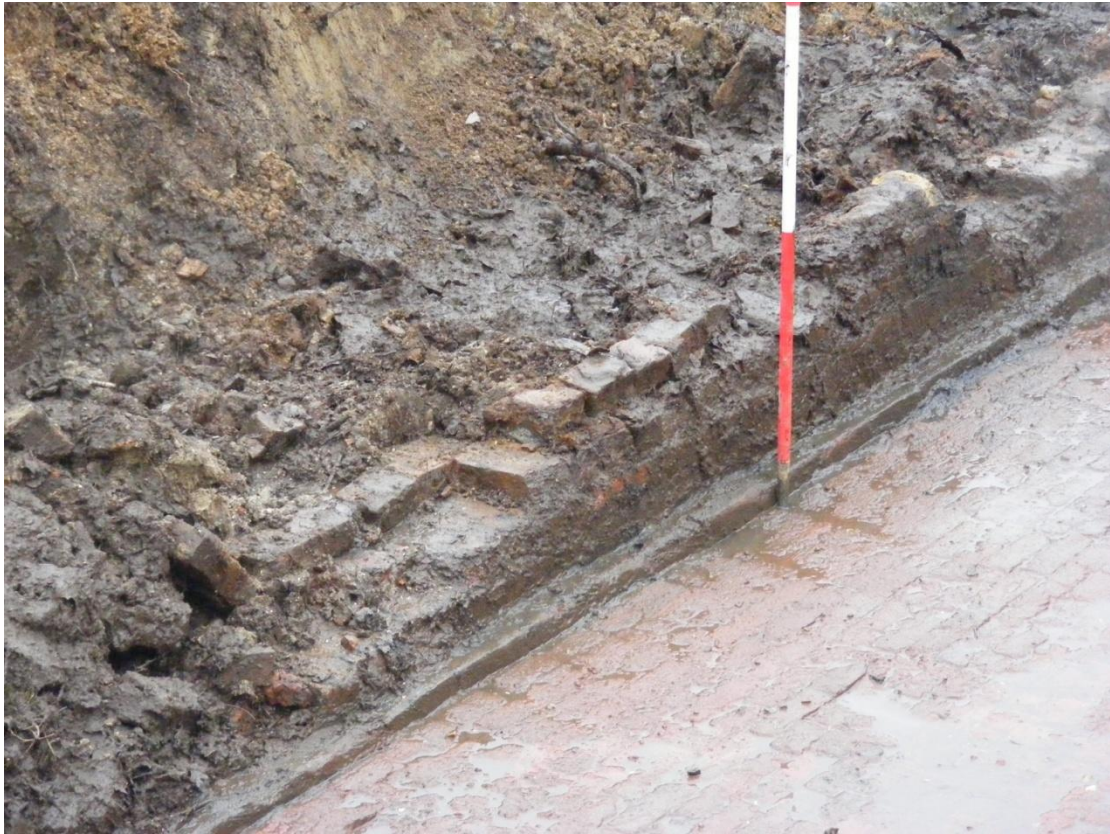
The south wall of the boathouse: Fig 12
