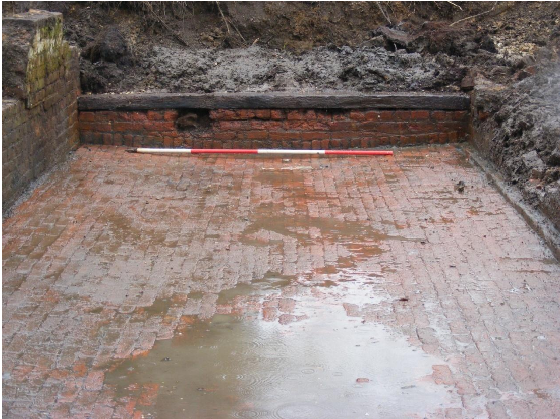
The rear wall of the boathouse: Fig 13
