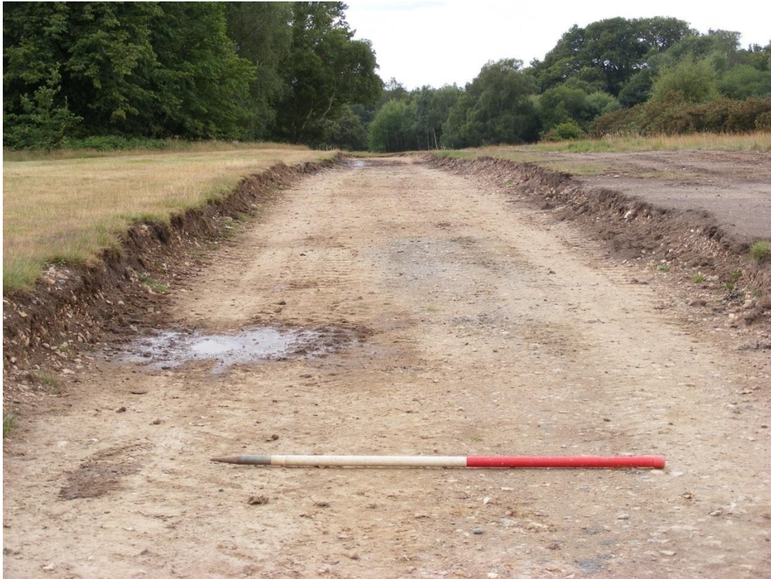
The footpaths during construction, looking to the south: Fig 4
