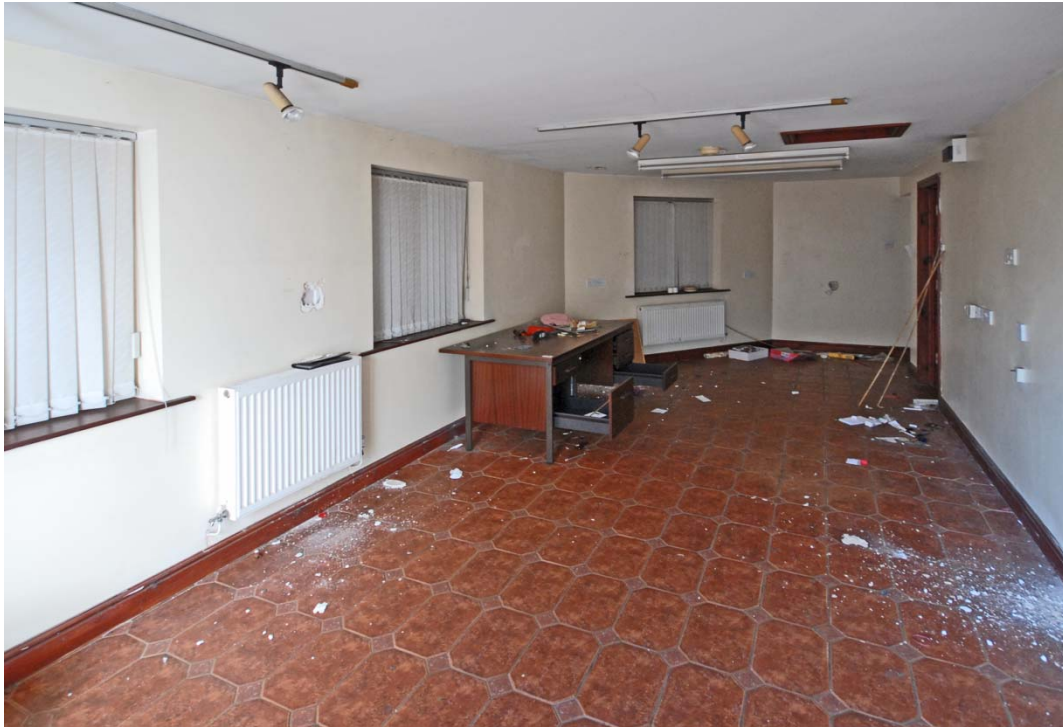
0043 Office G17, interior Fig 19
