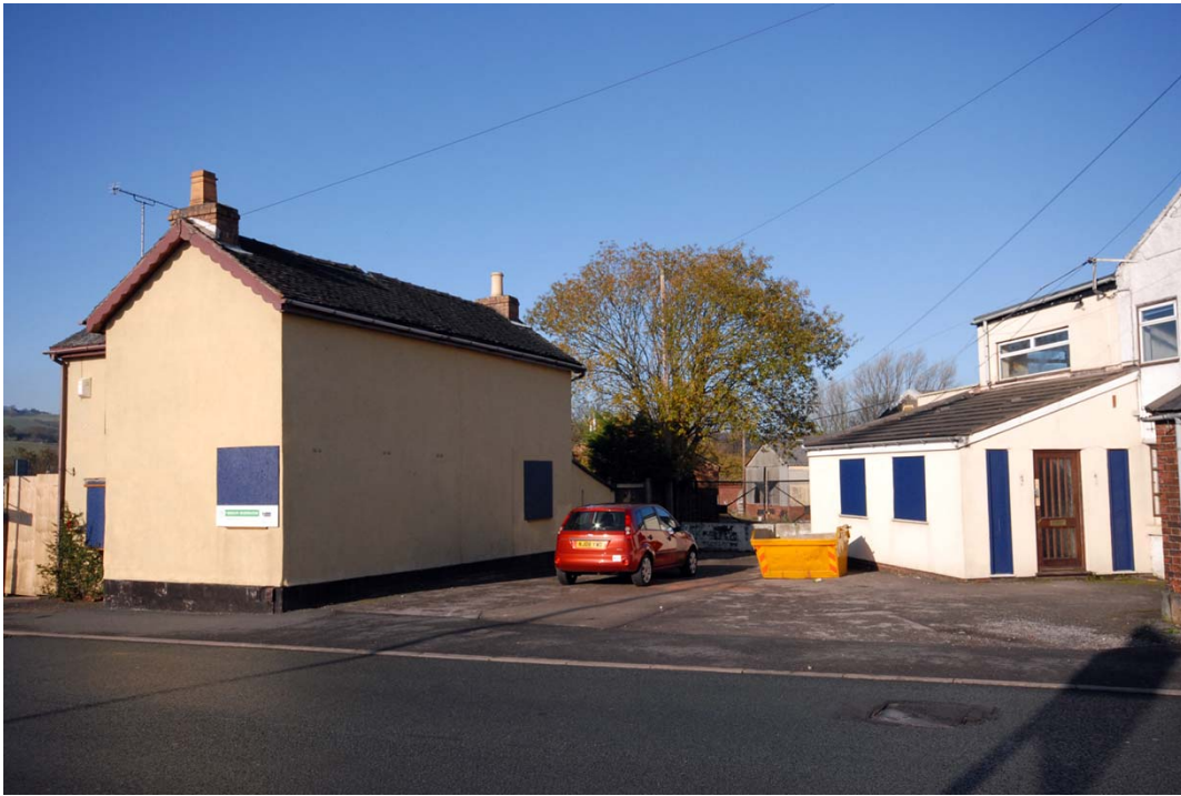
0009 Yew Tree Cottage from across Wharf Road; note distance and angle from Yew Tree House on right Fig 22
