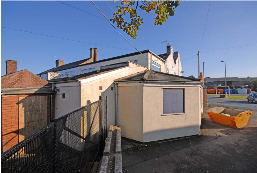
0046 Office G17 and workshop G12 from rear yard Fig 9
