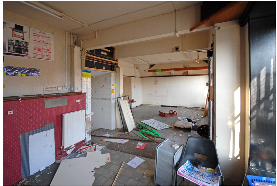
0053 The former shop interior Fig 4
