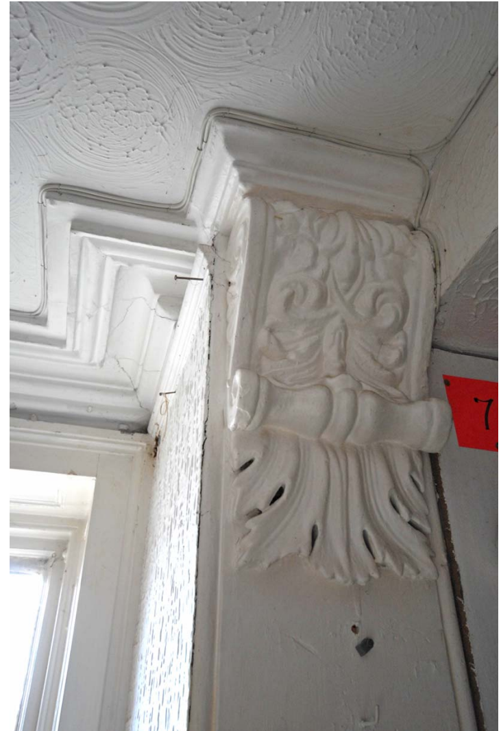
0056 Detail of plaster console bracket and cornice in G7 Fig 8
