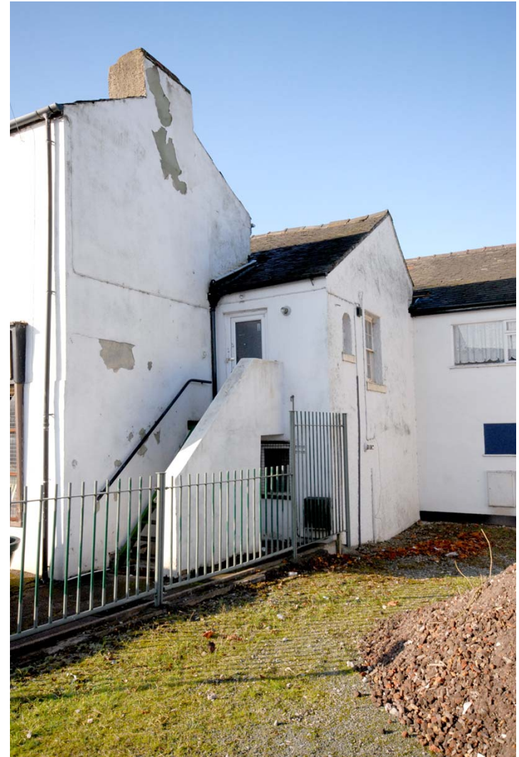
0013 Stair to upper floor flat Fig 10
