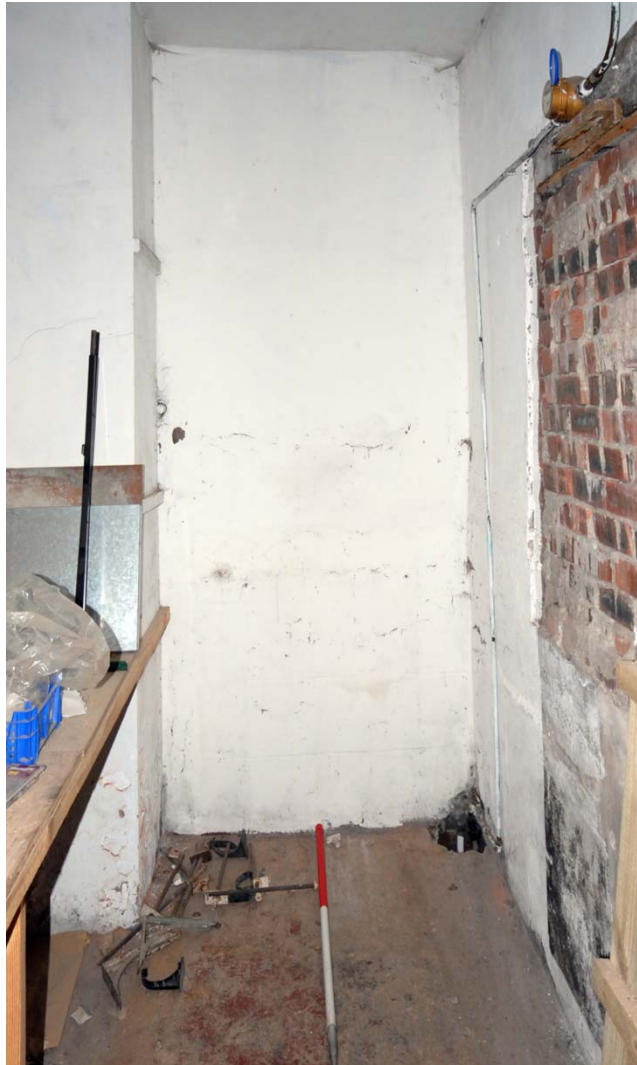
0090 Location of possible former copper in G12a, blocked window...
