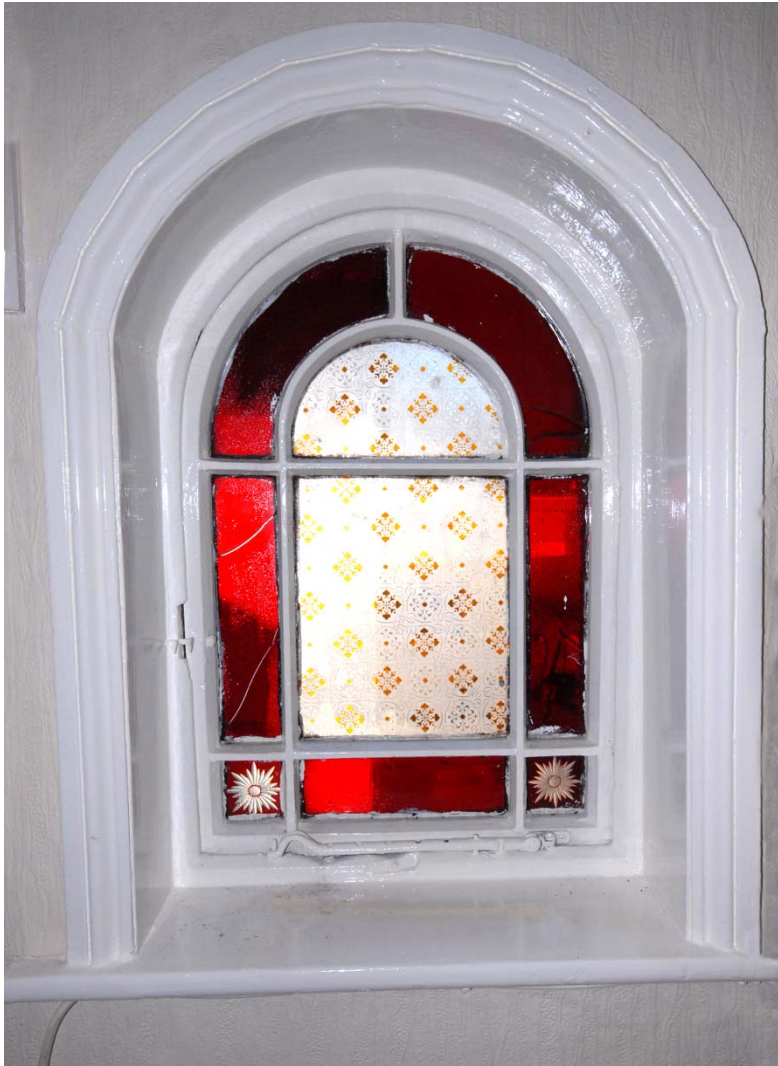
0040 Late Victorian window at top of stairs Fig 11
