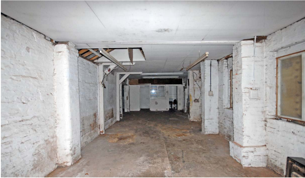
0024 Workshops G14, interior Fig 17
