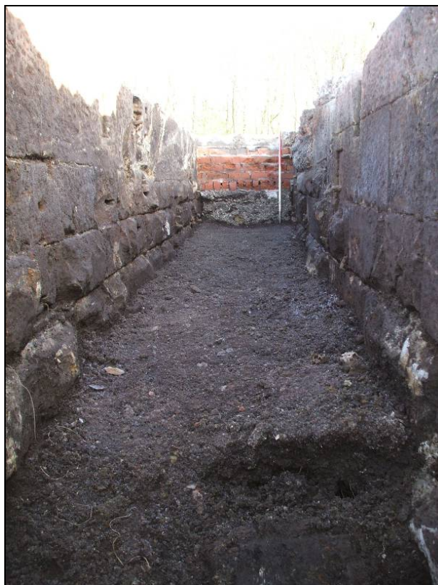
View of culvert/wheel pit, looking north Fig 8
