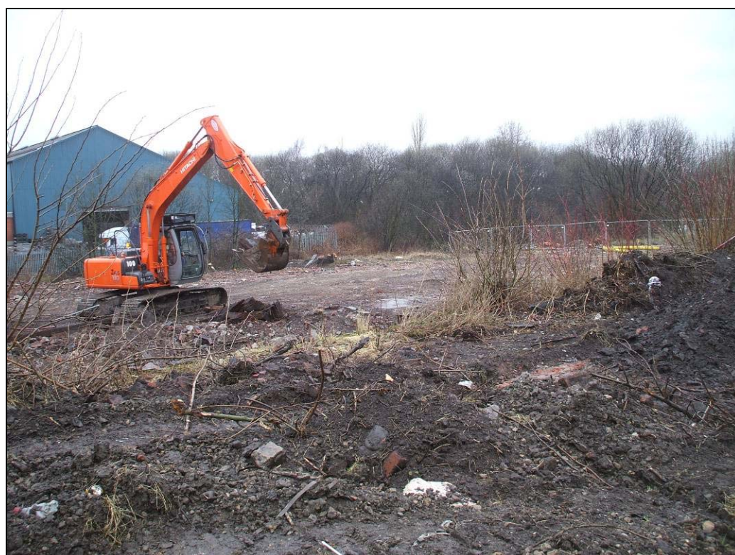
Pre-excavation view of site, looking north-west Fig 3
