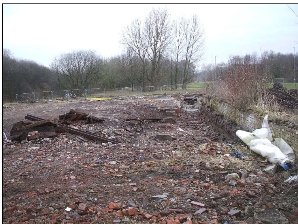
Pre-excavation ground works exposing upper level of goit, looking north Fig 11
