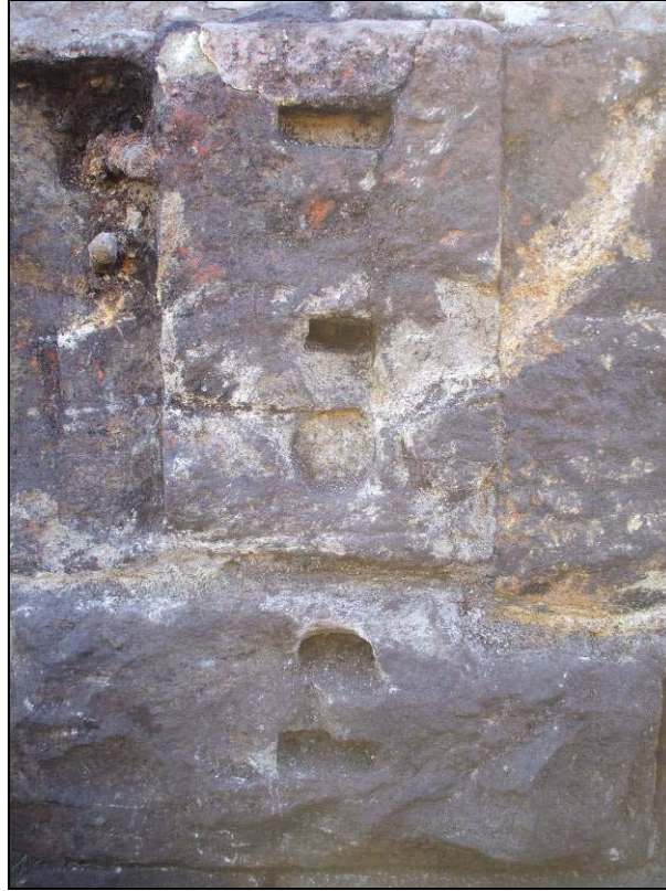
Example of fittings located in wall faces within stone-lined trough Fig 27
