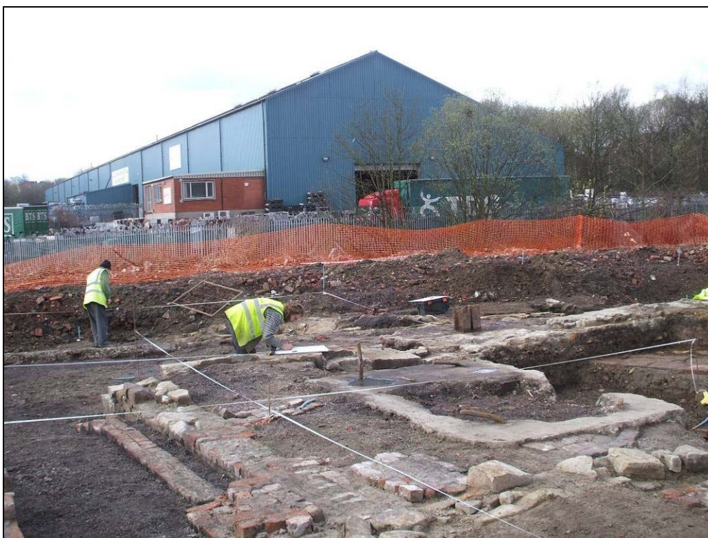
Concrete machine base [3041] (centre right) within New Machine Room, looking north-west Fig 29
