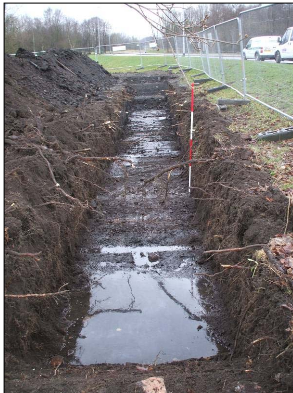
Trial excavation exposing upper level of reservoir silts, looking north Fig 14
