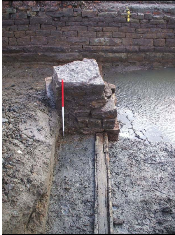
Late 19th-/early 20th-century bleach works extension across the goit, showing timber beam [3011] and pier [3012], looking east Fig 32
