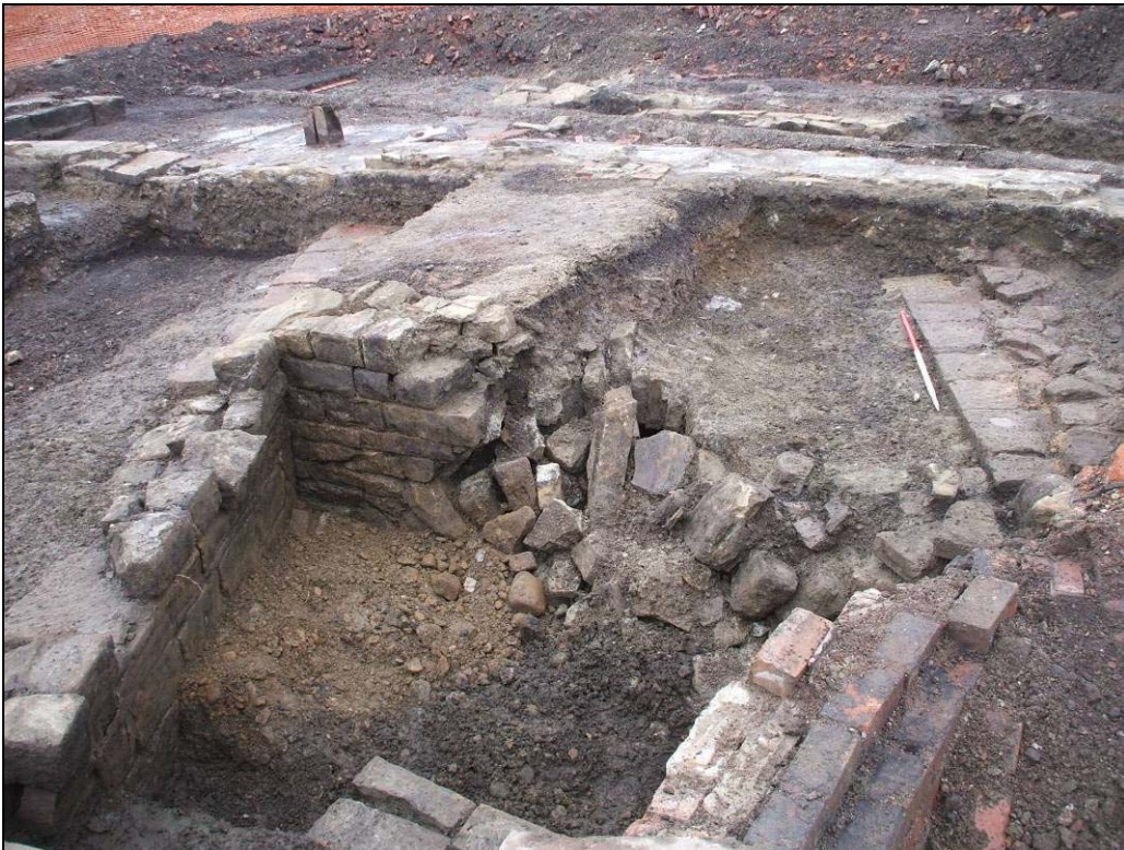
Collapsed leat vault opening [3024], looking south-west Fig 30
