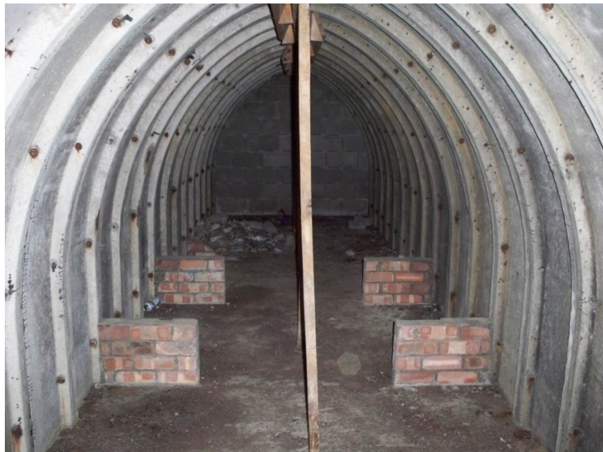
The interior of a underground structure in Area 1, looking north-east Fig 10
