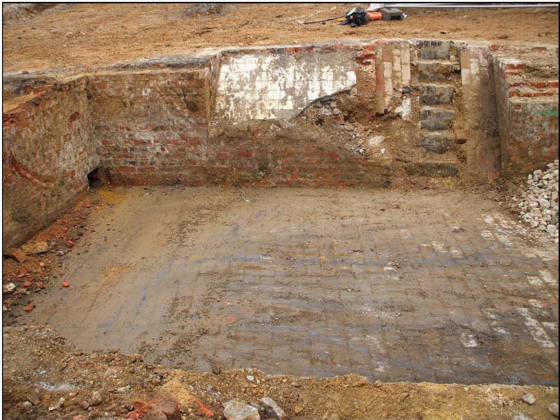
Cellar for Payne's Cake Shop, Plot 3, late 19th-century, looking east Fig 25
