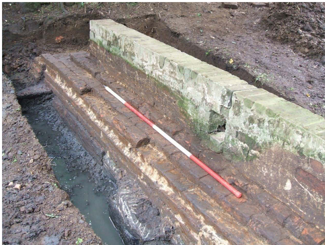
Trench 3, detail of weir foundations [305] looking south-west
