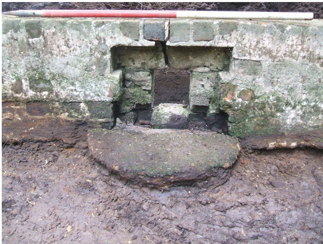
Trench 3, opening in wall [304] and concrete pad, looking north
