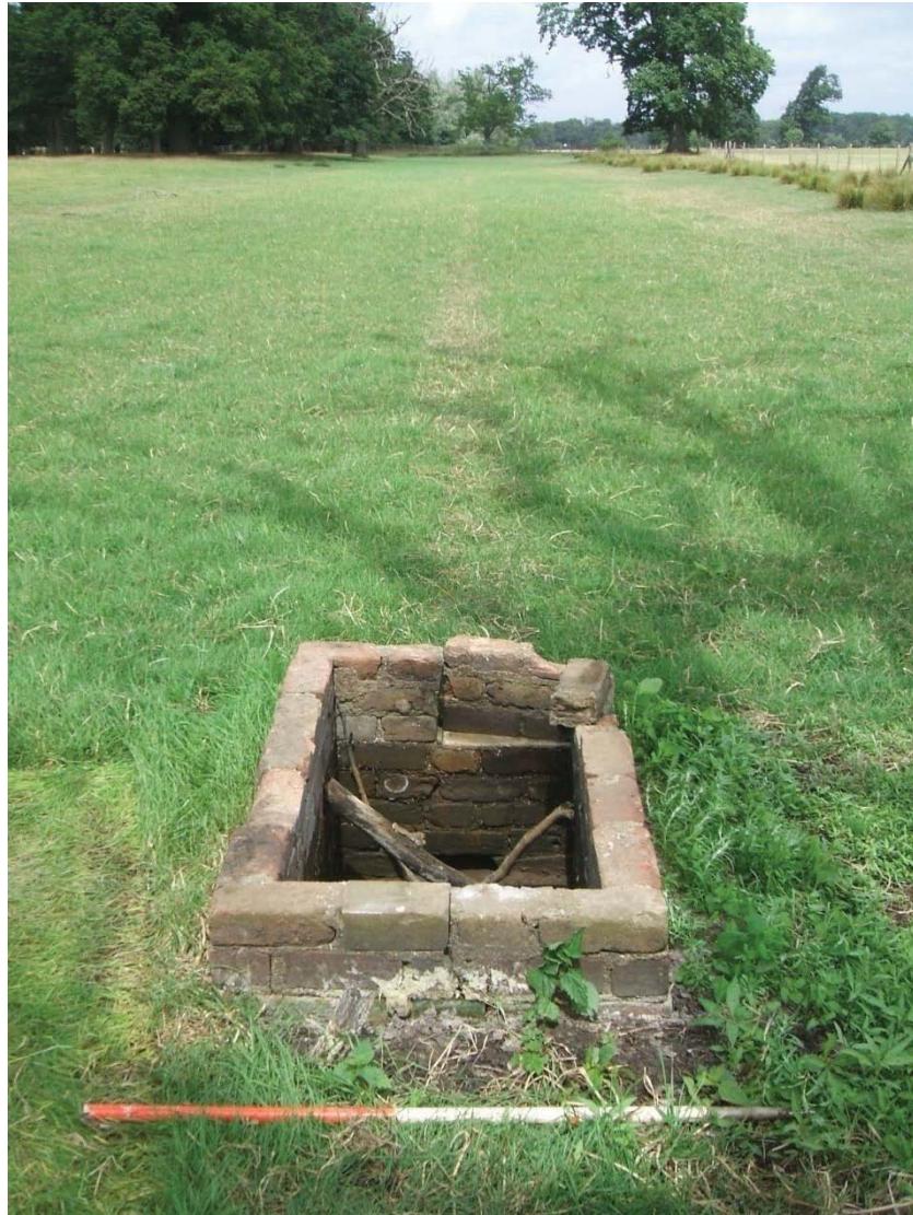
Brick inspection hatch and parchmark looking north-east Fig 23
