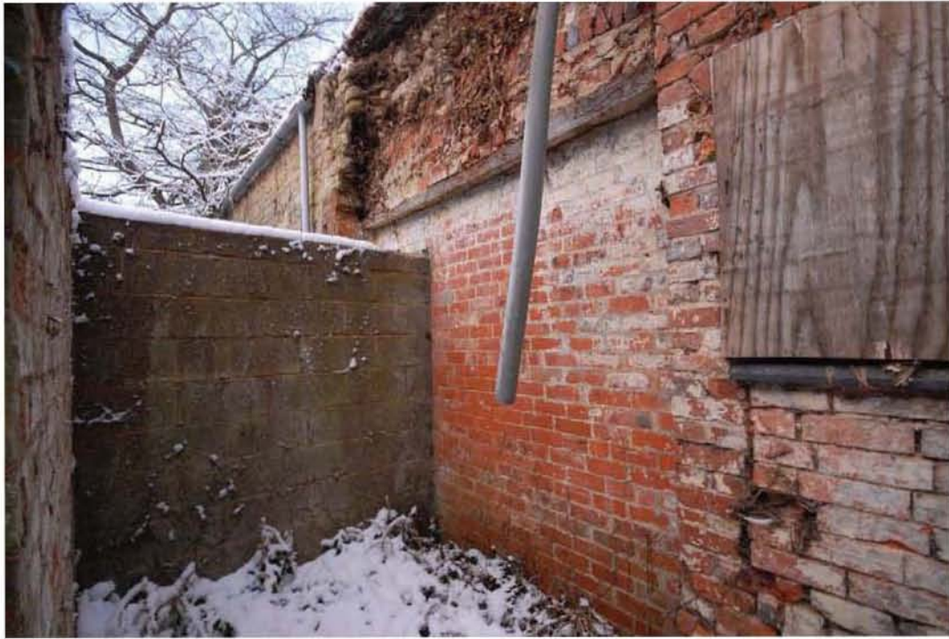
0098 Blocked-in former carriage entrance Fig 21
