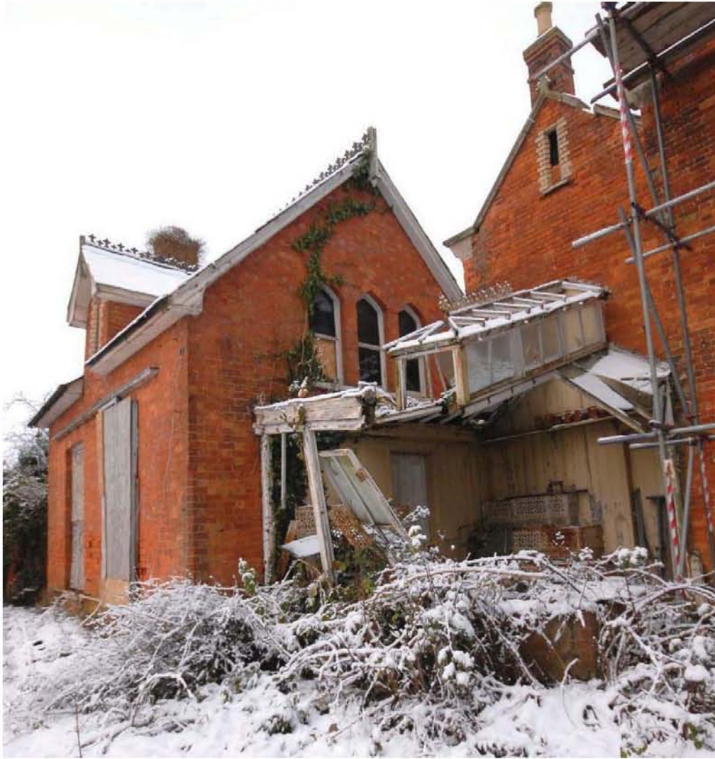
0080 Exterior view of chapel G17 Fig 57
