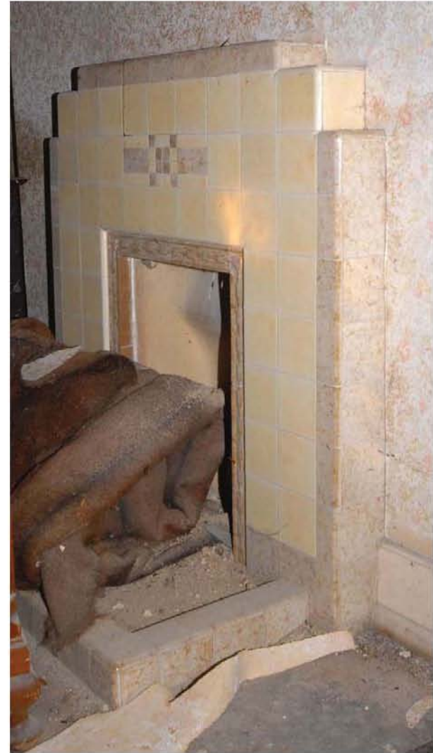
0060 Fireplace in bedroom F5 Fig 40
