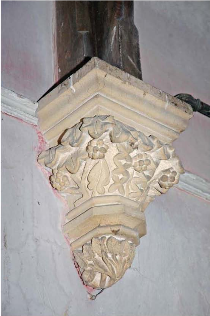
2979 Corbel supporting roof truss on wall-post, G17 Fig 59
