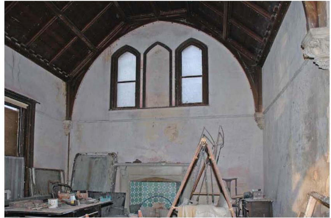
2966 Interior of chapel G17 Fig 58
