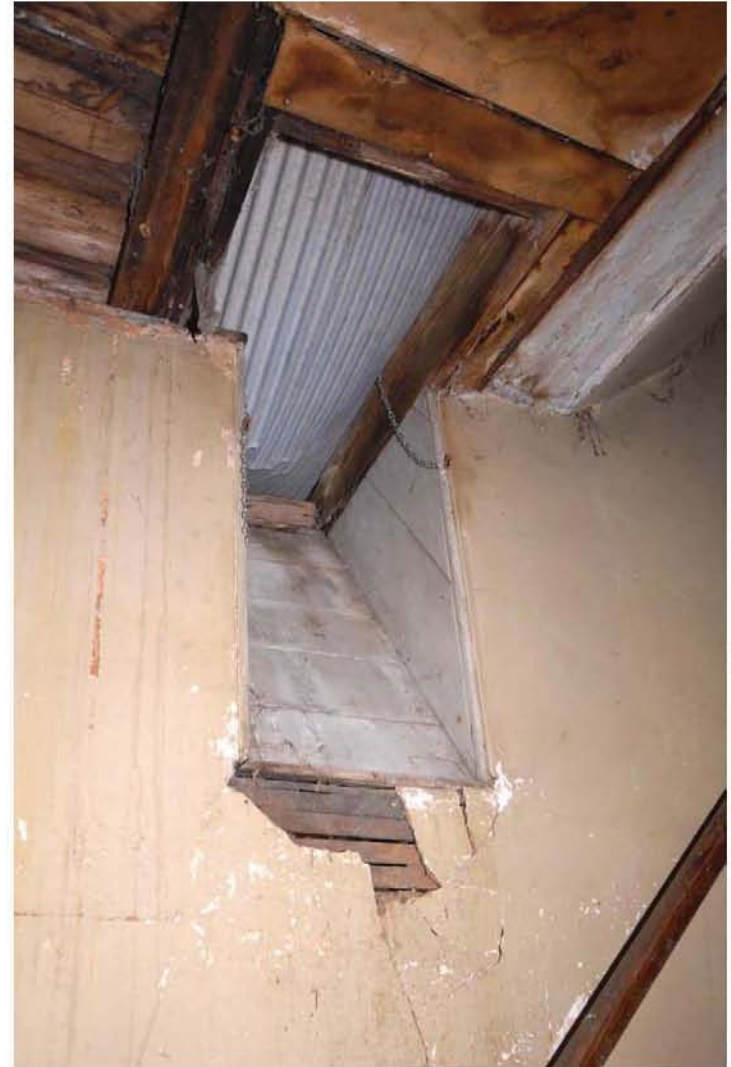
0064 High window lighting second floor stairs Fig 46
