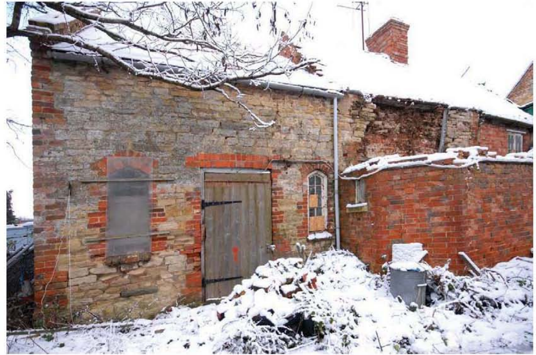
0091 Rear of stable and coach house, later Ousebank Cottage Fig 20
