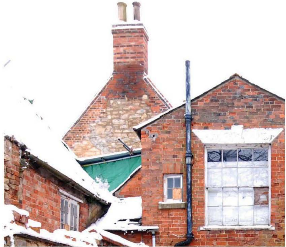
0089 Altered gable on main house (zoom in) Fig 16
