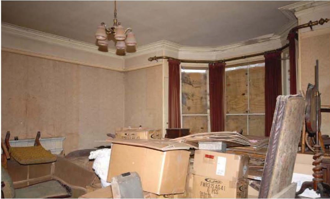
0037 View across G7 towards bay window Fig 33
