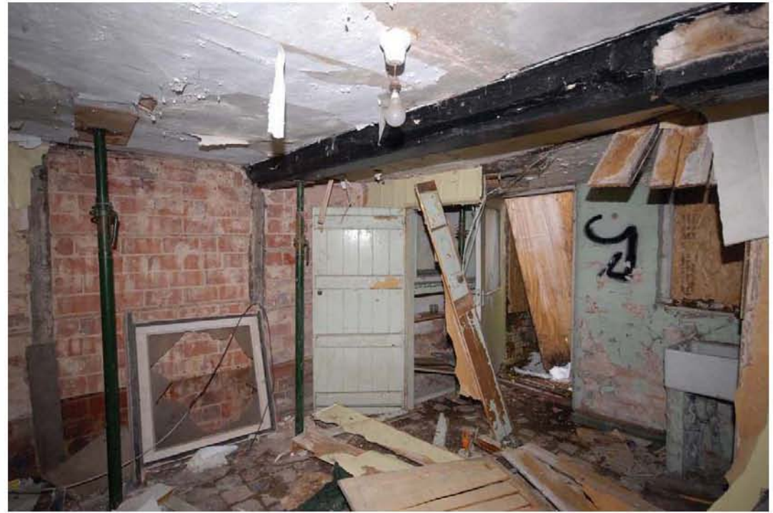
0100 Rooms G8-G9, looking frontage to rear Fig 48
