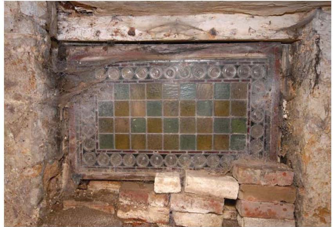
0029 Curiosity window in cellar Fig 10
