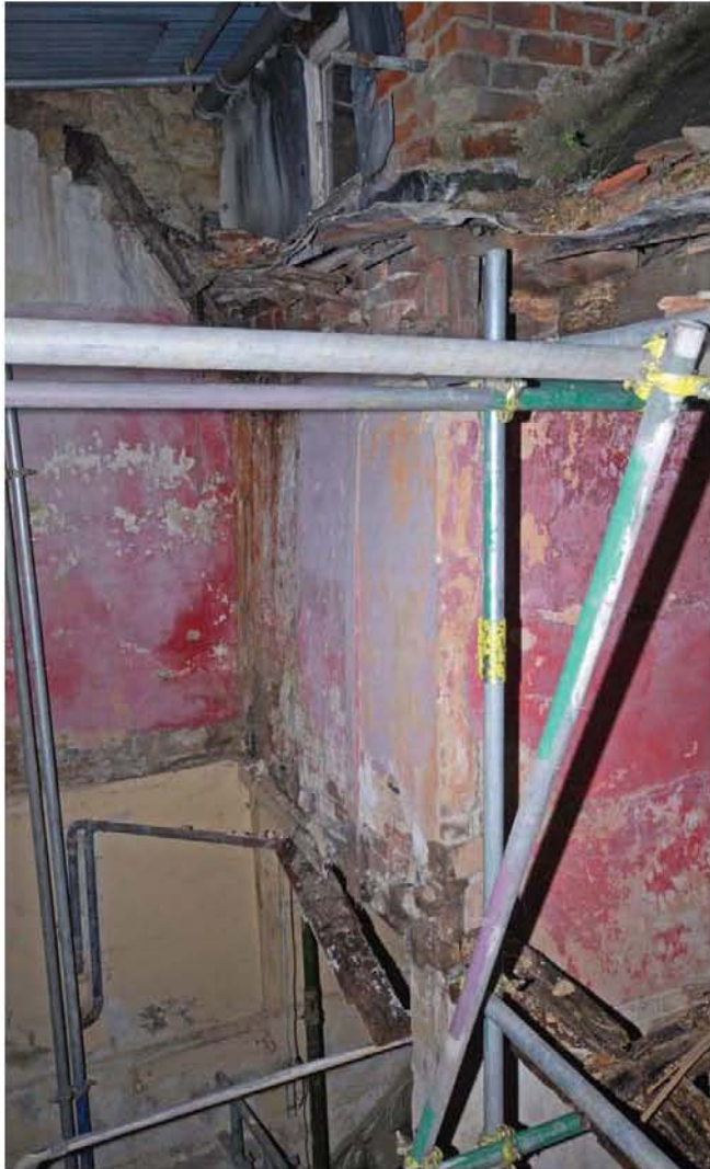
0105 Stair-tower viewed across F13 Fig47
