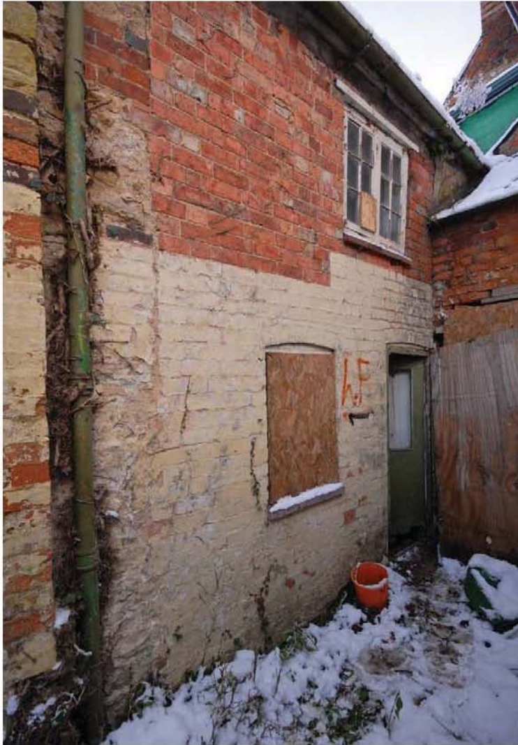
0097 Butt joint in brickwork of converted carriage house (left) and Ousebank...
