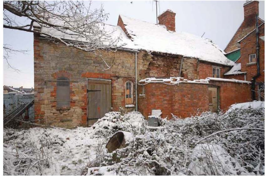
0088 Narrow yard-space G12 behind Ousebank Cottage Fig 64
