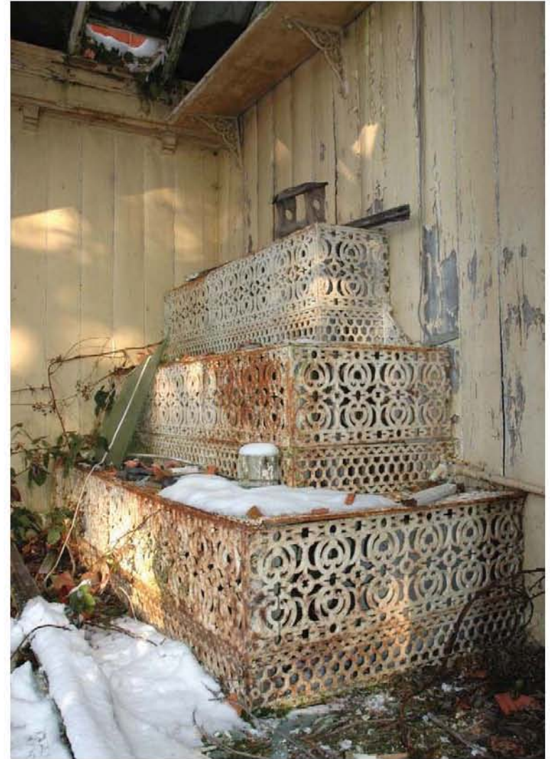
2986 Cast iron heating grates reused in conservatory G18 Fig 62
