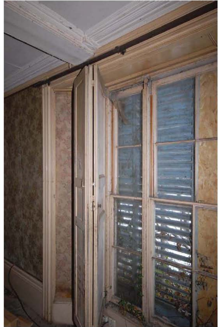
0036 Ceiling detail in G6 Fig 32
