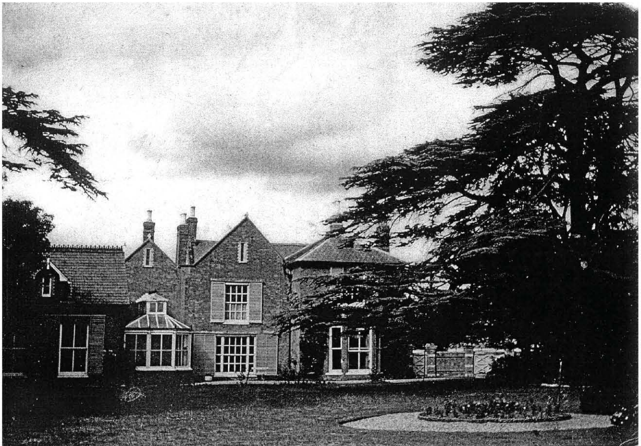
1950s view of rear of property (photo provided by Colin Clayson) Fig 5
