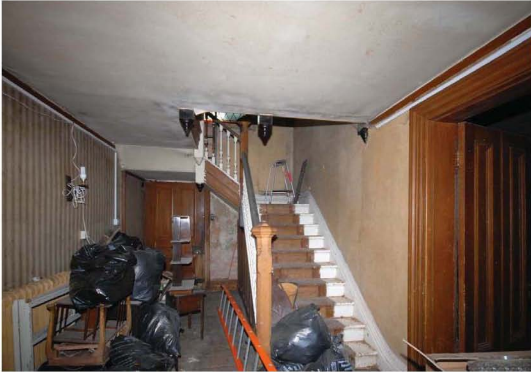
0010 Hallway and stairs G4 Fig 23
