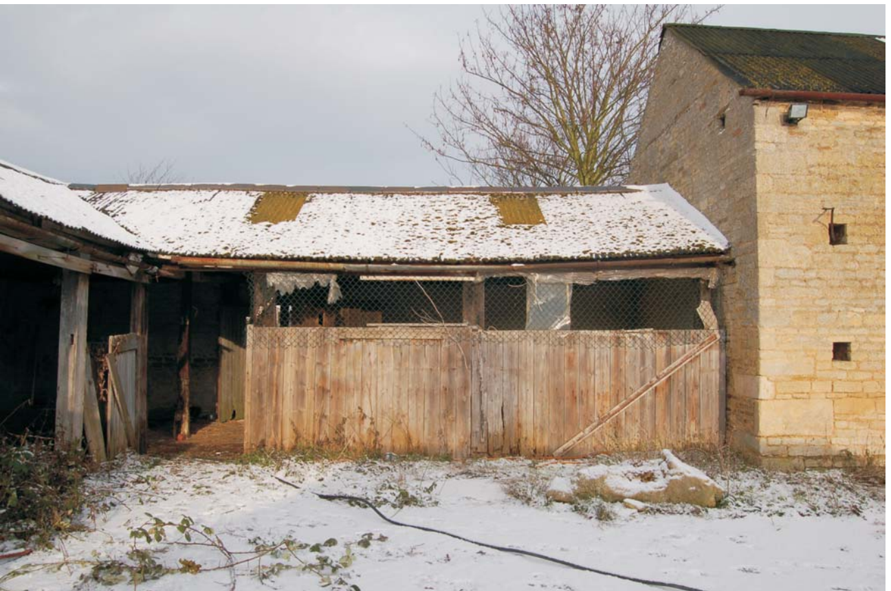
Stalls, looking north Fig 22
