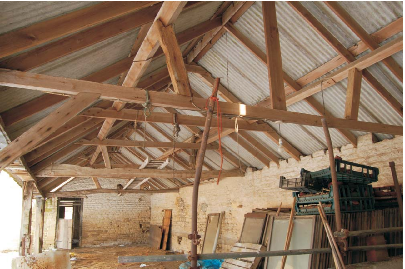
Roof of stock hovel, looking north Fig 21
