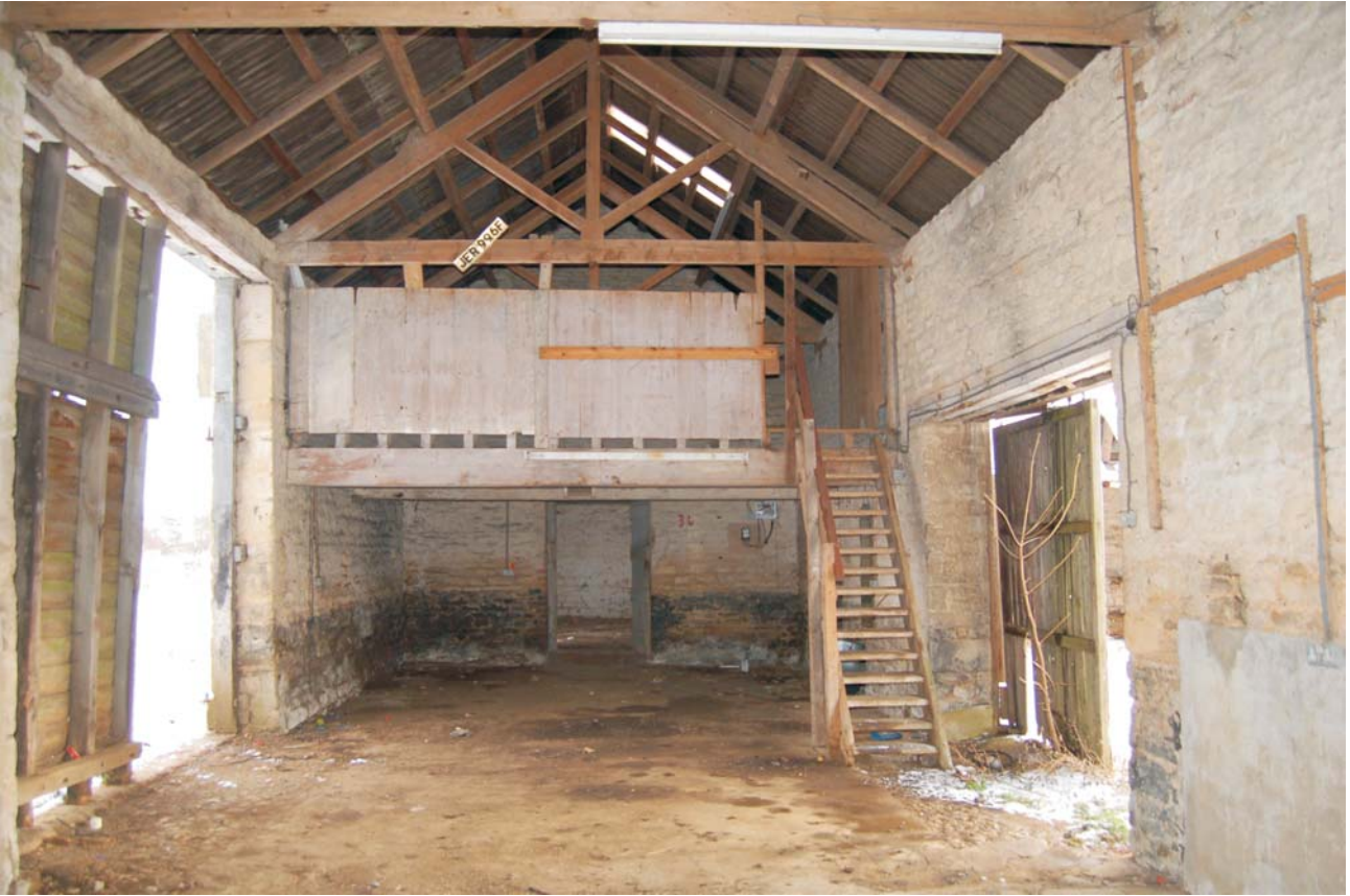
Roof of store barn, looking east Fig 15
