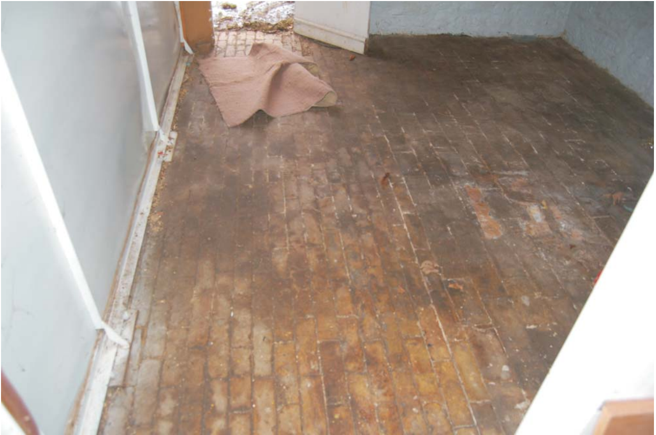
Floor of detached barn Fig 30
