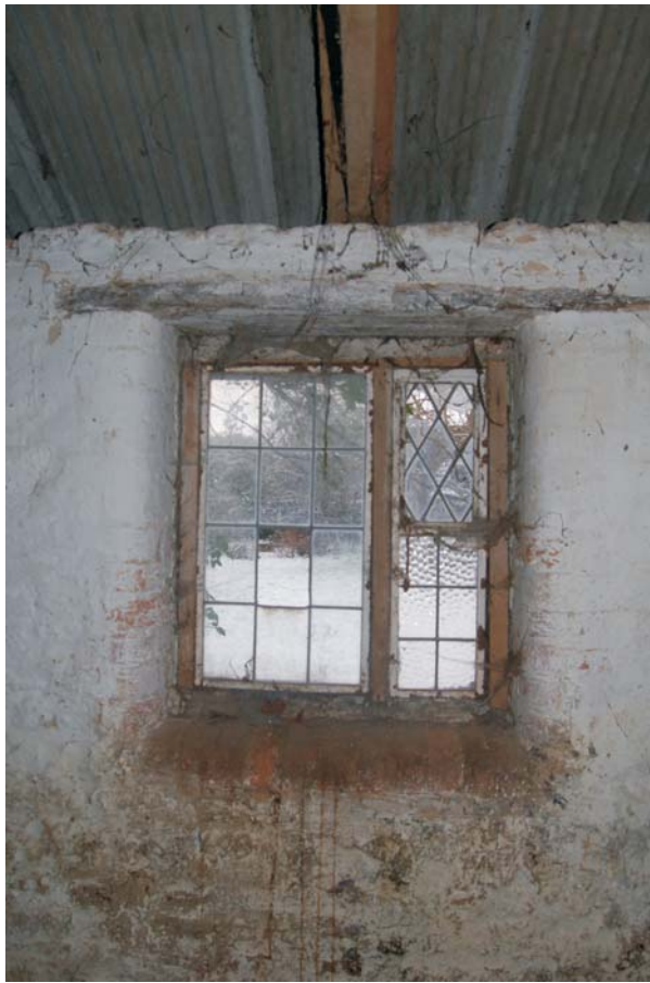
Window in west wall of Stable 2 Fig 25
