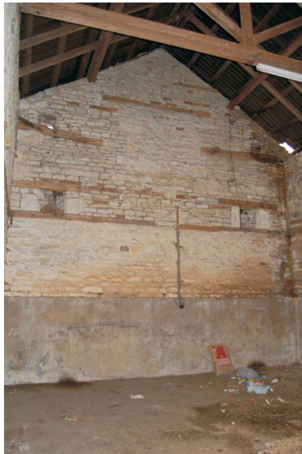
West gable wall of store barn Fig 14
