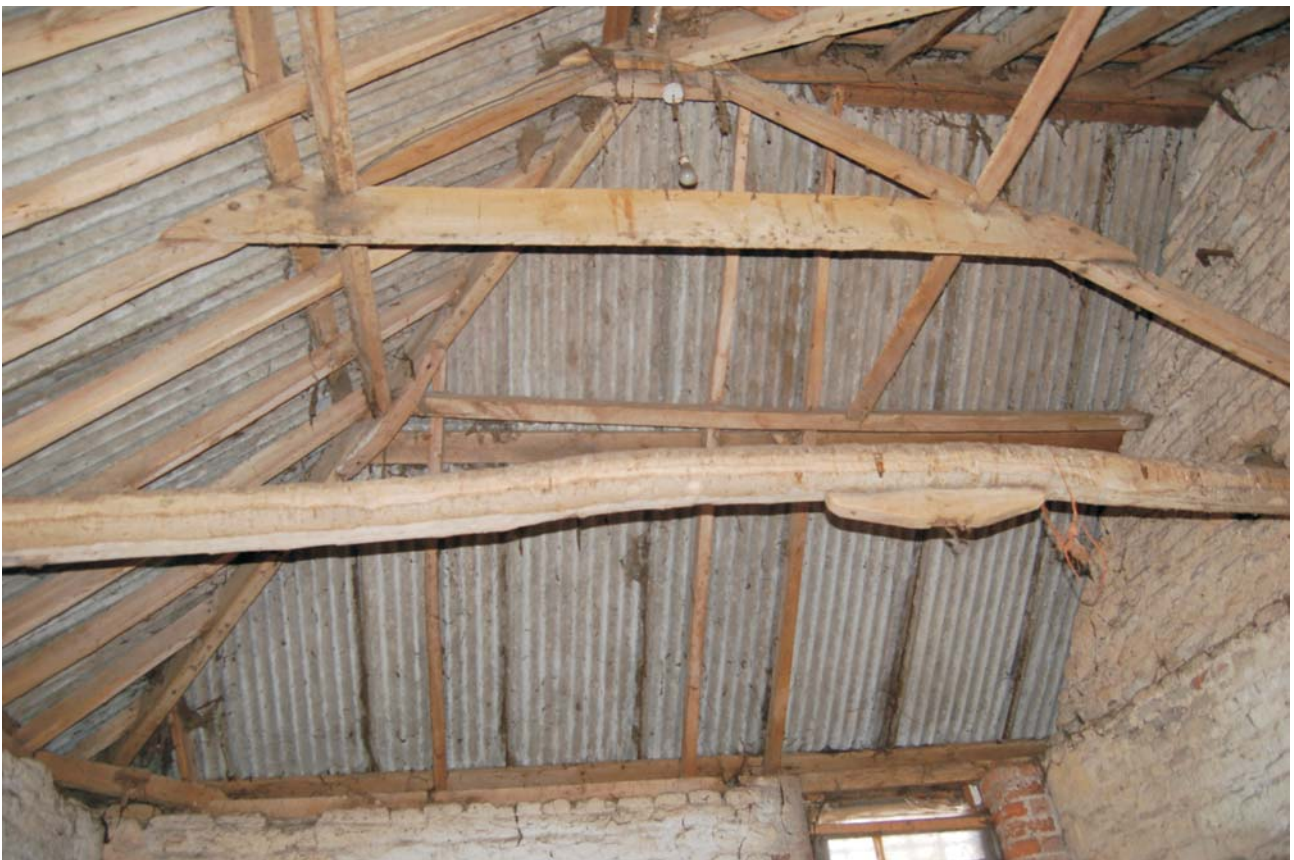
Roof of loose box, looking east Fig 18
