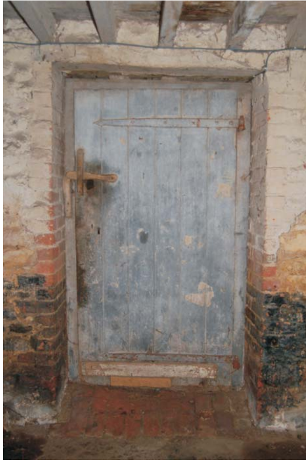
Door in east wall of store barn Fig 13
