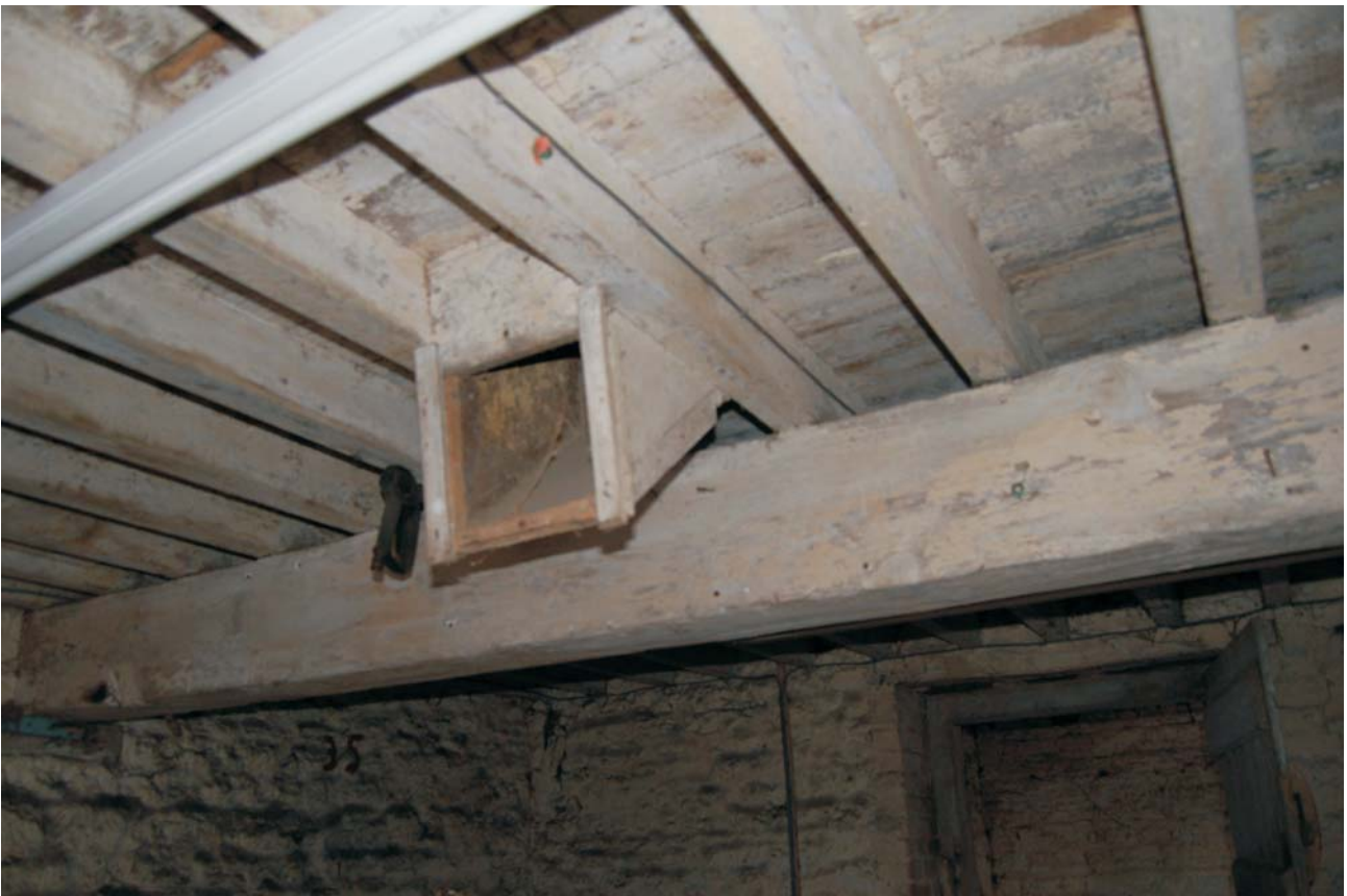
Chute beneath hayloft Fig 16
