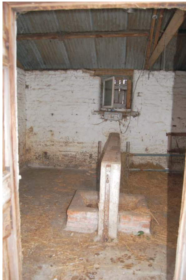
Breeze block wall and troughs in Stable 1 Fig 24
