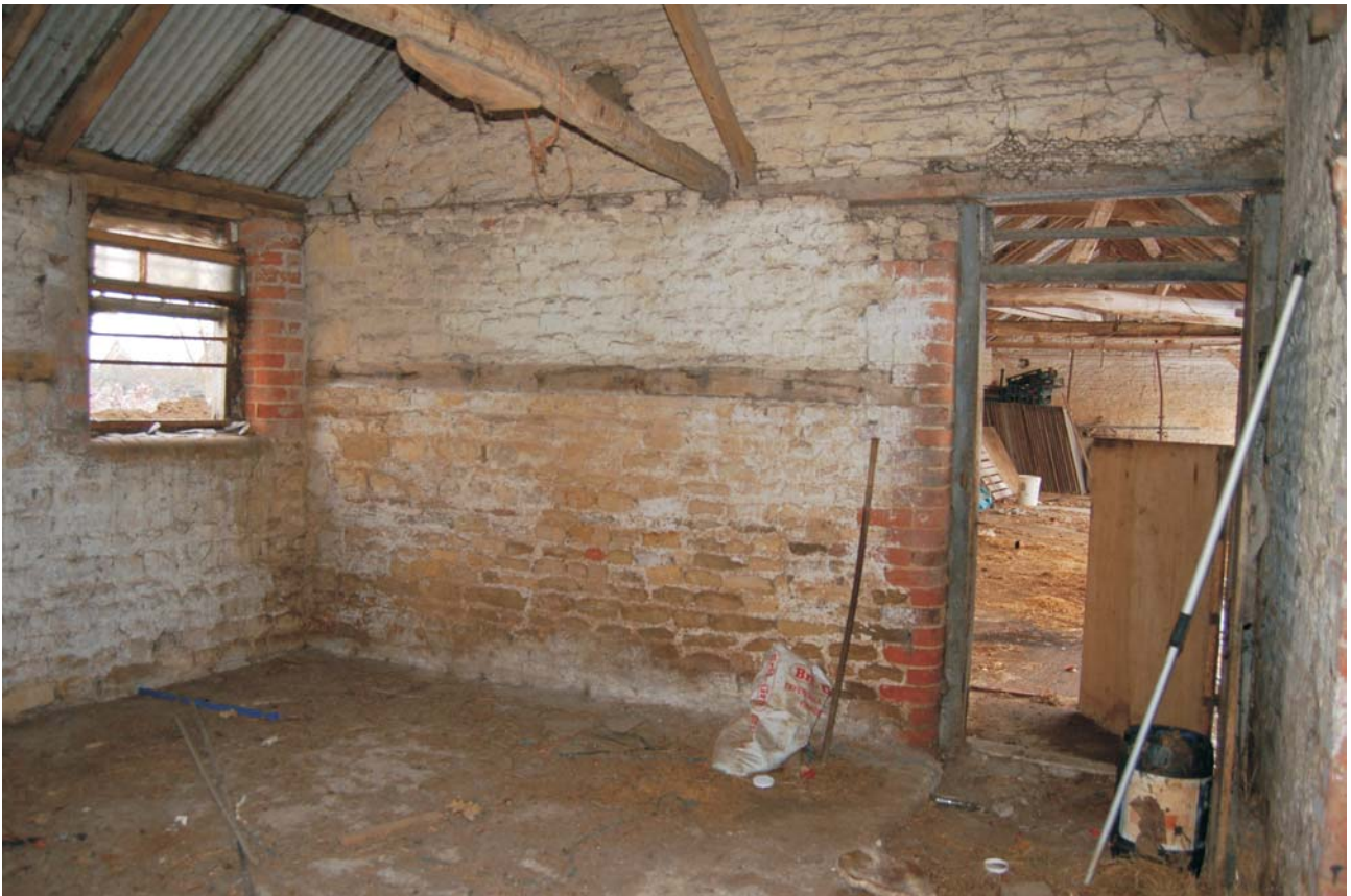
Loose box, looking south-east Fig 17
