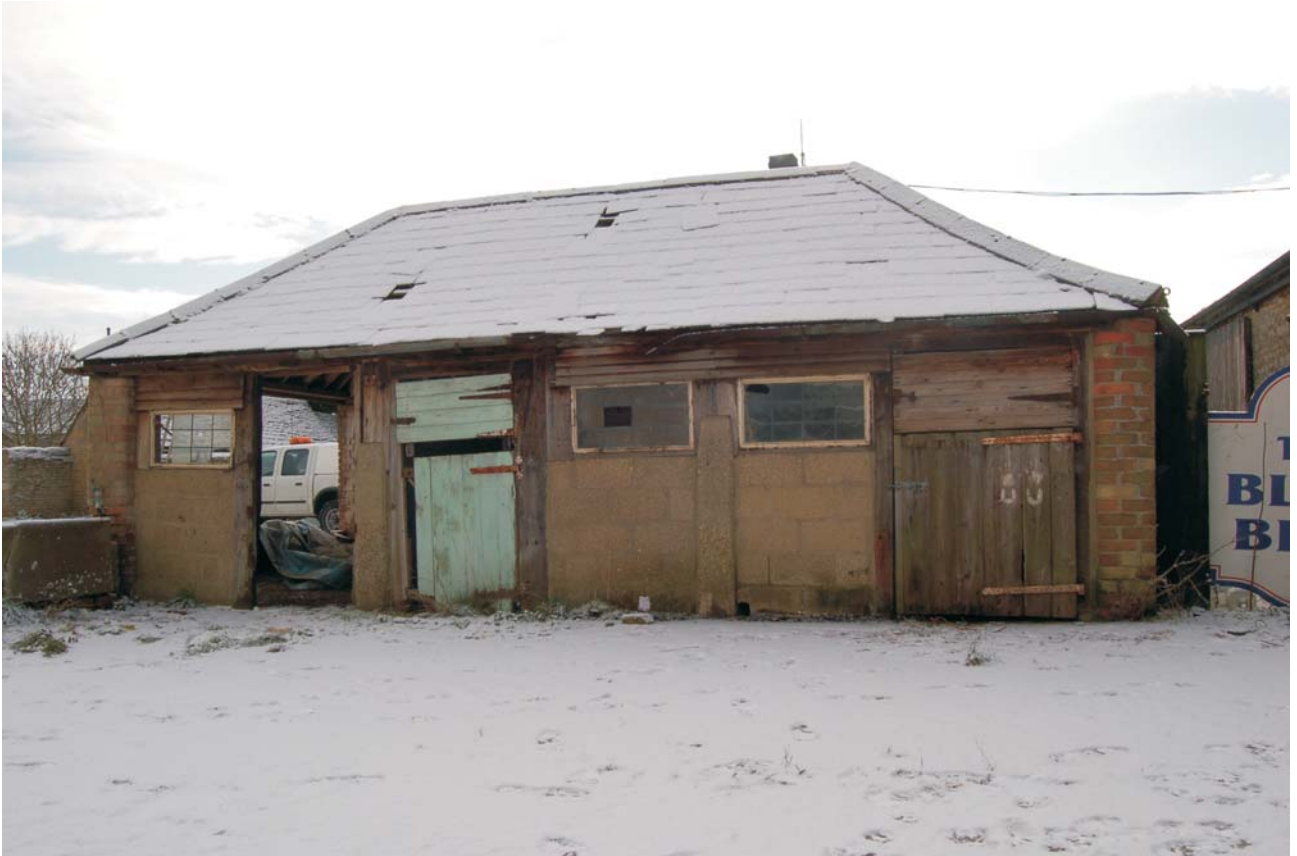
Brick building, looking south Fig 26
