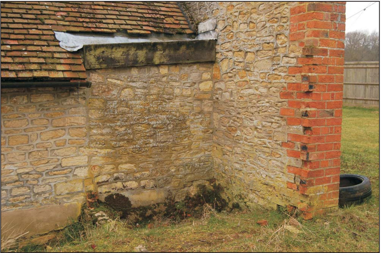
Location of possible former outside WC Fig 21
