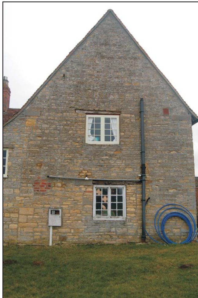
Rear gable of the service wing; reduced window width at ground floor Fig 12
