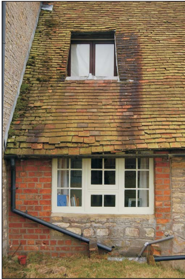
Former yard-space, enclosed and blocked to create G9 Fig 19
