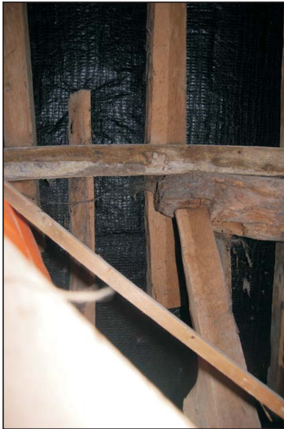
Propped south purlin of service wing roof Fig 17
