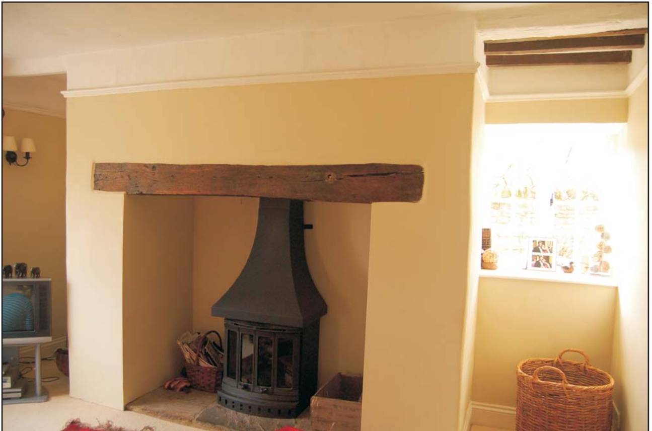
The rebuilt inglenook fireplace in G2 Fig 6
