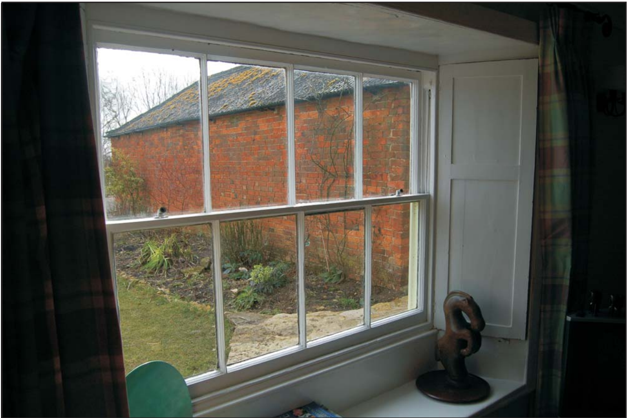
The early sash window and shutter/boxes in G2 Fig 7
