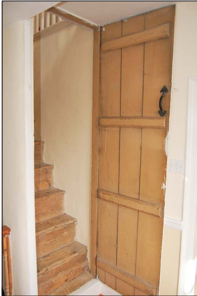
View of stairs and door to second floor attic Fig 15
