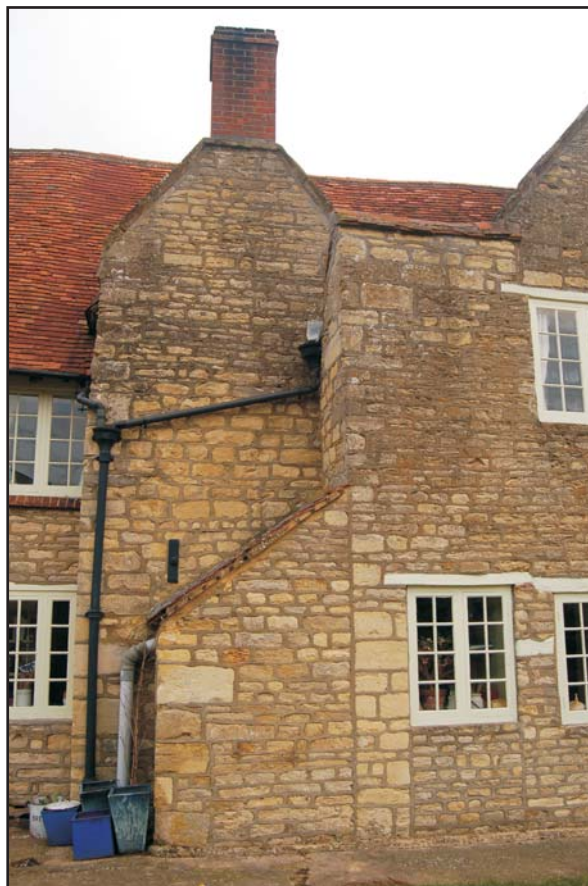
Agglomeration of stonework at the Fig 10 junction of the wings
