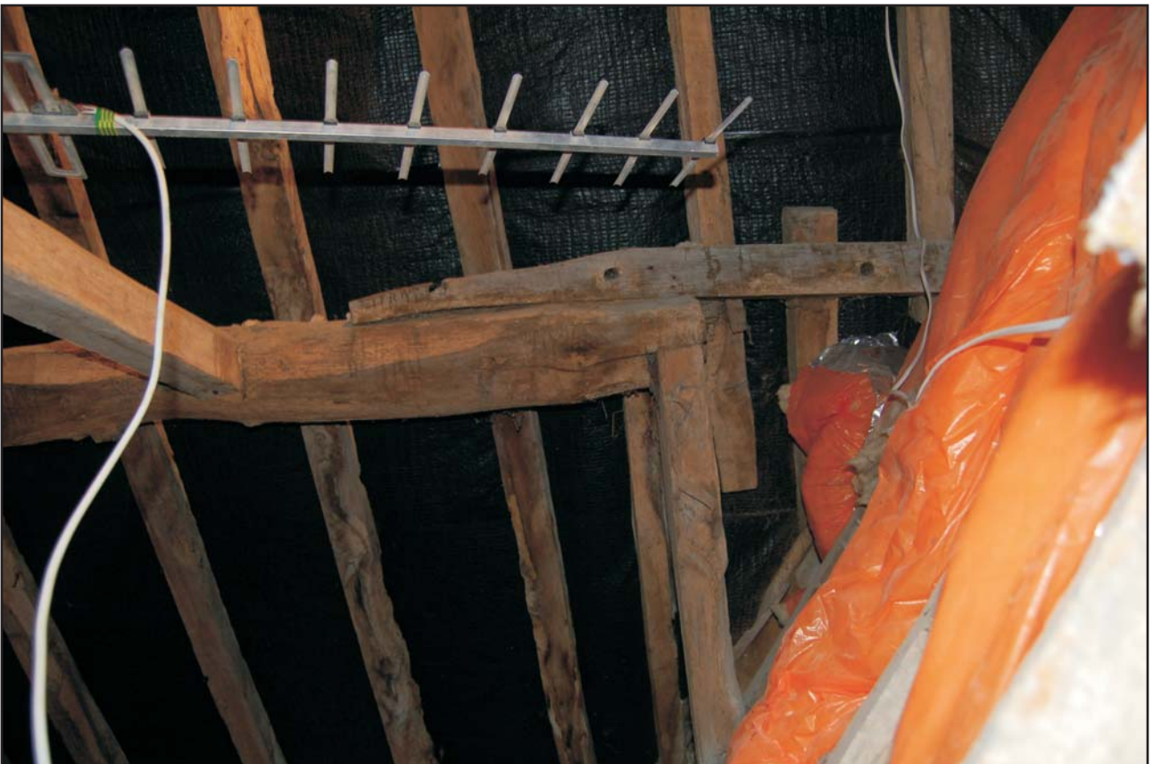
Propped north purlin of service wing roof Fig 18
