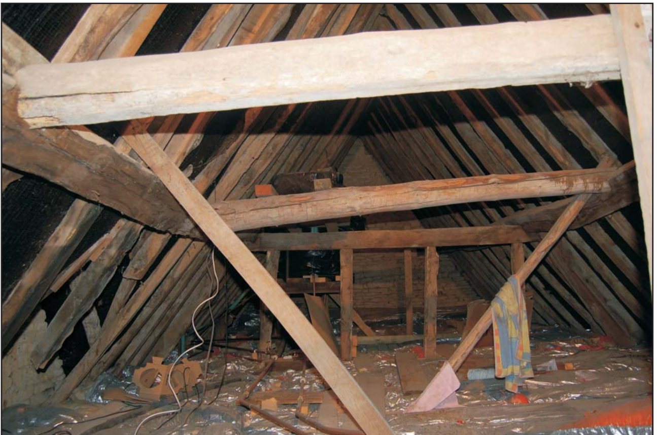
View along service wing roof Fig 16
