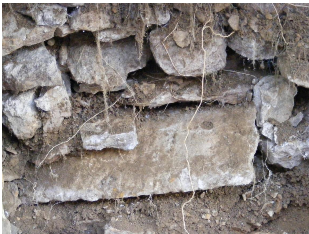
Former coping stone built into retaining wall Fig 4
