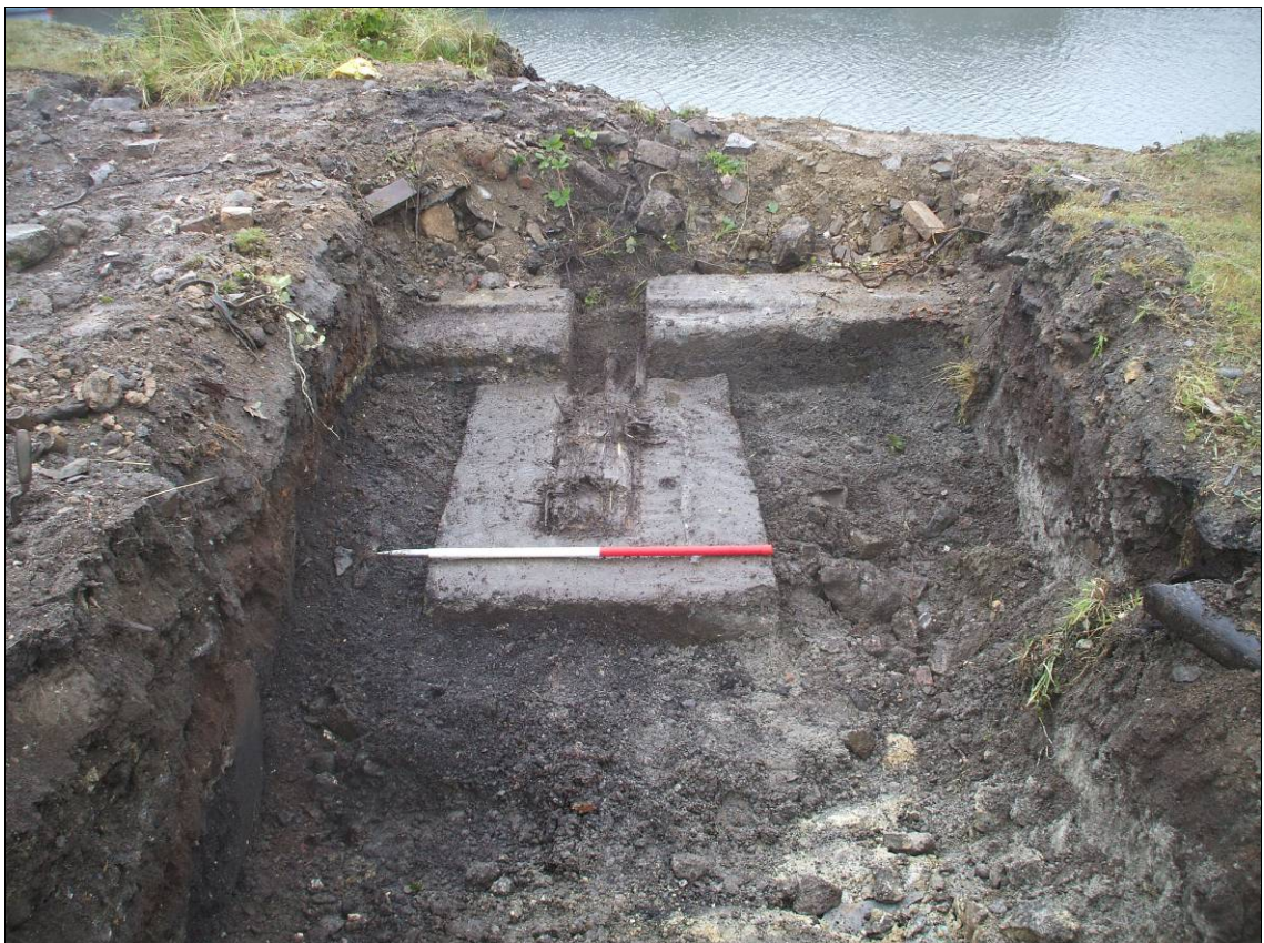
Timber beam [1010] tied into concrete base [1009] and passing through quay wall, Trench 1, looking west Fig 23
