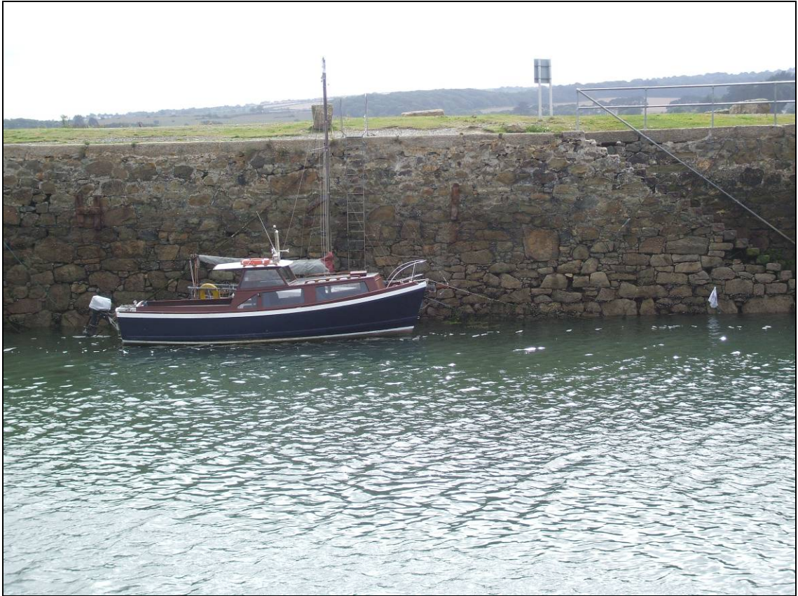
Granite construction of Carnsew Quay, looking west
