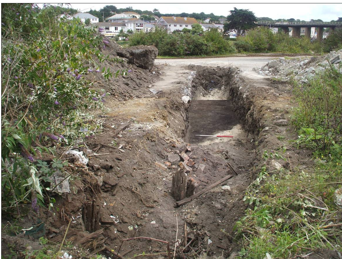
Slipway timbers [5013] (foreground) and compacted iron-slag slip (5007), Trench 5, looking south-east Fig 29
