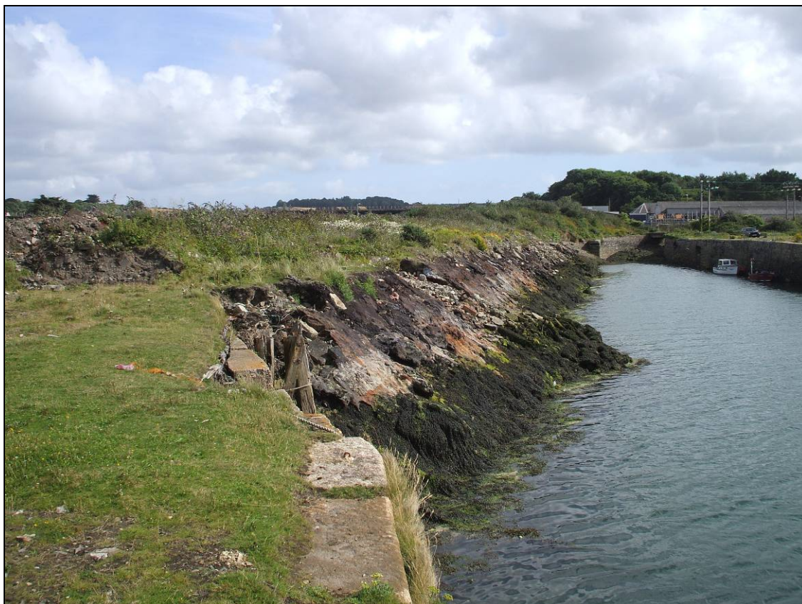
A view of the material in-filling South Quay and Carnsew Channel, looking south Fig 3
