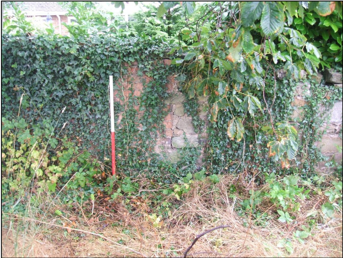
Change of brick to stone in northern wall, looking north Fig 8
