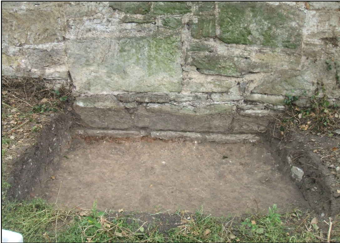
The wall foundations exposed in Test Pit 3, looking north Fig 6
