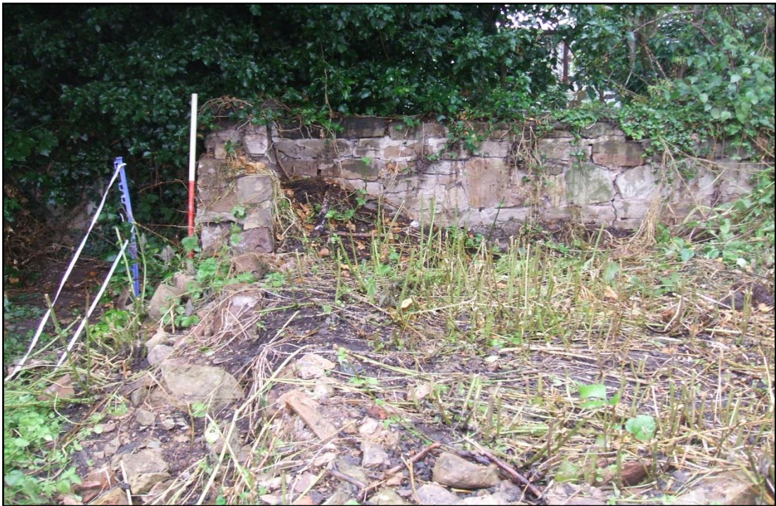
Corner of central and western boundary wall, looking west Fig 9
