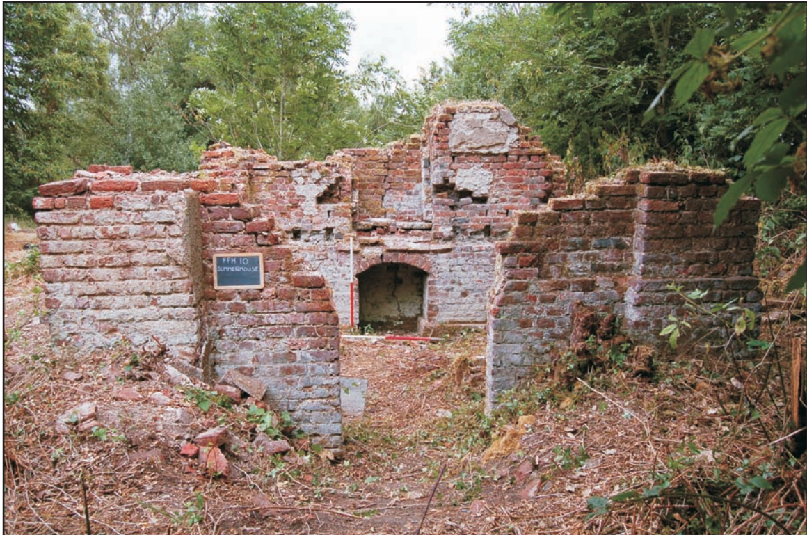
South external elevation showing door to basement Fig 8
