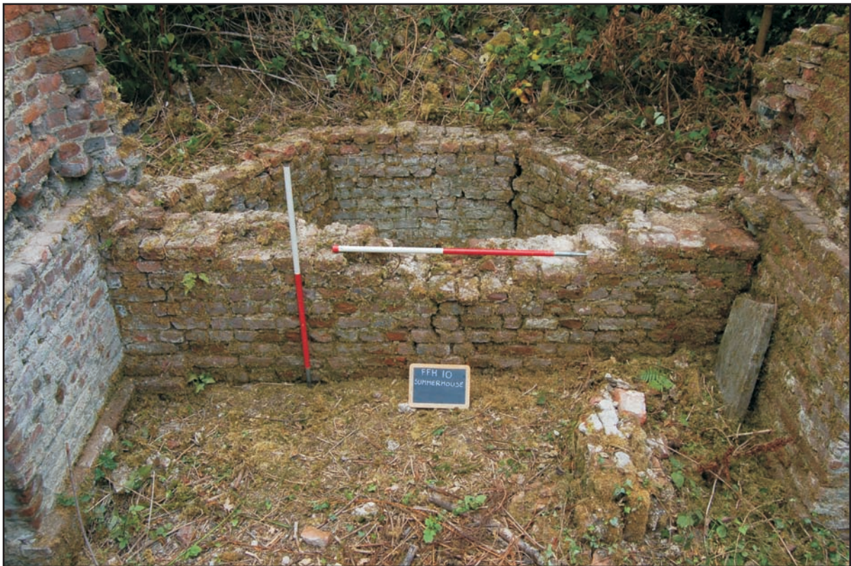
East internal elevation looking into canted bay Fig 12
