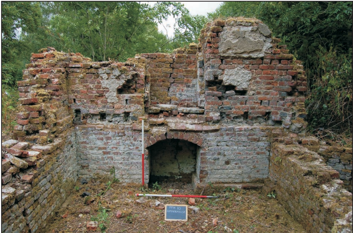
North internal elevation showing fireplace Fig 11
