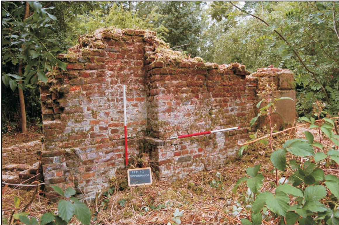
North external elevation with chimney stack Fig 6
