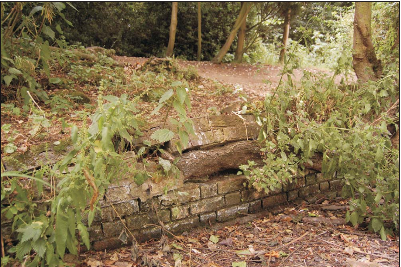
Upper Lake, London stock brick on western edge of lake showing root penetration, looking west
