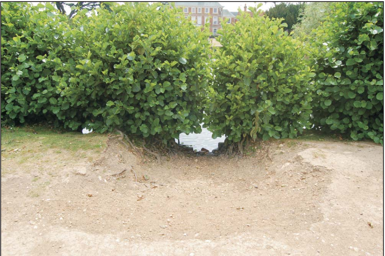
Upper Lake, eroded soil behind lost edging on north side of the lake, looking south
