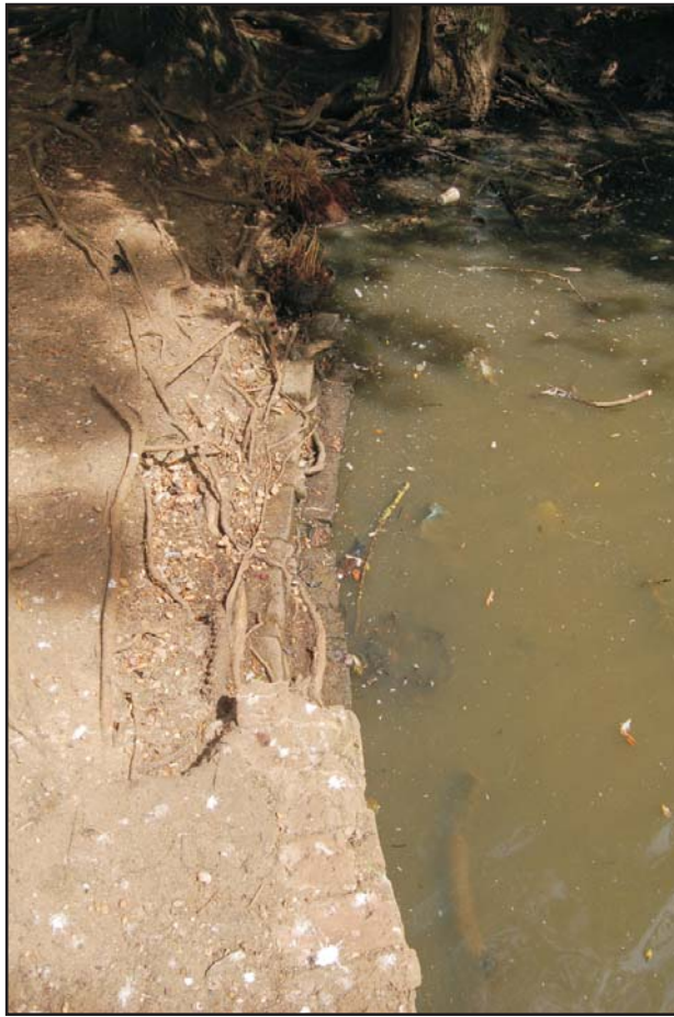
Upper Lake, north-eastern edge showing loss of stock brick edging Fig 34
