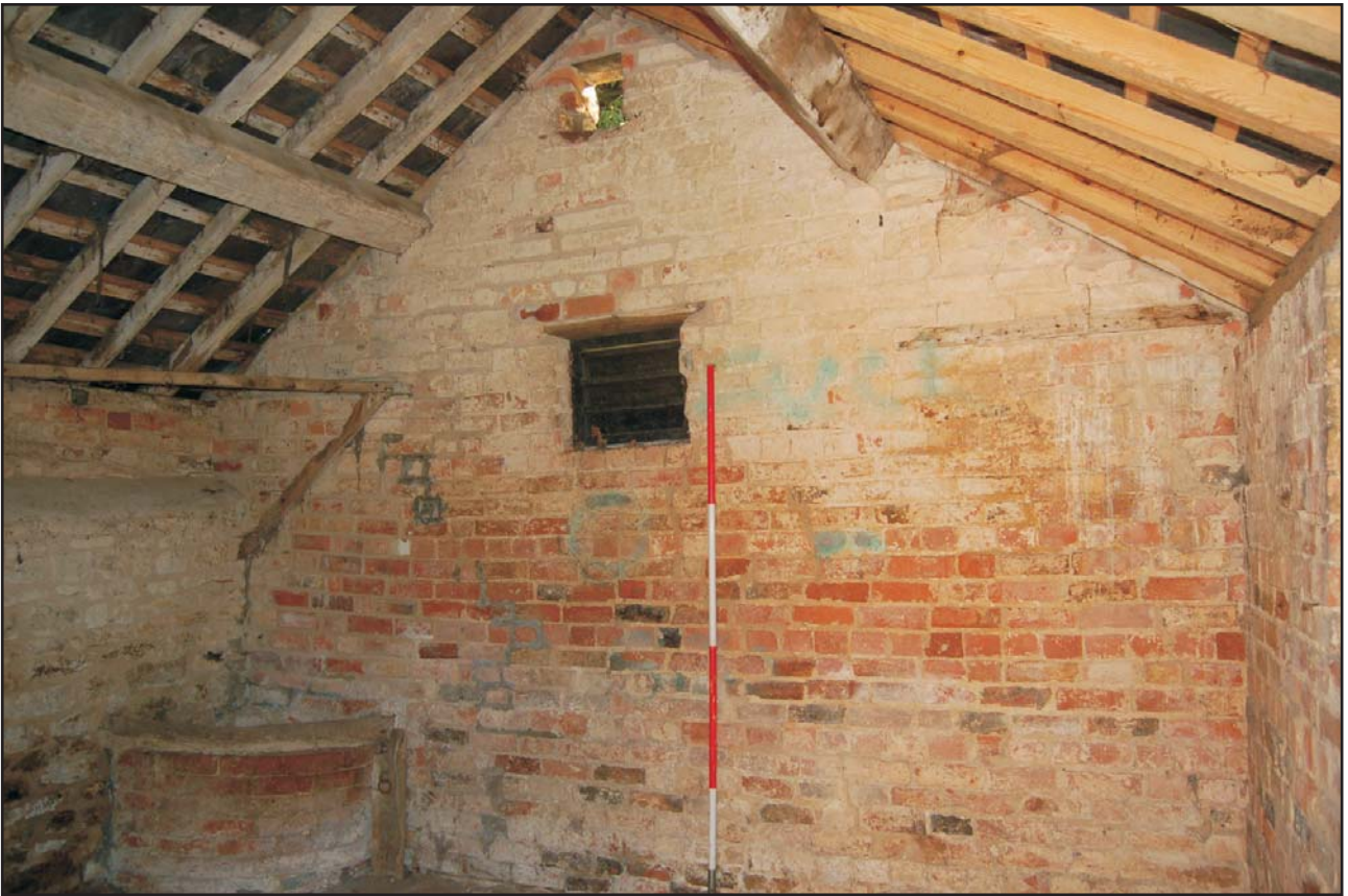
The south internal wall of the southern room, looking south Plate 9
