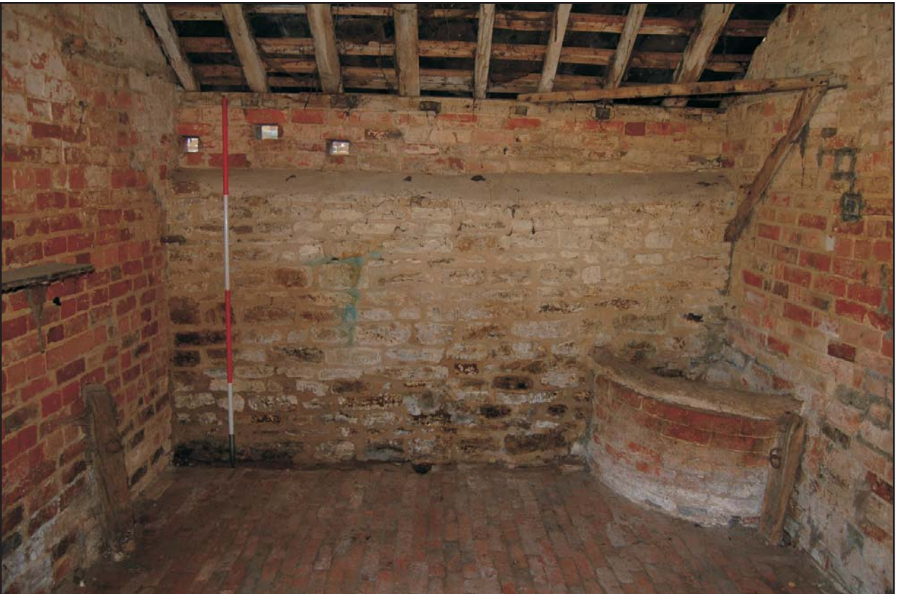
The east internal wall of the southern room, looking east Plate 8
