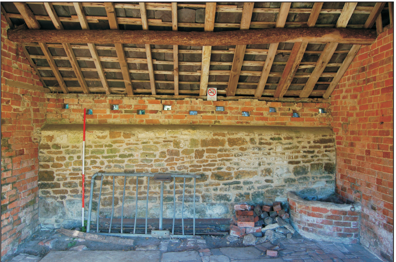
The east internal wall of the hovel, looking east Plate 2
