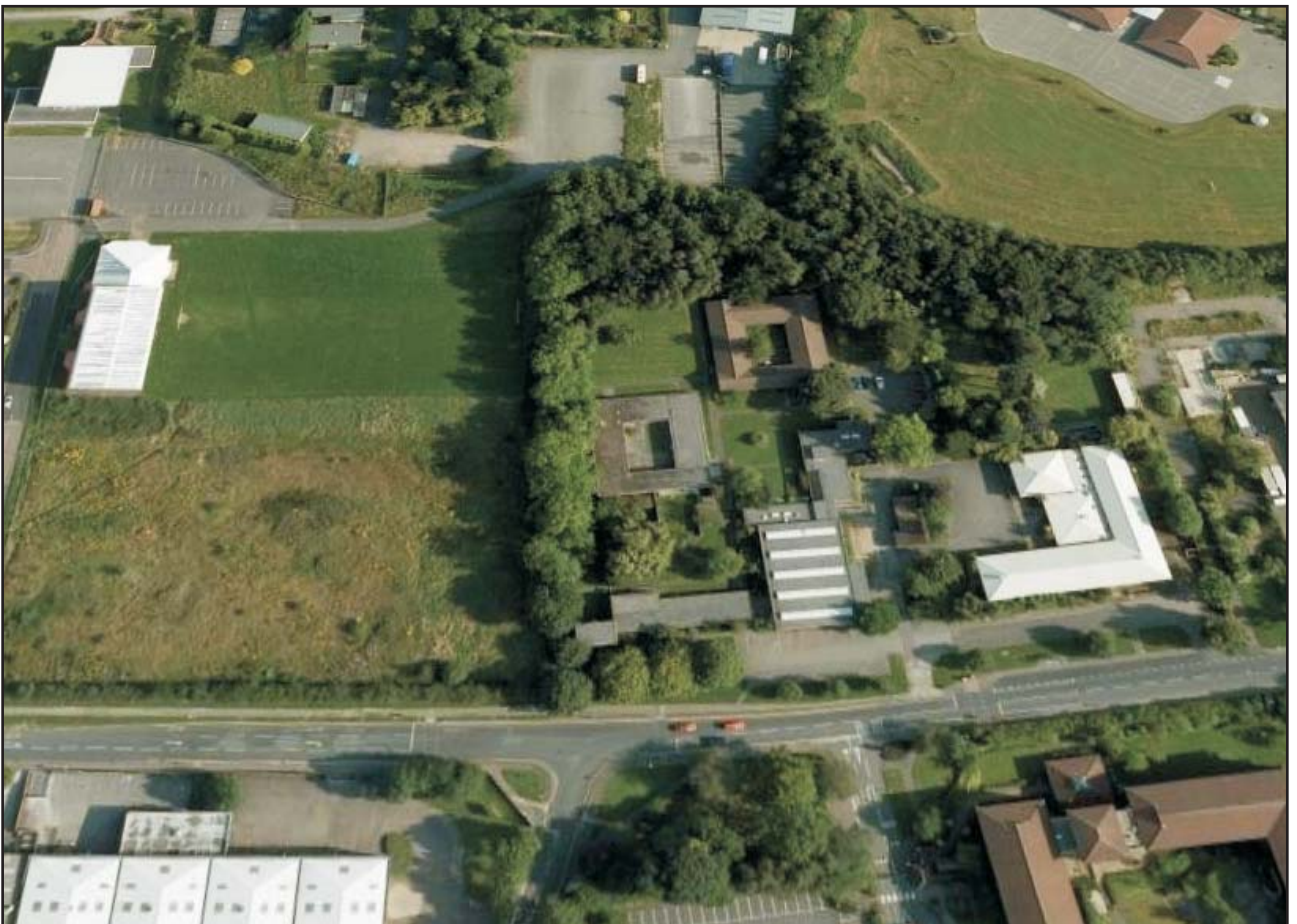
Aerial photograph of site prior to demolition and clearance 2005 Fig 10
