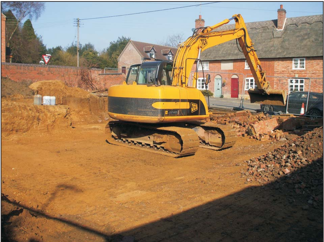
View of the development area, post excavation, looking north Fig 9
