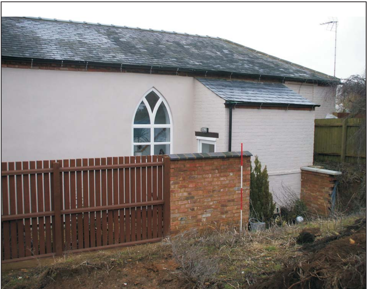
The western elevation before development, looking south-east Fig 5
