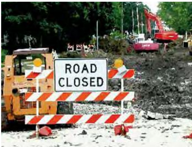
Traditional open cut pipe replacement project
