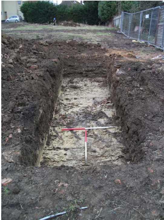
Trench 2, looking south-west
