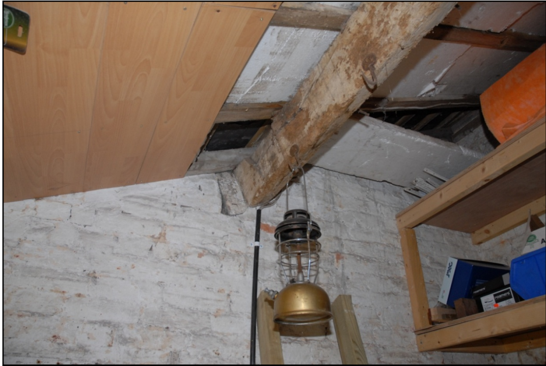
Purlin in Room 3, showing timber re-use and iron hooks Fig 11
