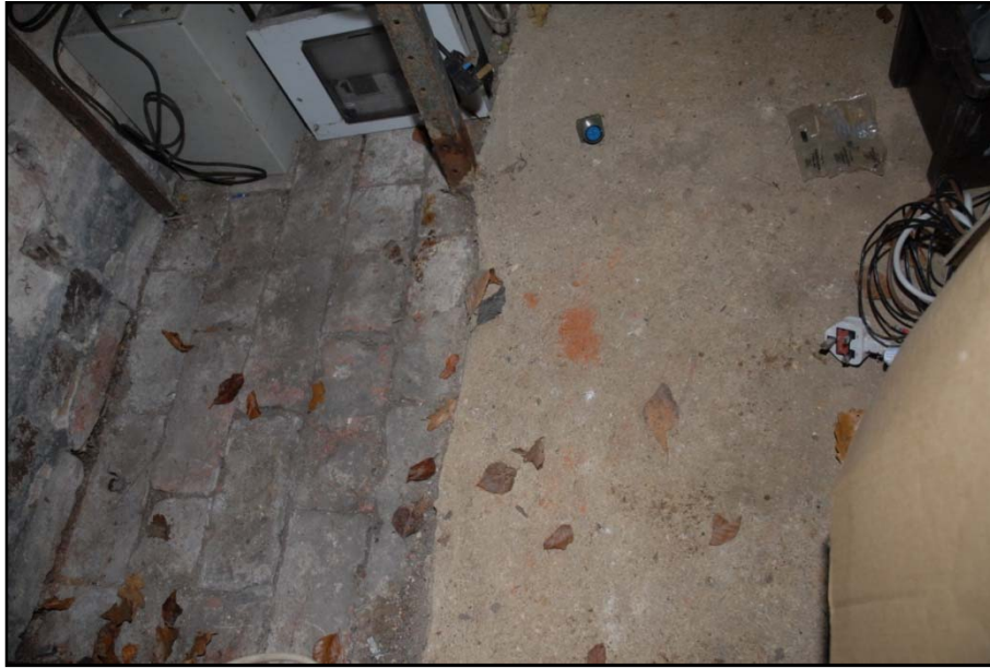
The original brick floor, overlain by concrete, Room 1 Fig 8
