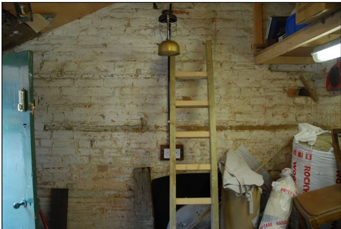
The timber courses in the brickwork of Room 3, looking south Fig 12
