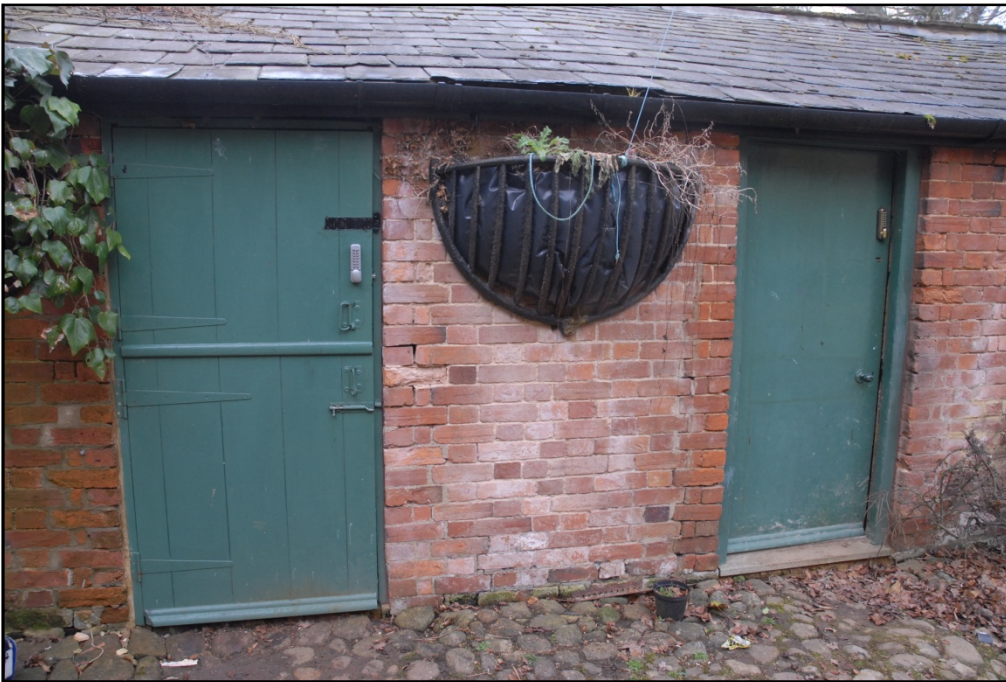
The doorways to Rooms 2 and 3, and later iron manger Fig 18
