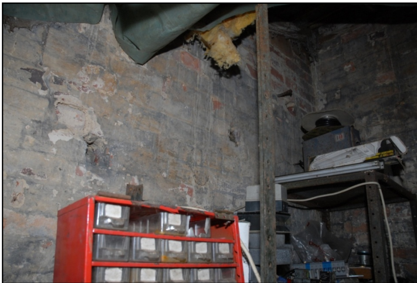
Beam slots in the southern wall of Room 1 Fig 7
