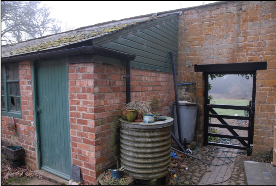
North elevation showing weather boarding (Fig 4)
