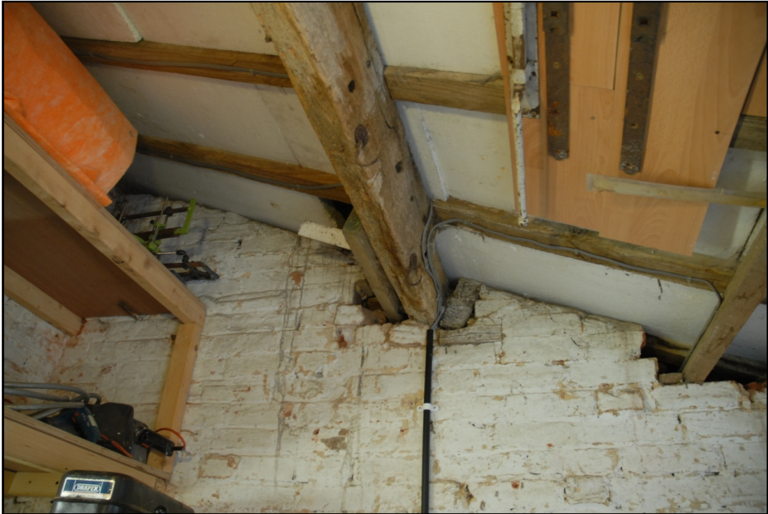
The alteration of brickwork to accommodate the purlin, Room 3 Fig 13
