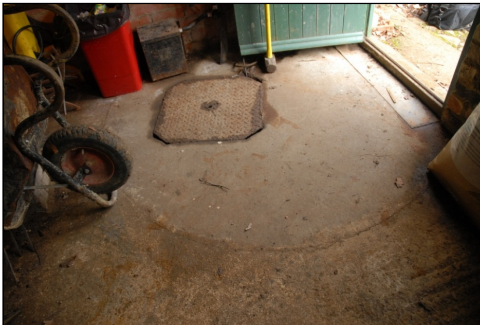
The drain access and concrete surround in Room 4, looking north Fig 16
