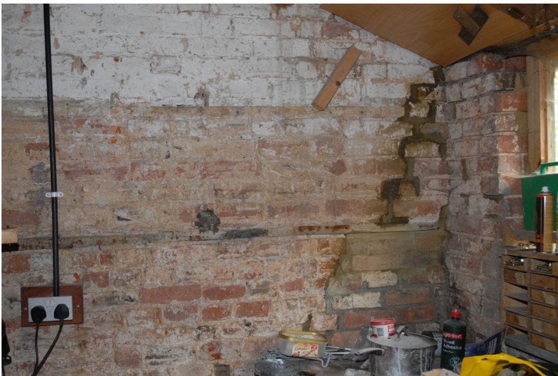
Area of modern brickwork in the north eastern corner of Room 3 Fig 14
