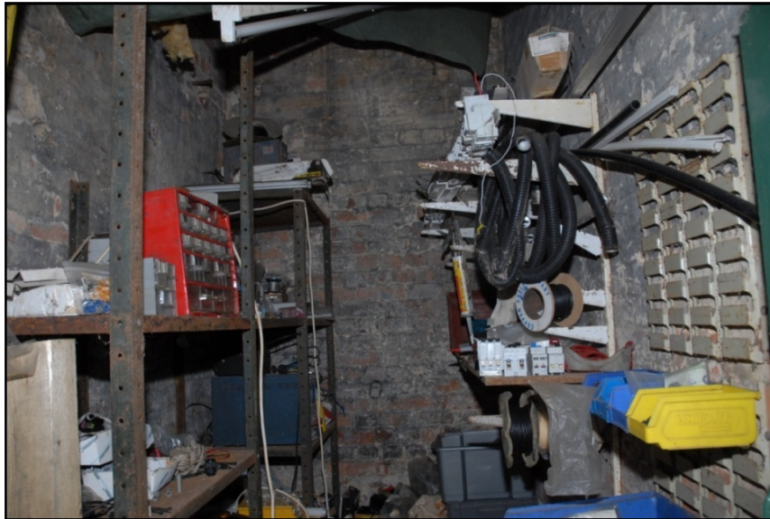
Room 1, looking west Fig 6
