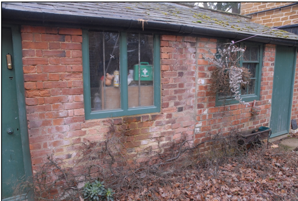
Demolition scar and vertical joint between Rooms 3 and 4 Fig 19
