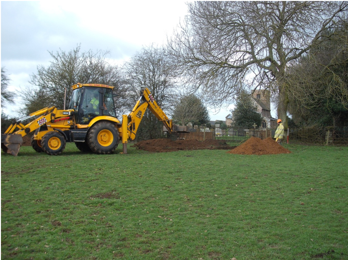
General view of the excavation of trench 1, looking west Fig 4
