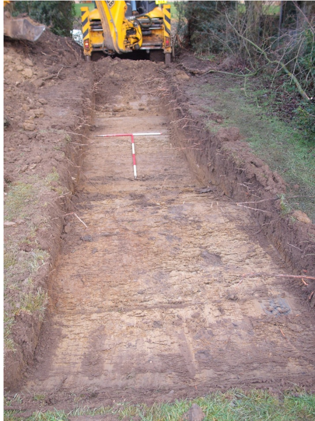
Trench 2 after excavation, looking north Fig 5
