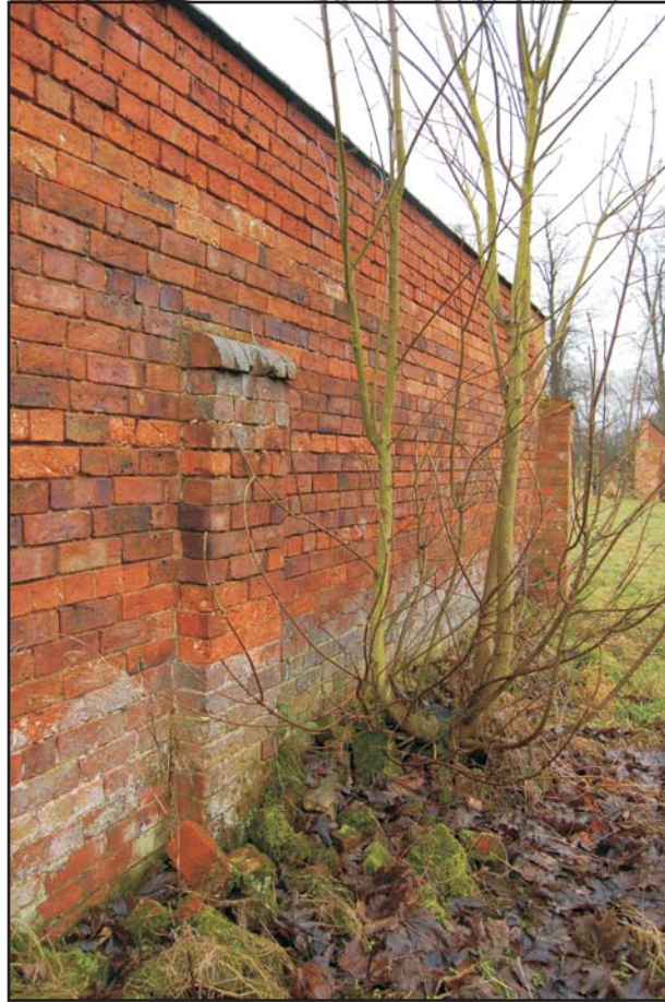
Wall buttress with capping of bullnose bricks laid on edge Plate 5
