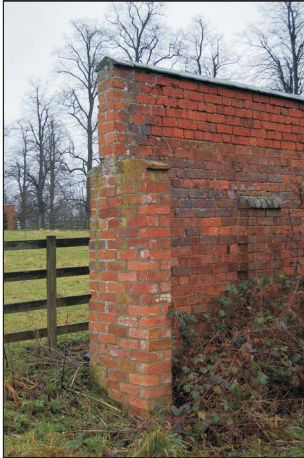
Re-built ends of the east wall with terminal buttresses, looking south-east Plate 7
