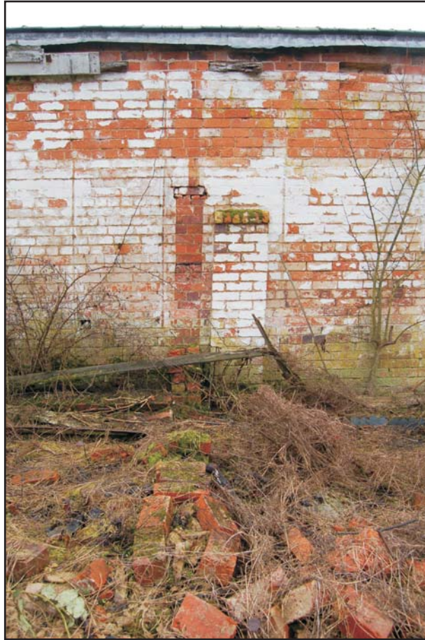
Scar of middle internal dividing wall within the glasshouse, looking east Plate 17
