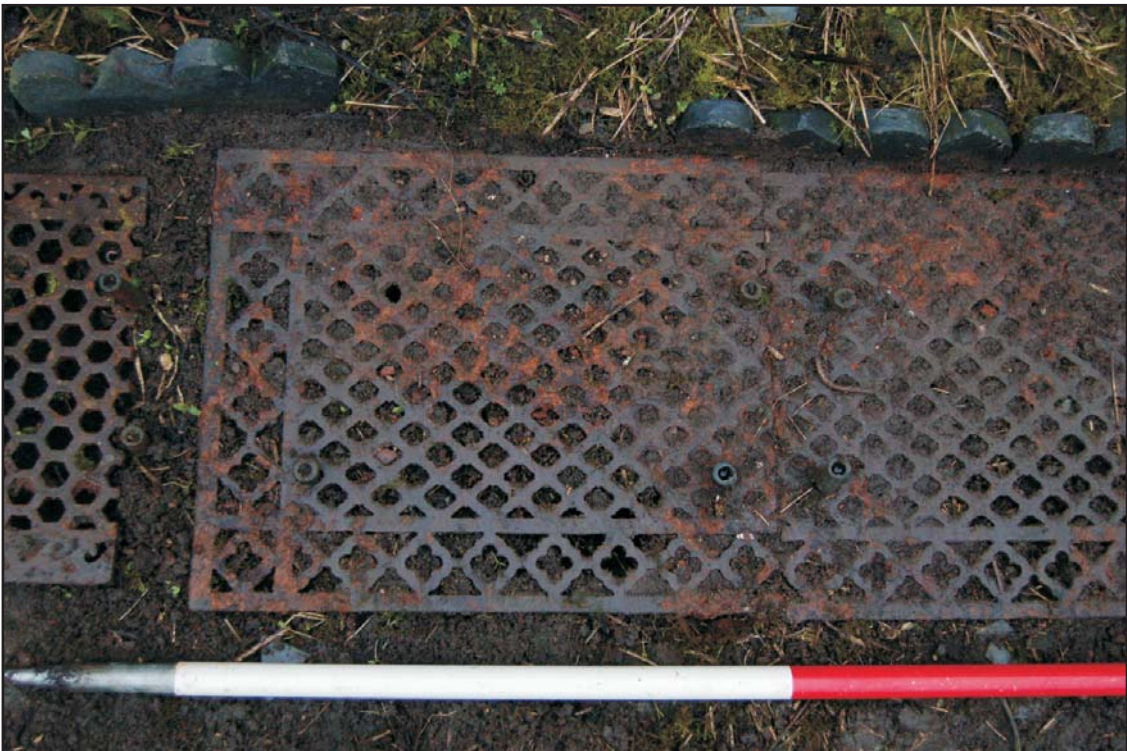
Heating grille, scale 0.5m Plate 20
