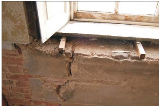
Window sill in State Bedroom Fig 14
