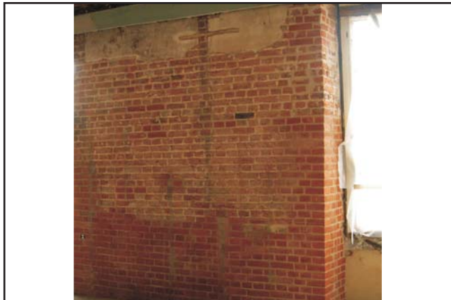
Mark left by removal of former panelling style Fig 7
