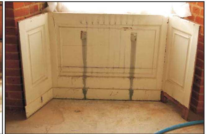
Panelling removed from beneath Library windows Fig 6
