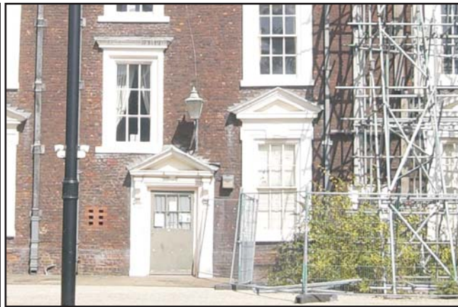
Stair-landing window in west front of house Fig 11
