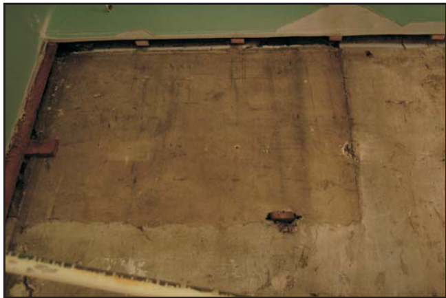
Blocked embrasure in Library south wall Fig 10
