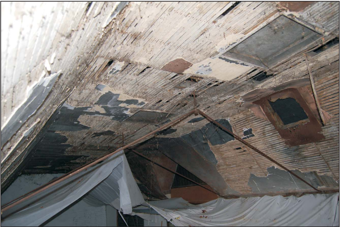
The ceiling of the eastern range, looking south Plate 13
