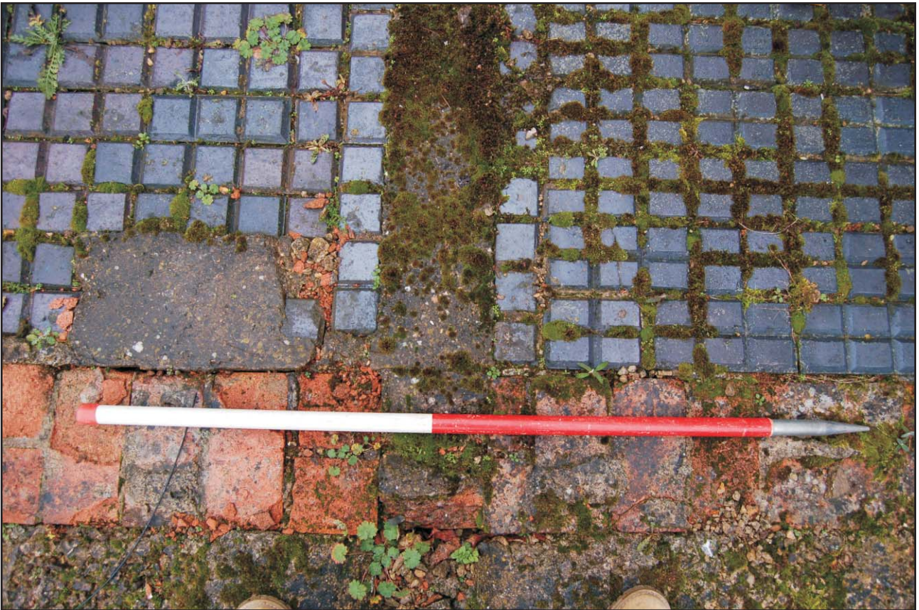
Staffordshire blue pavers; three section bricks to the left, six section bricks to the right Plate 8
