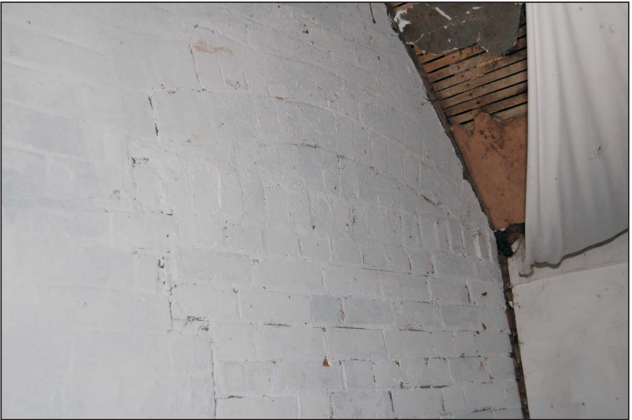
Segmental arch over blocked doorway in the south gable wall Plate 17
