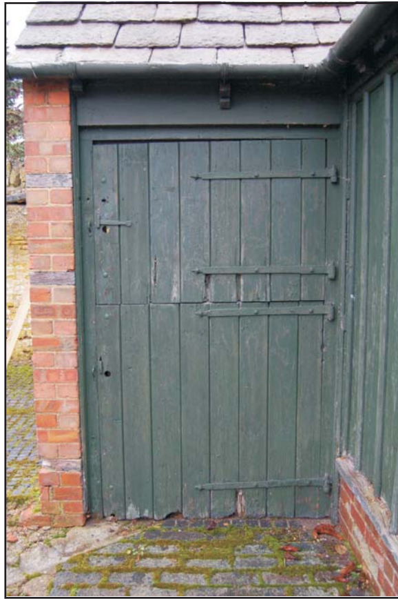
Stable door exterior, looking north Plate 4
