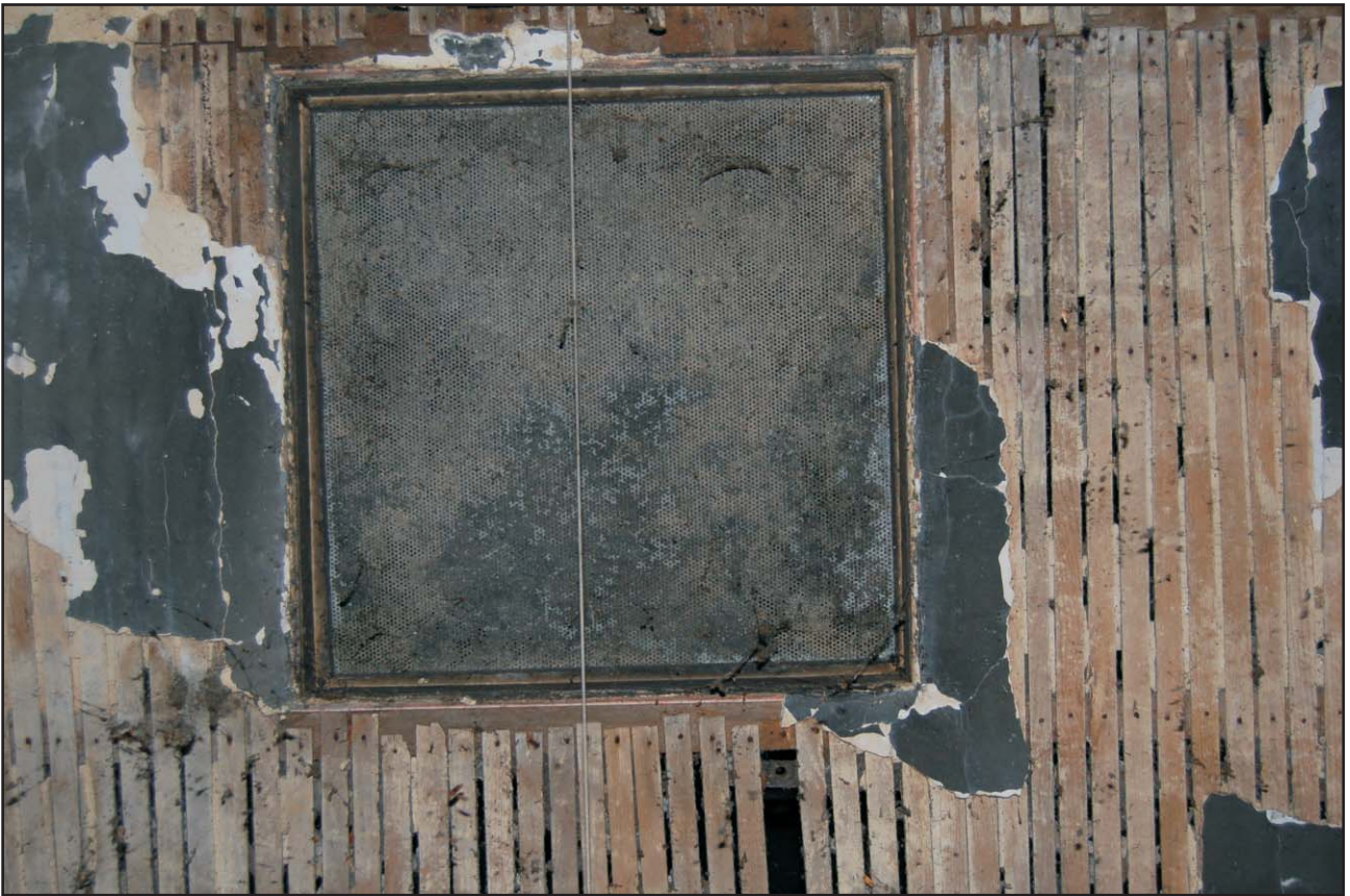
Mesh filled ceiling vent Plate 15
