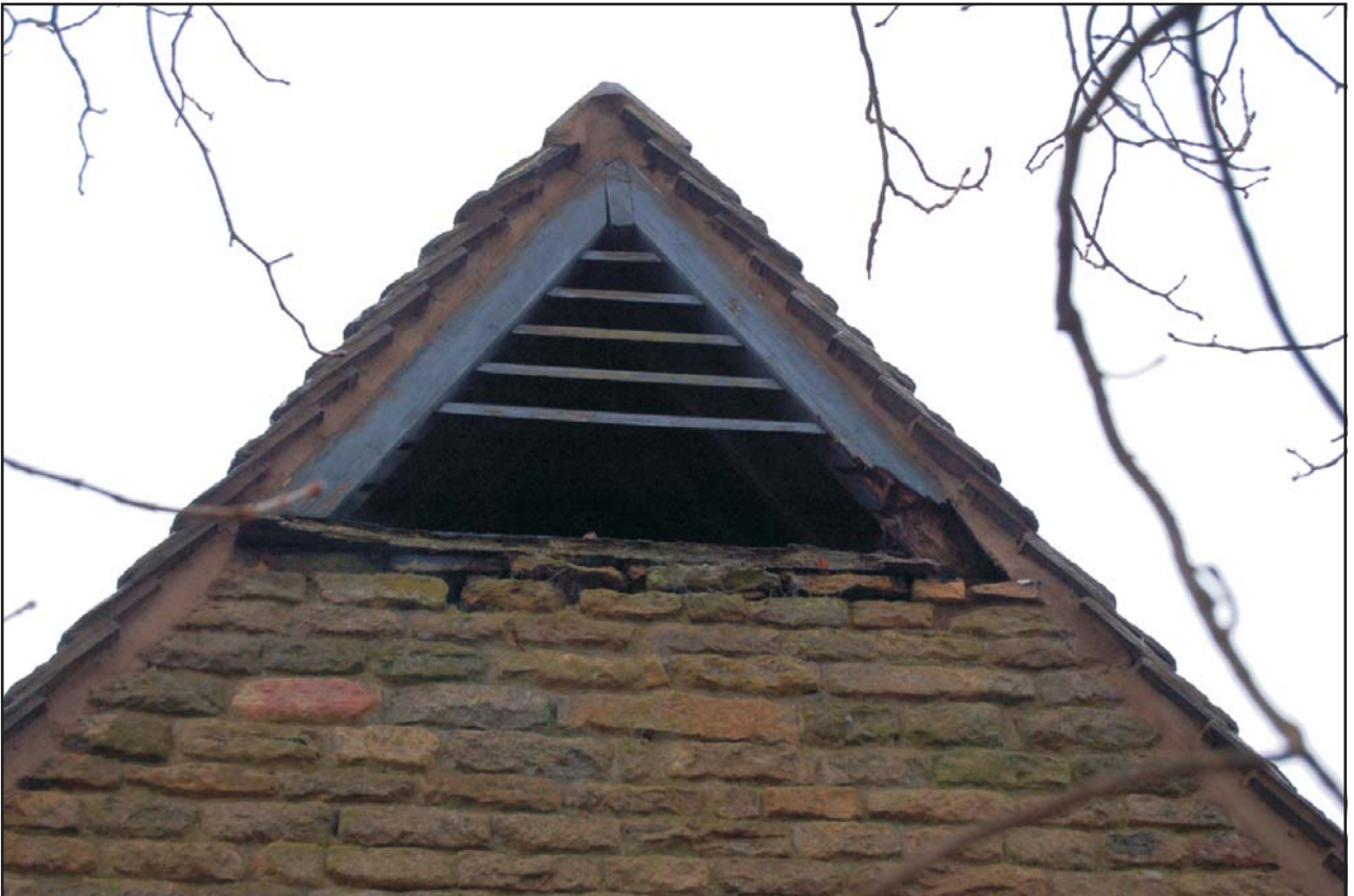
Louvred gablet in south gable wall Plate 5
