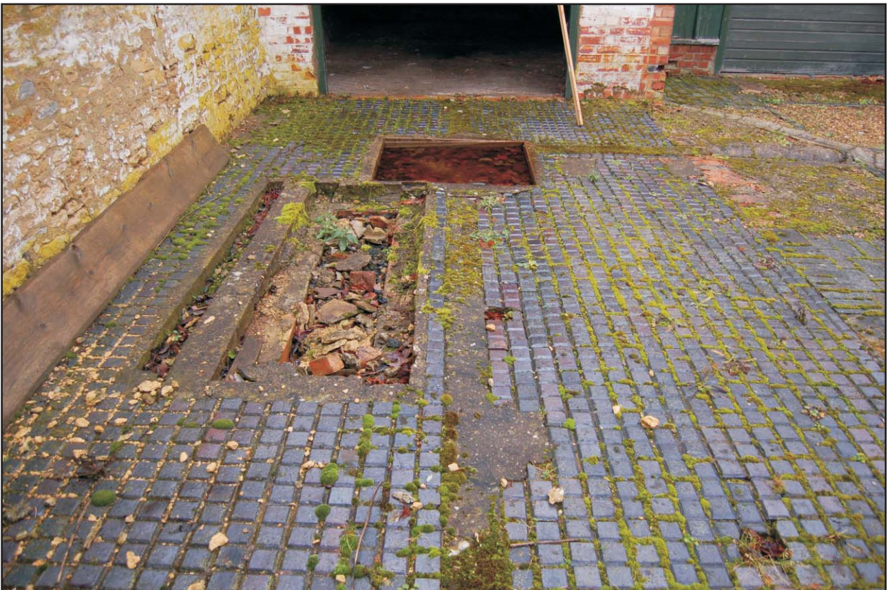
Brick and cement sumps in floor of demolished range, looking east Plate 7
