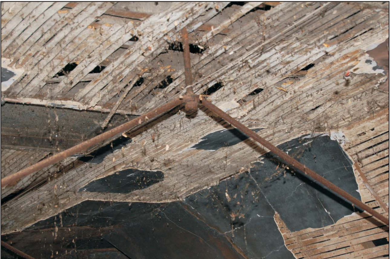
Detail of iron tie rods Plate 14
