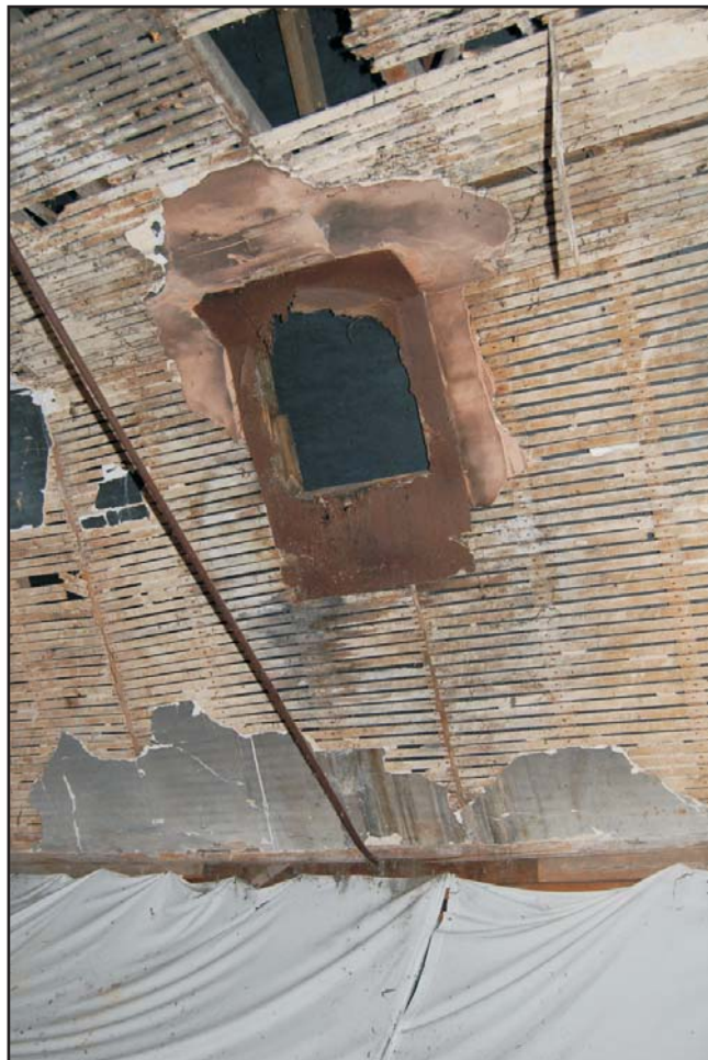
Metal sheet fixed over plaster around former flue Plate 16
