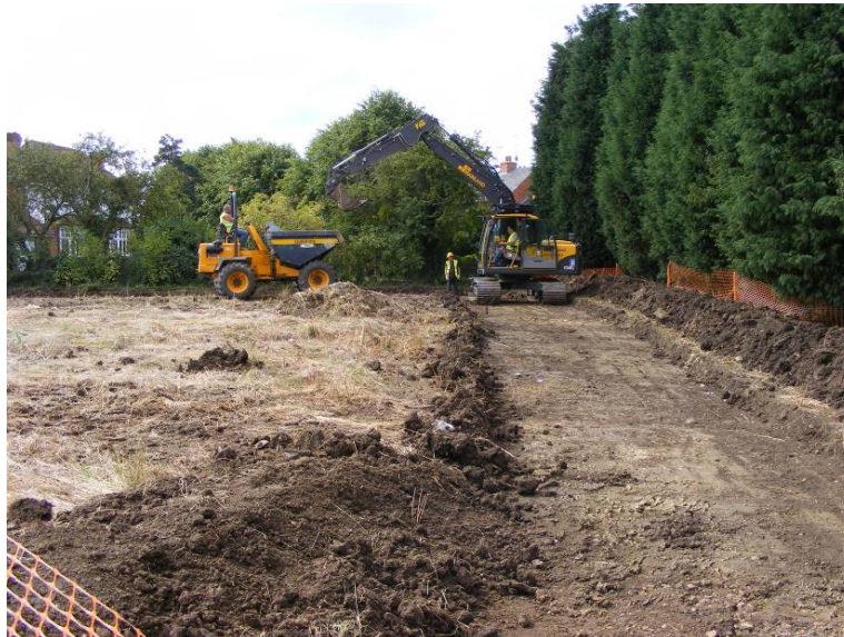
Area 1 under excavation, looking south-west Fig 4
