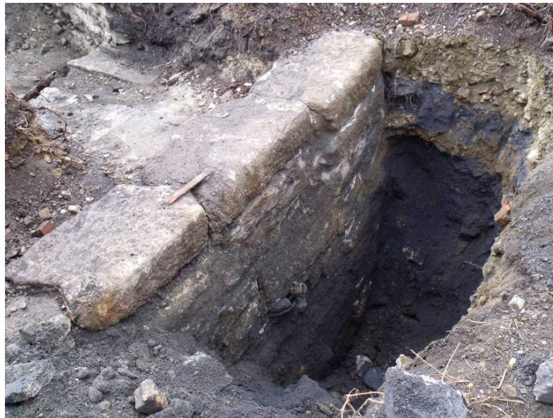
Trench 20, showing vertical joint between the two stones at the top of the picture and the chevron style of joint Fig 48
