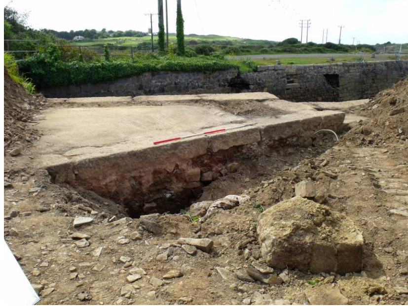
Trench 18, west wall of Carnsew Dock, looking north-east, the step visible on the right of the wall is that also seen in Figure 13 (Scale 2m) Fig 44
