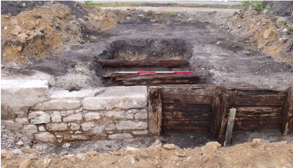
Trench 8, the join between the stone quay and timber slipway revetment (Scale 2m) Fig 21
