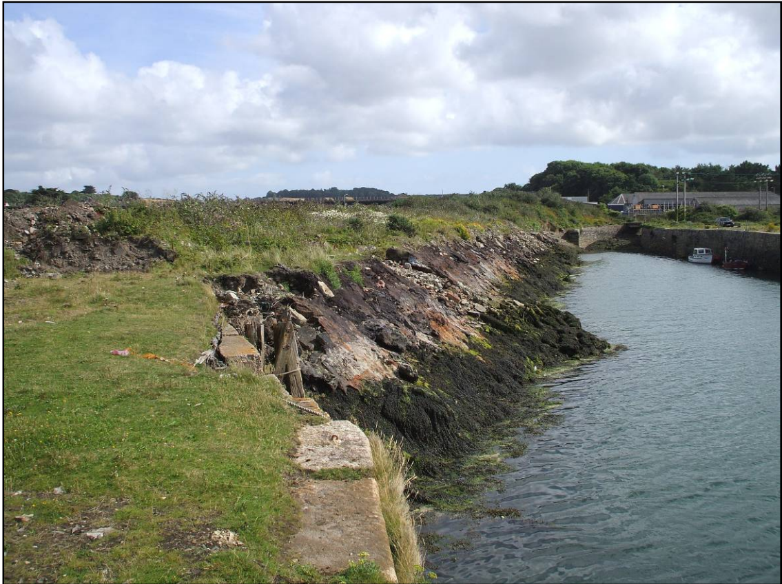
A view of the material in-filling South Quay and Carnsew Channel, looking south Fig 3
