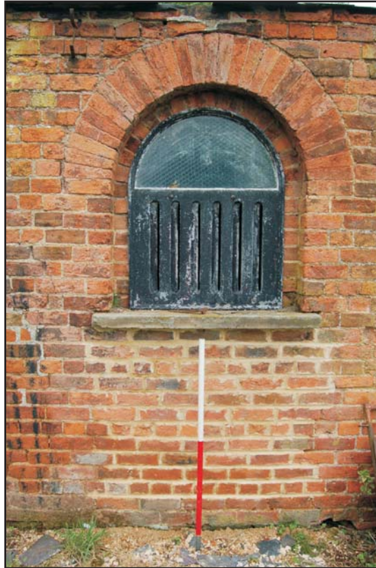
The south range arched window with cast iron frame and ventilation slats, looking east
