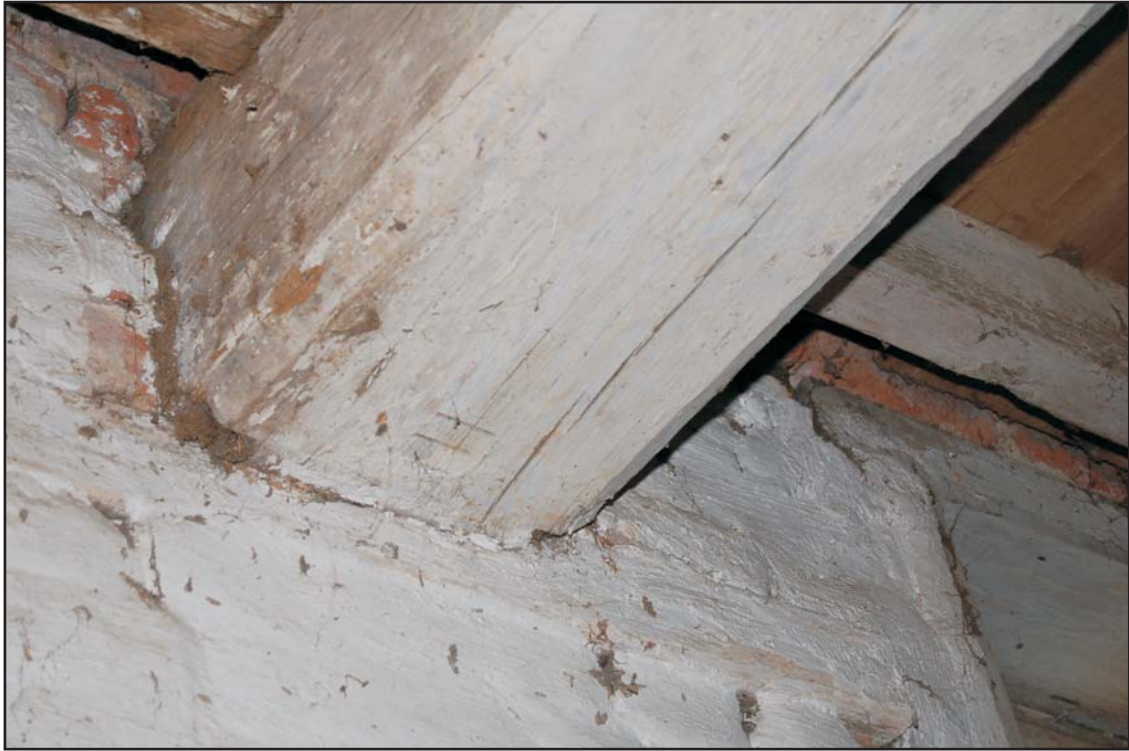
East end of the south beam in Room 1 with carpenters marks IIII Plate 3
