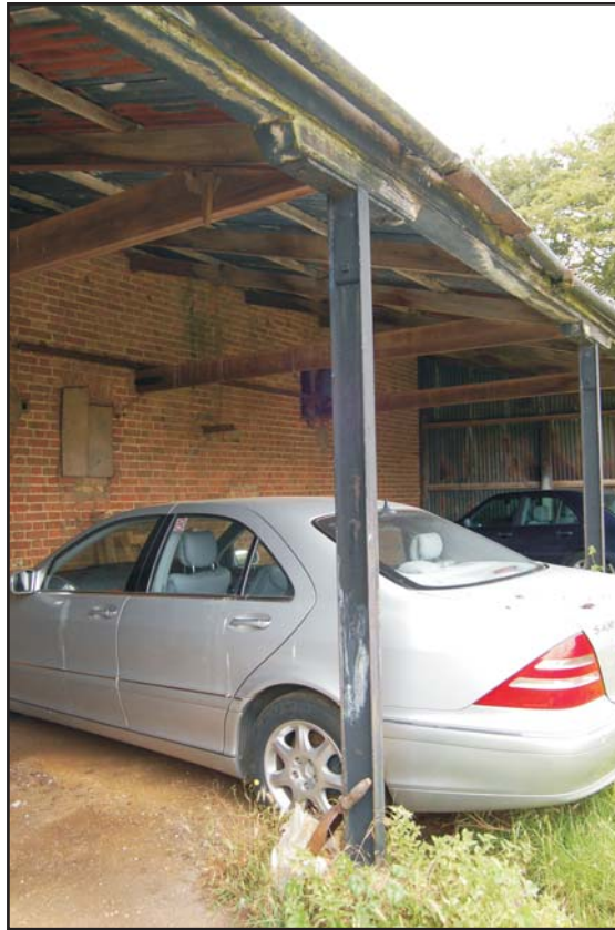
Cart hovel on the east side of the two storey barn showing H-section post, looking north-west Plate 21
