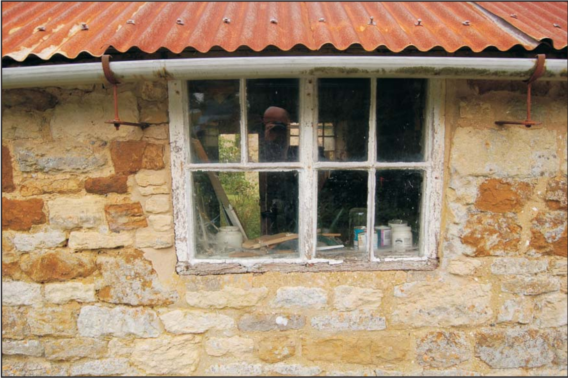
The window in the south wall, looking north Plate 5
