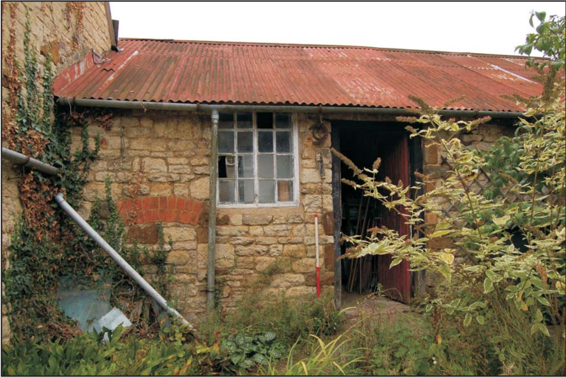
The north elevation showing current and blocked openings, looking south Plate 1
