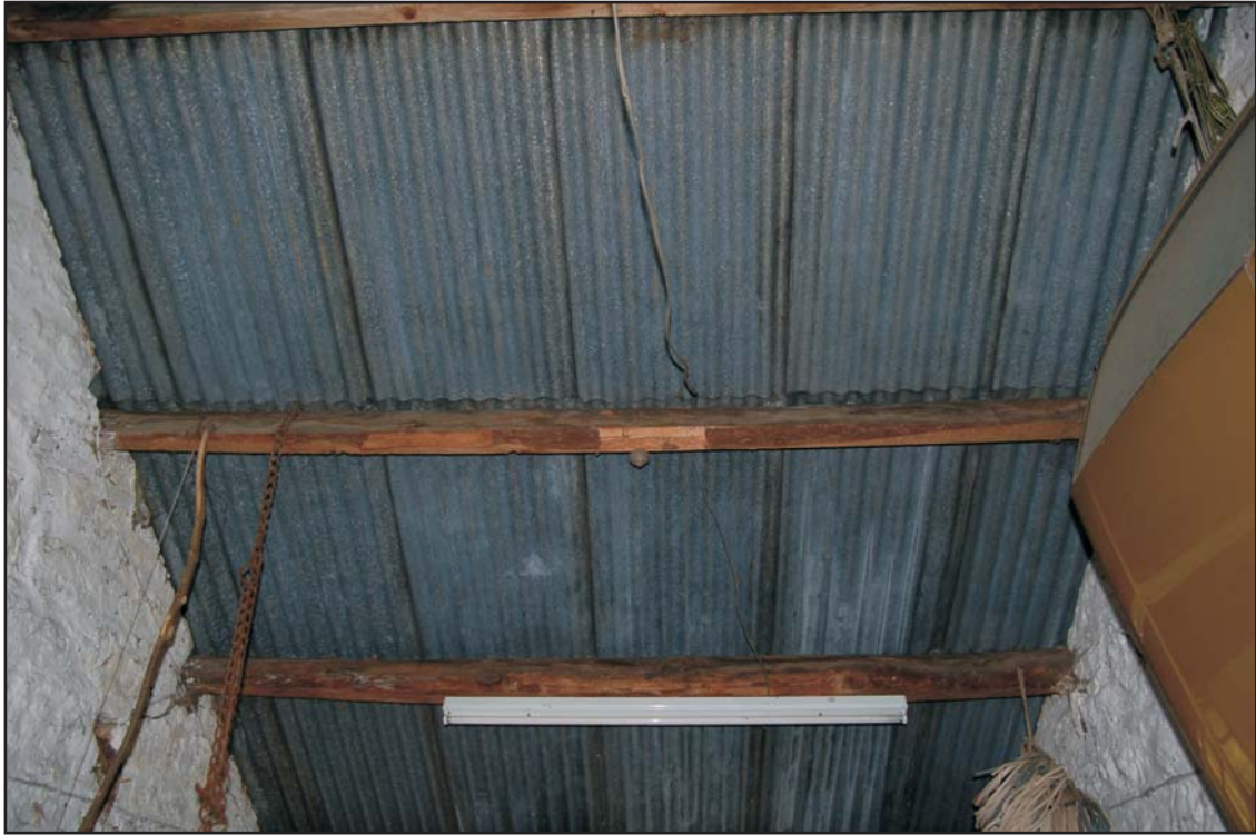
The roof structure in Room 1, looking north Plate 7
