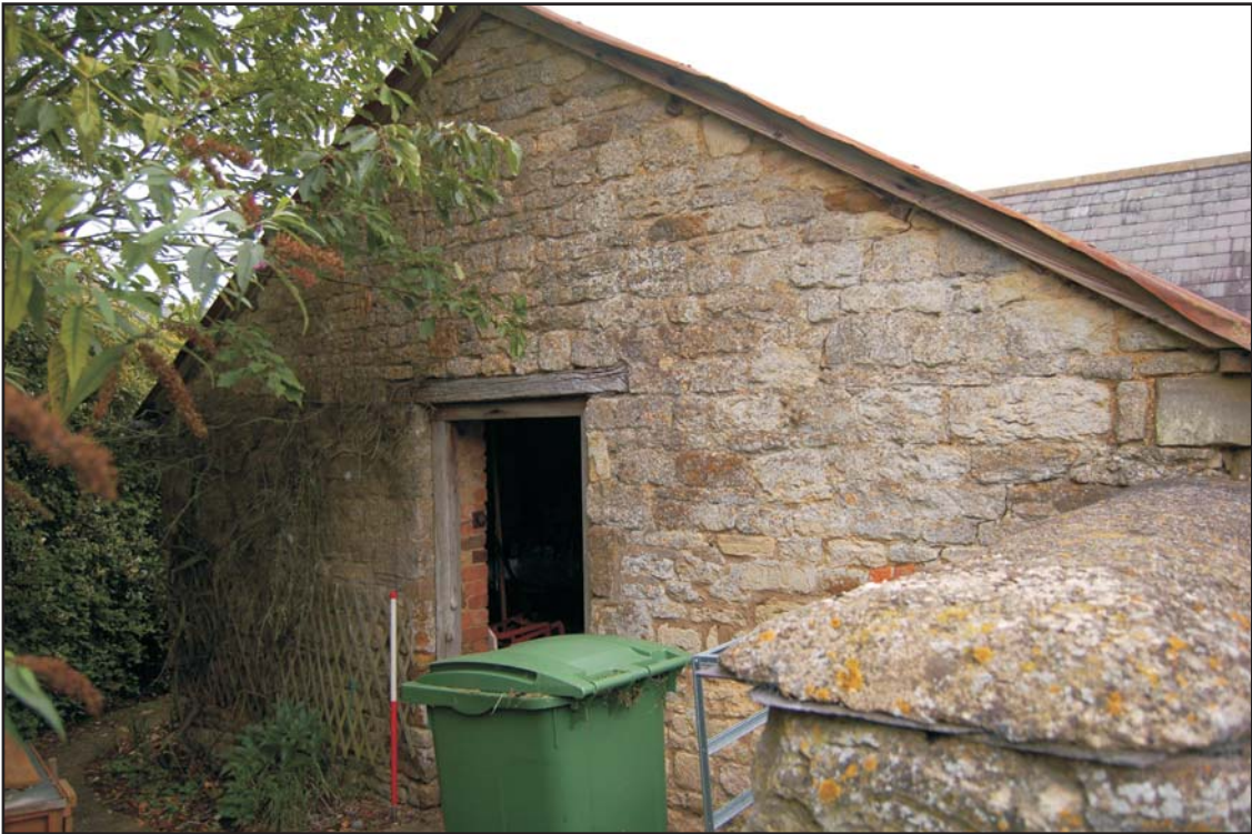
The west elevation, looking north-east Plate 2
